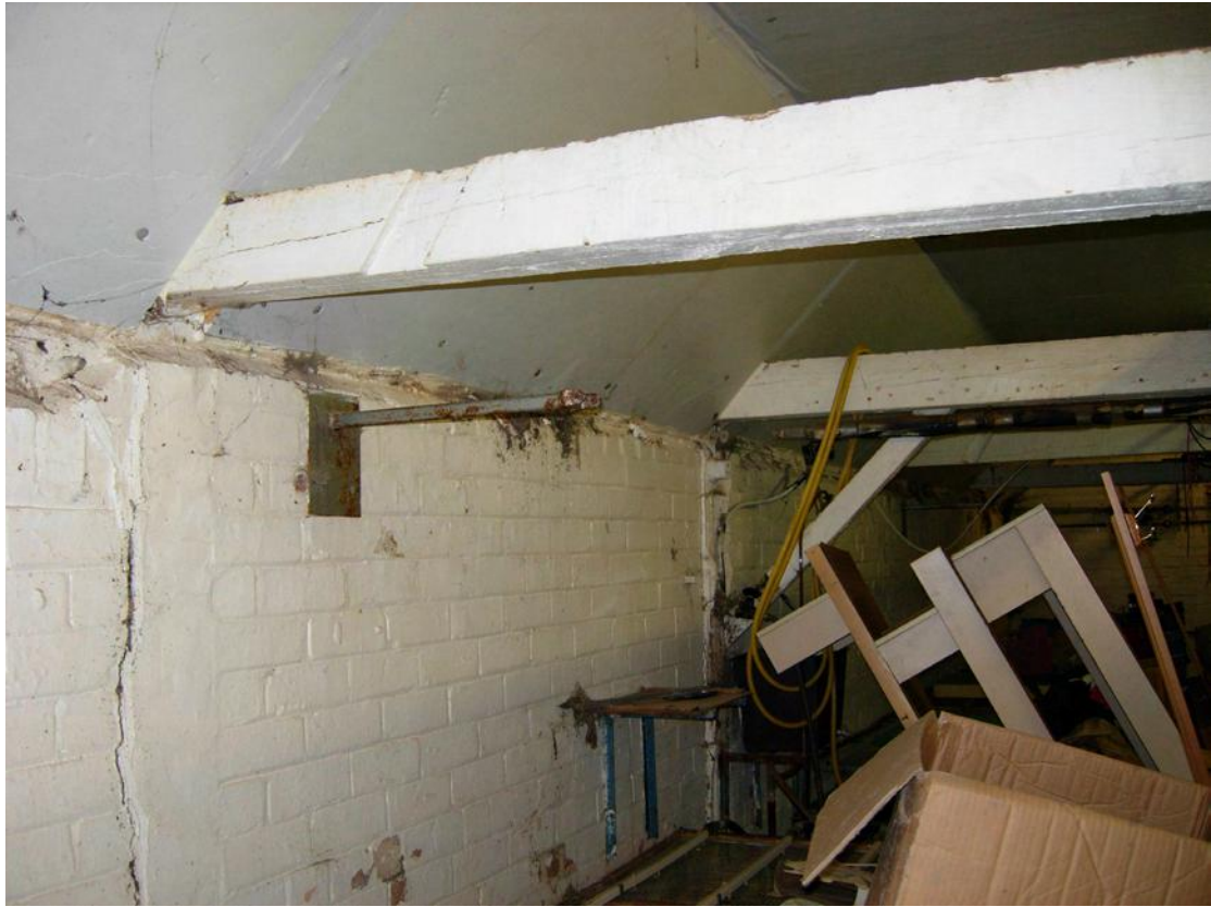
Plate 29 Beam, strut and evidence for former struts in building D, looking north
