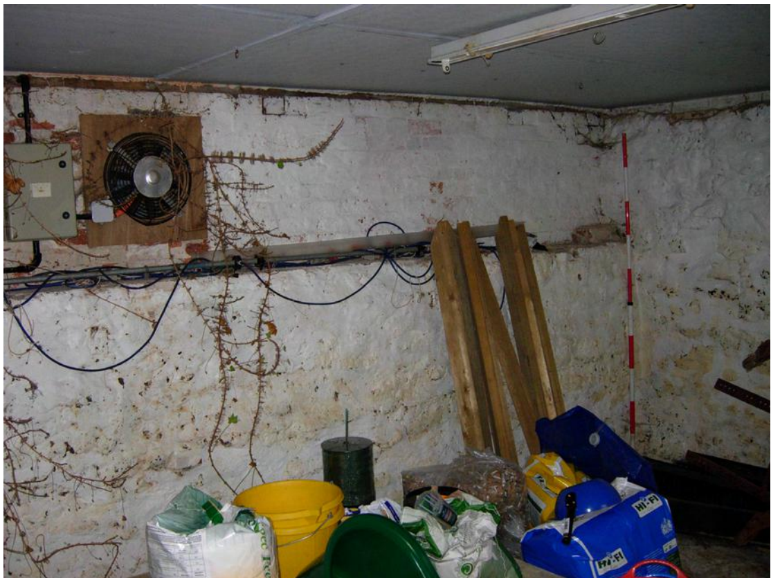
Plate 26 Brick and rubble-stone north wall of room 1, building C
