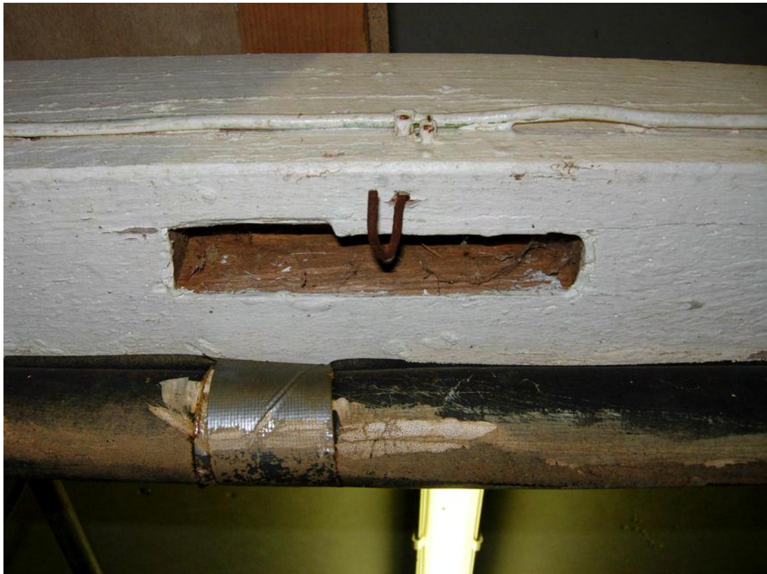
Plate 31 Mortice in the underside of a beam, building D
