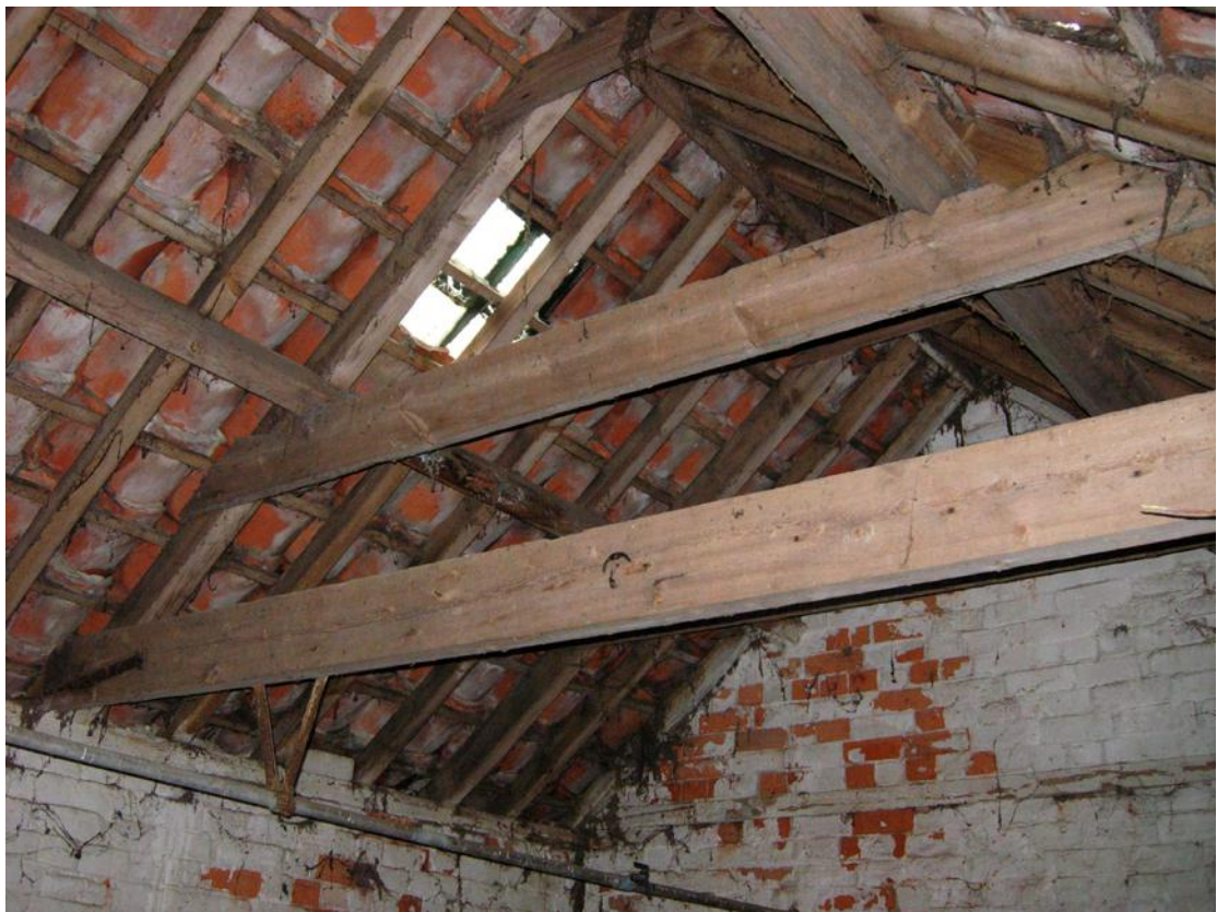
Plate 24 Collar detailing, room 3 building B, looking south-west
