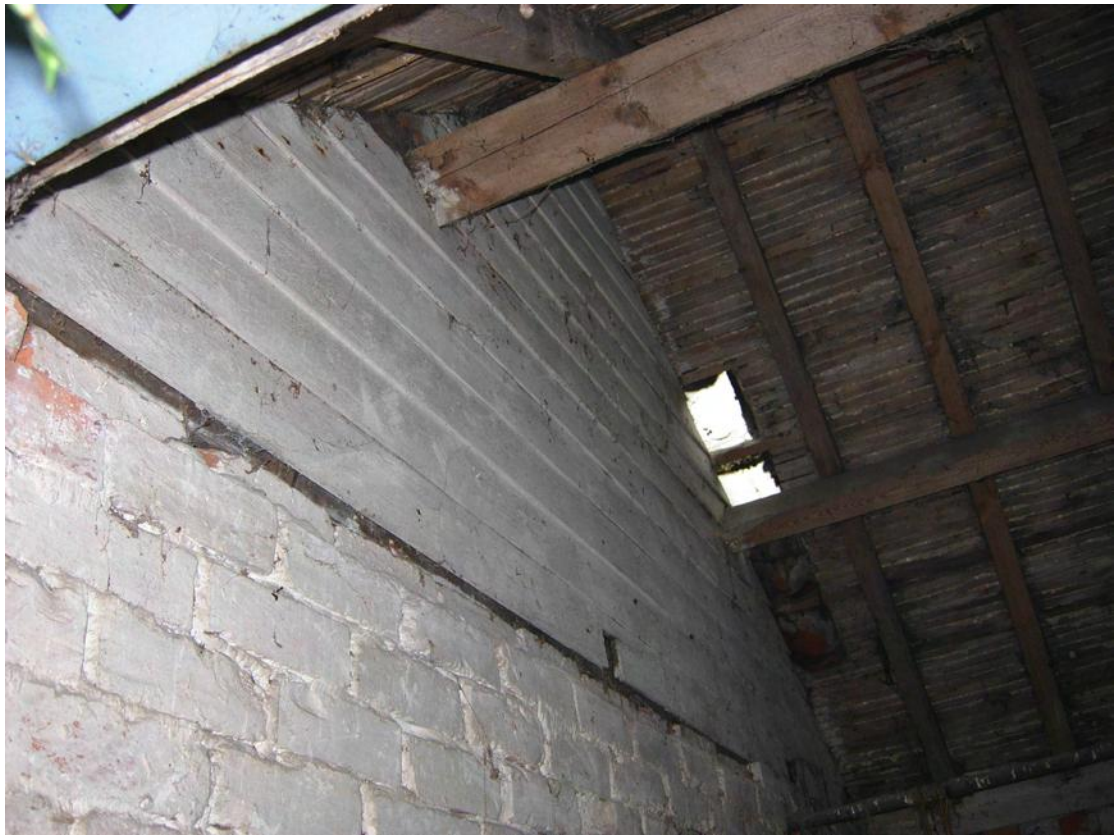
Plate 23 Clapboard upper partition above east wall of room 2, building B
