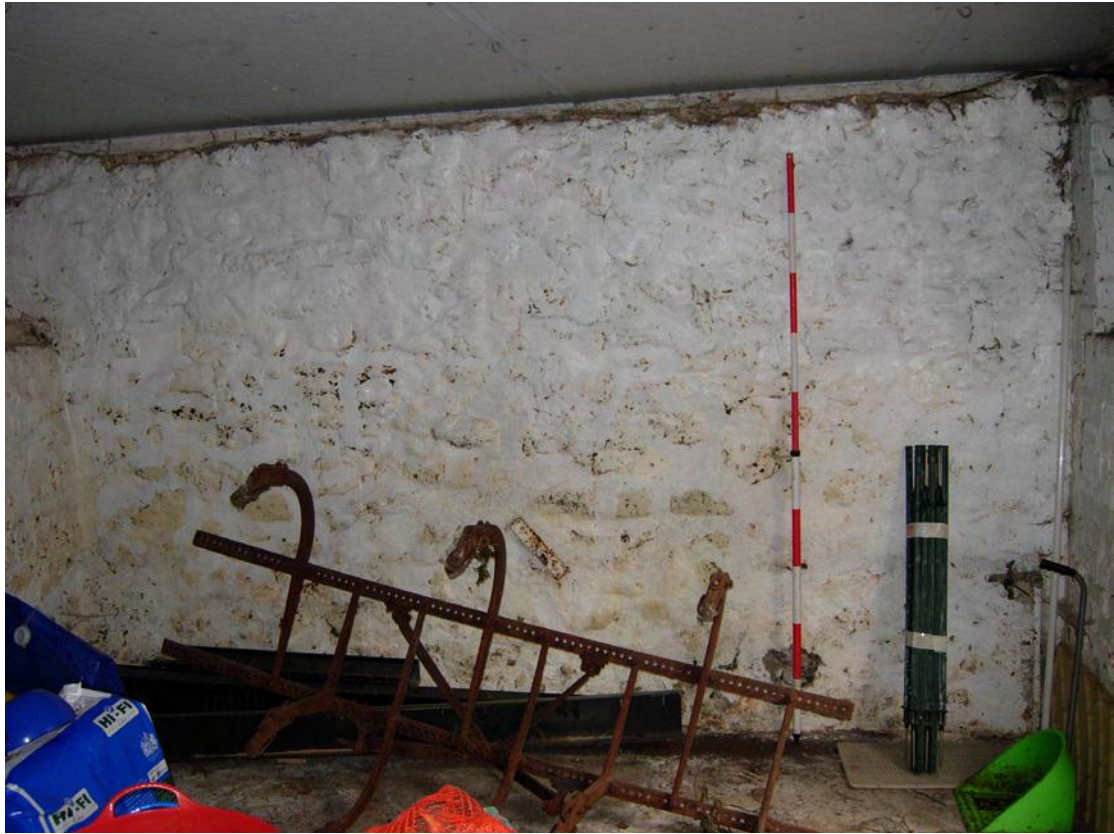
Plate 25 Rubble-stone east wall of room 1, building C
