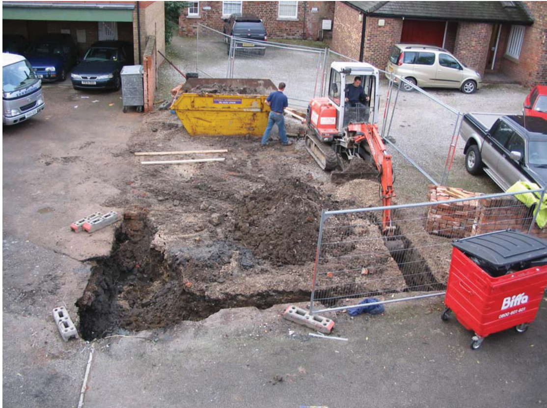
Plate 3 The foundation trenches under excavation with the modern wall foundation visible in the western trench
