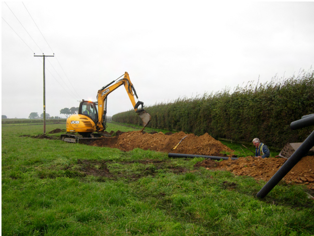
Plate 12 Spur 2 of the cable trench viewed from the east
