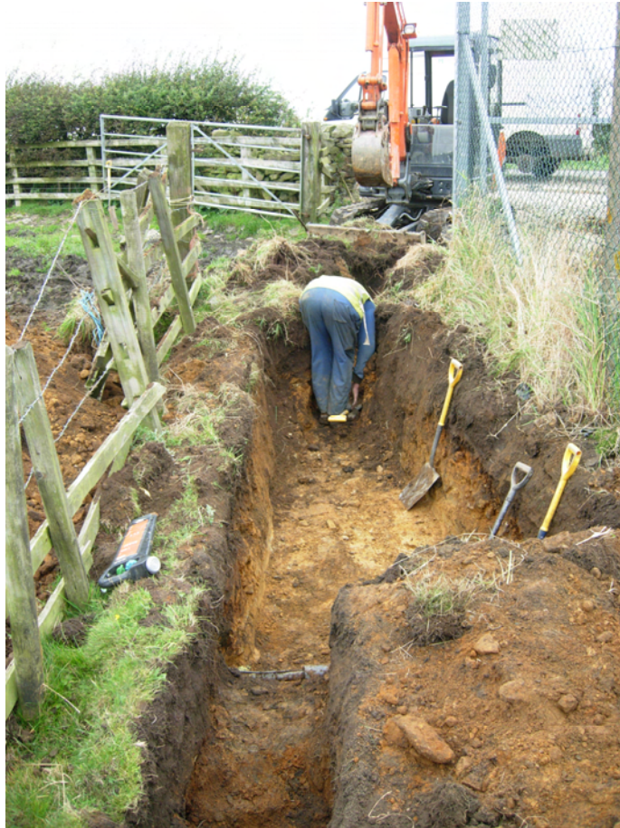
Plate 11 Spur 1 of the cable trench viewed from the south
