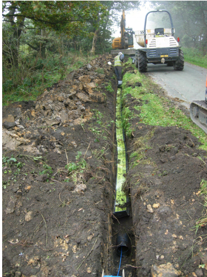
Plate 3 The eastern portion of the cable trench being excavated looking west
