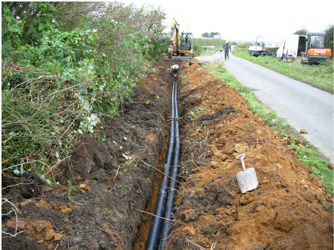
Plate 8 The western portion of the cable trench being excavated looking west
