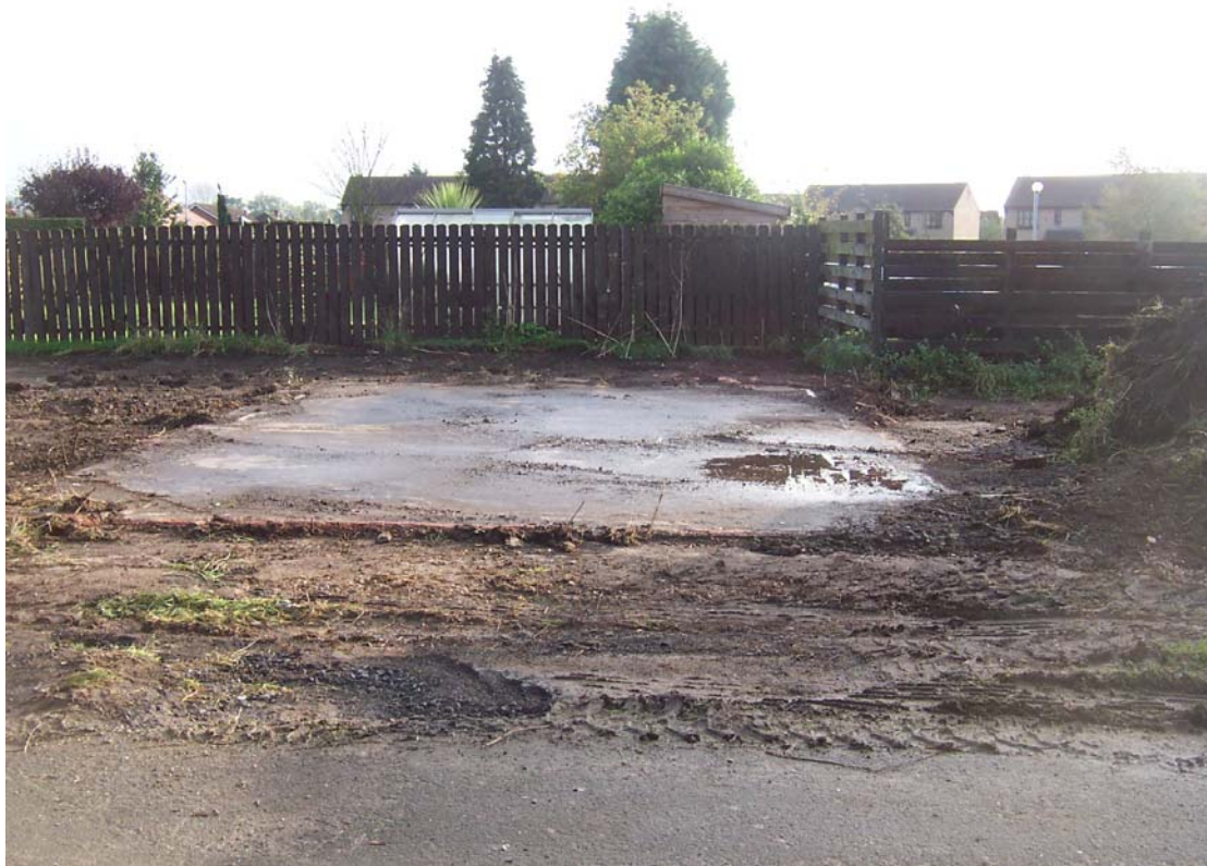
Plate 3 Remains of shallow 20 th century concrete and brick structure bases in the north-eastern area of the development, looking east.
