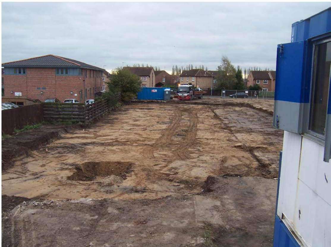
Plate 6 The building raft foundations nearing completion, viewed from the north.
