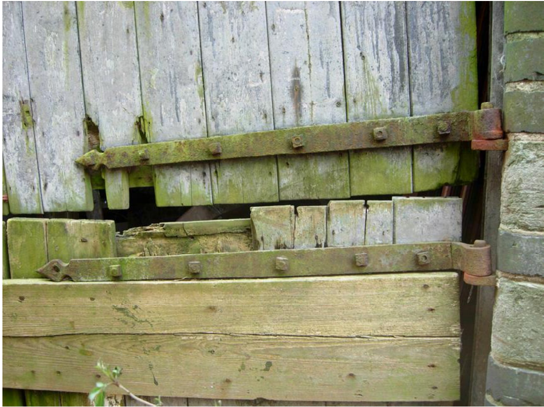
Plate 25 Detail of the iron straps on the heck doors of one of the loose boxes (room 5)
