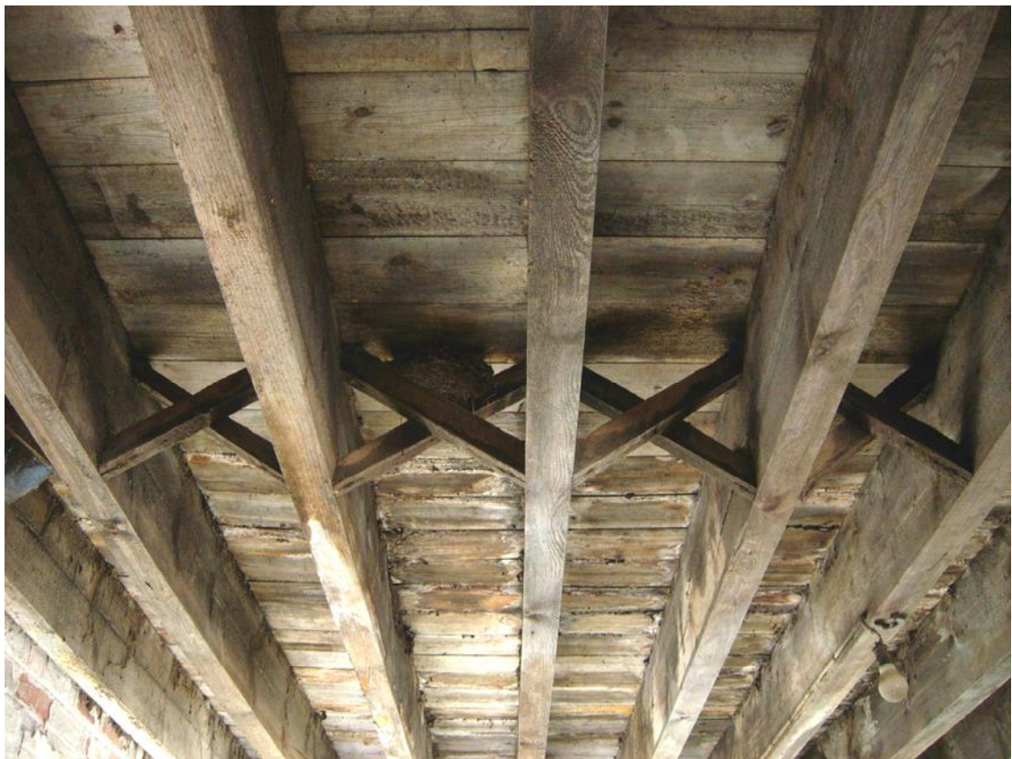
Plate 24 Herringbone strutting (cross-nogging) in the ceiling of room 4
