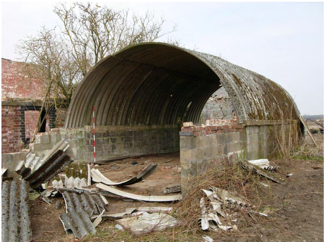
Plate 8 The corrugated asbestos shelter to the east of the other farm buildings (2m scale)
