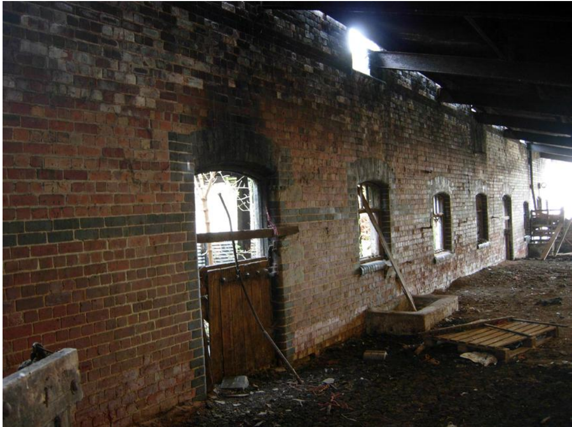
Plate 17 The south elevation of the north range
