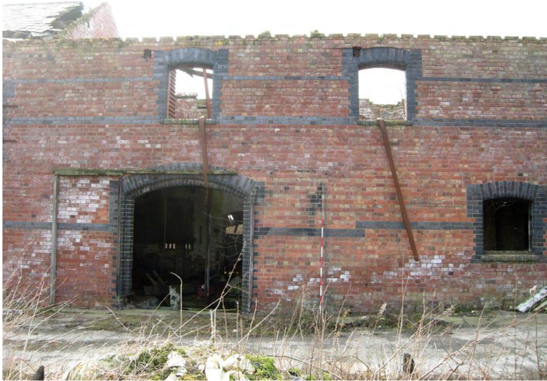
Plate 5 The eastern part of the north range (2m scale)
