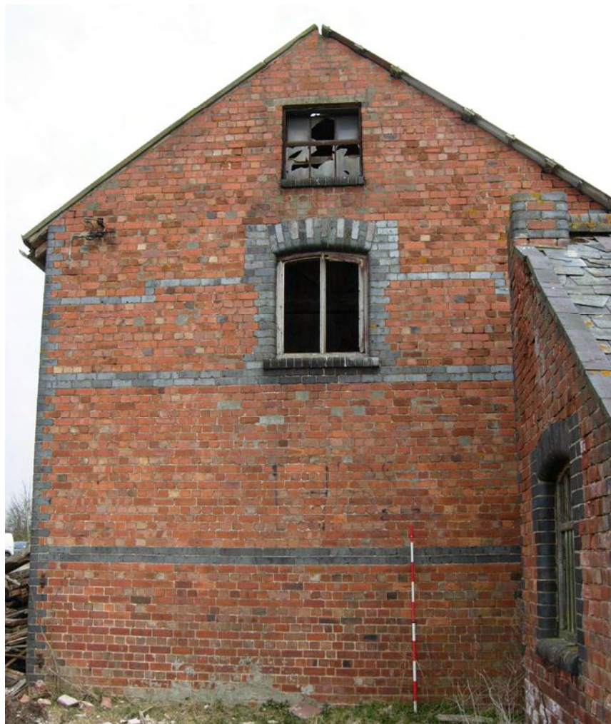
Plate 12 The south elevation of the west range (2m scale)
