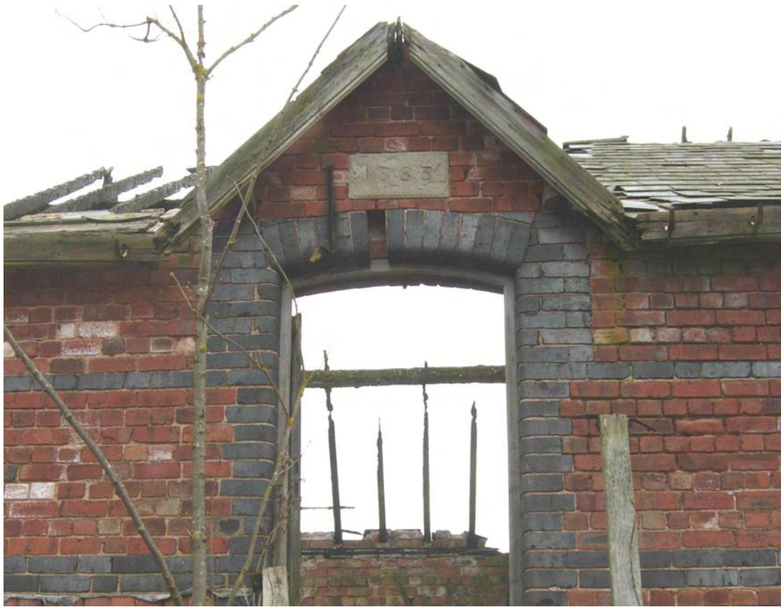
Plate 15 Date stone (1883) over the central portion of the west range
