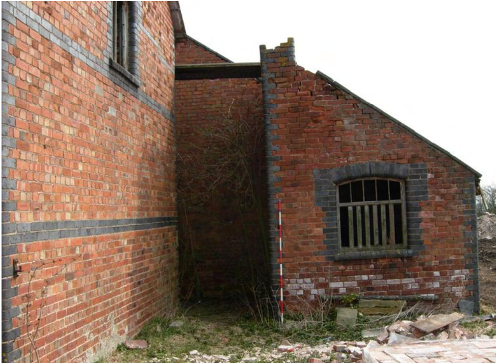
Plate 11 The west elevation of the south range (2m scale)
