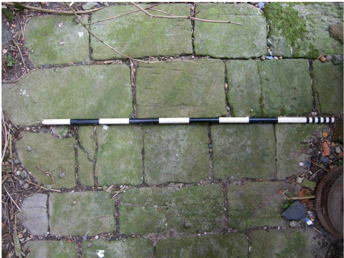
Plate 26 Detail of the stone setts in the passageway between the calf house (?) and the loose boxes (1m scale)
