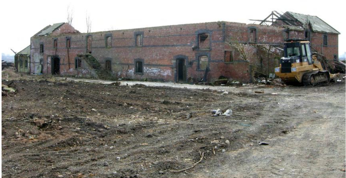
Plate 2 General view of the farm buildings from the north-west
