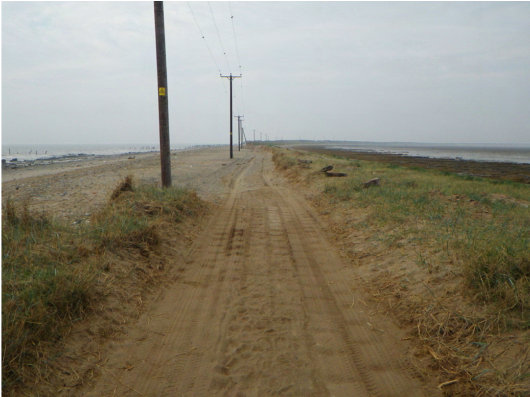
Plate 1 The site of the development, showing the collapsed and washed-out road; the proposed road is to the west (right). Viewed from the north.
