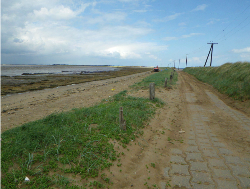
Plate 5 Showing the remainder of the water service pipe trench from the southerly extent of the works, looking north.
