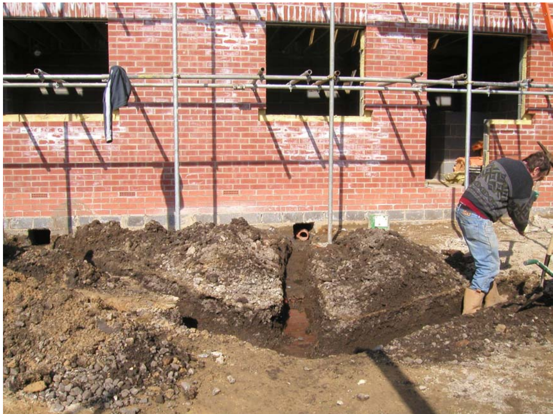
Plate 4 The hand excavation of the shallow service trenches, looking north-west.
