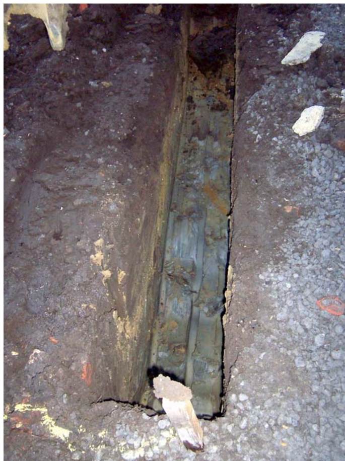
Plate 2 The excavation of the foundation trenches in progress, viewed from northwest
