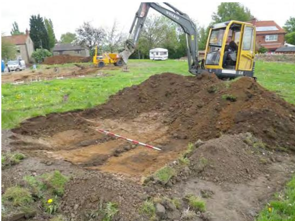
Plate 4 Topsoil strip for the wildlife pond viewed from the south
