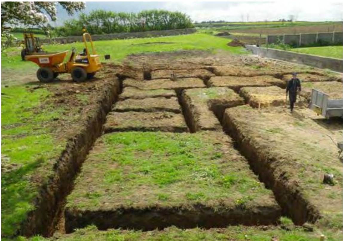
Plate 2 The completed foundation trenches viewed from the north
