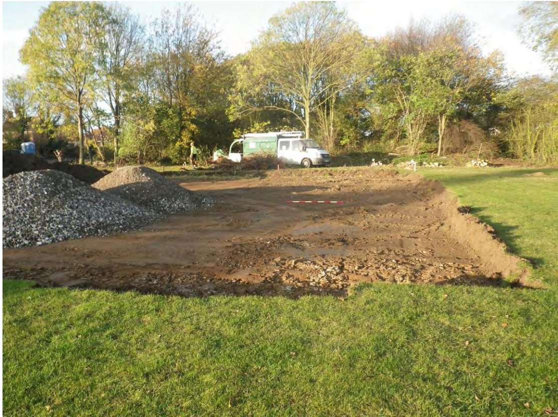
Plate 3 Stripping the northern half of the extension, looking north, 2m scale
