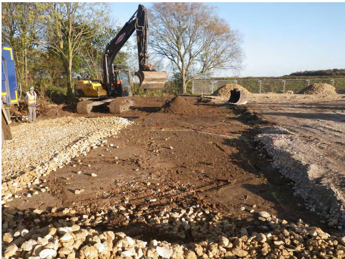
Plate 4 The location of the emergency access road (far left), looking east
