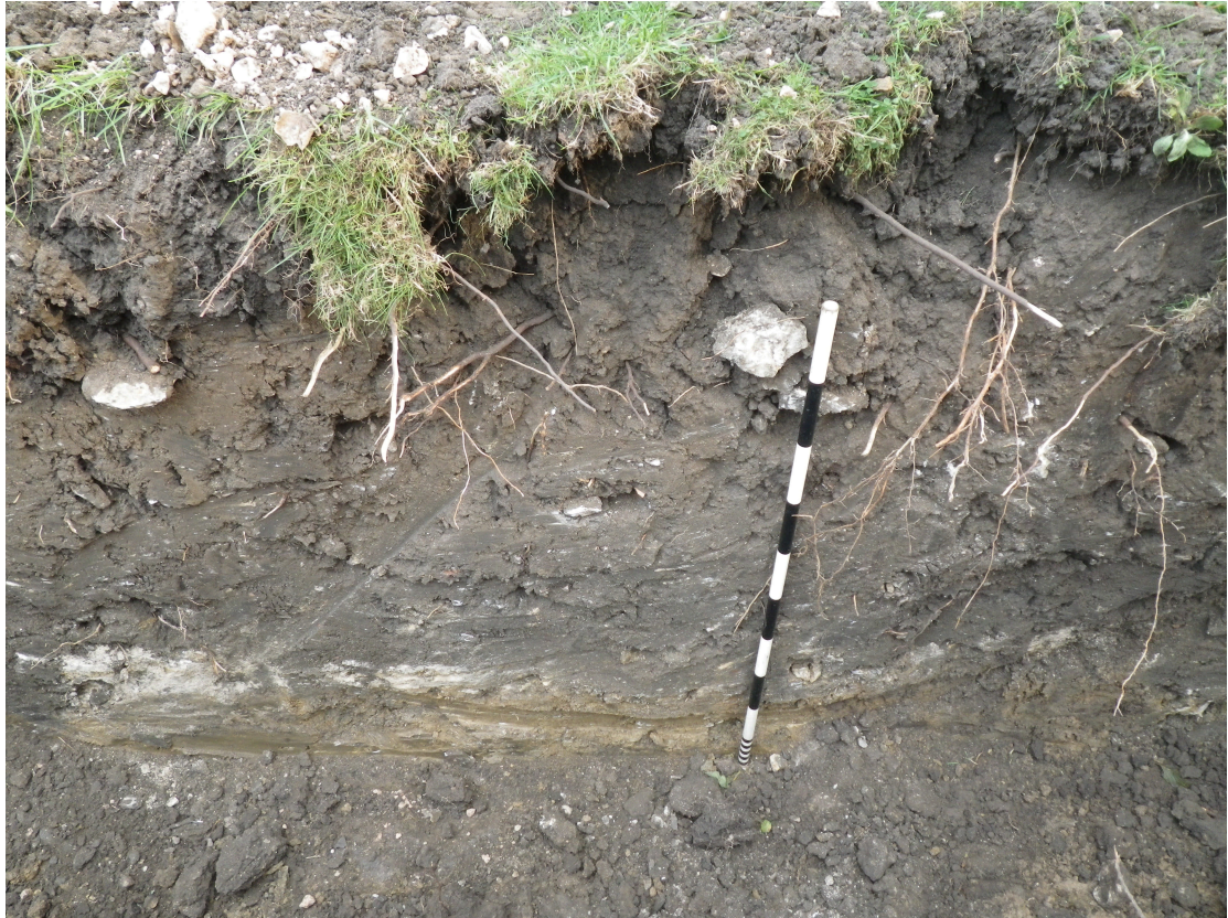
Plate 5 Contexts (2001)-(2004) in the extension foundation trenches
