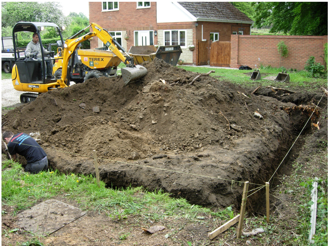
Plate 2 The garage foundation trenches viewed from the south-east
