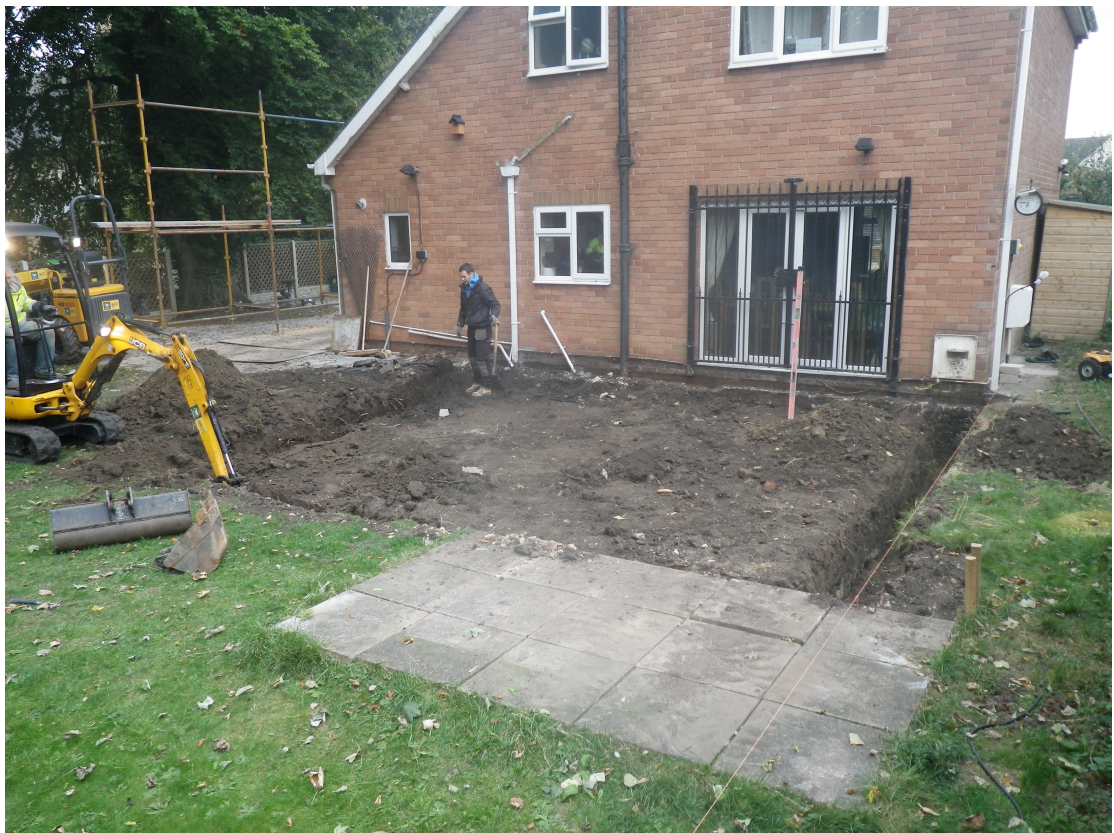
Plate 4 The extension foundation trenches viewed from the north-west
