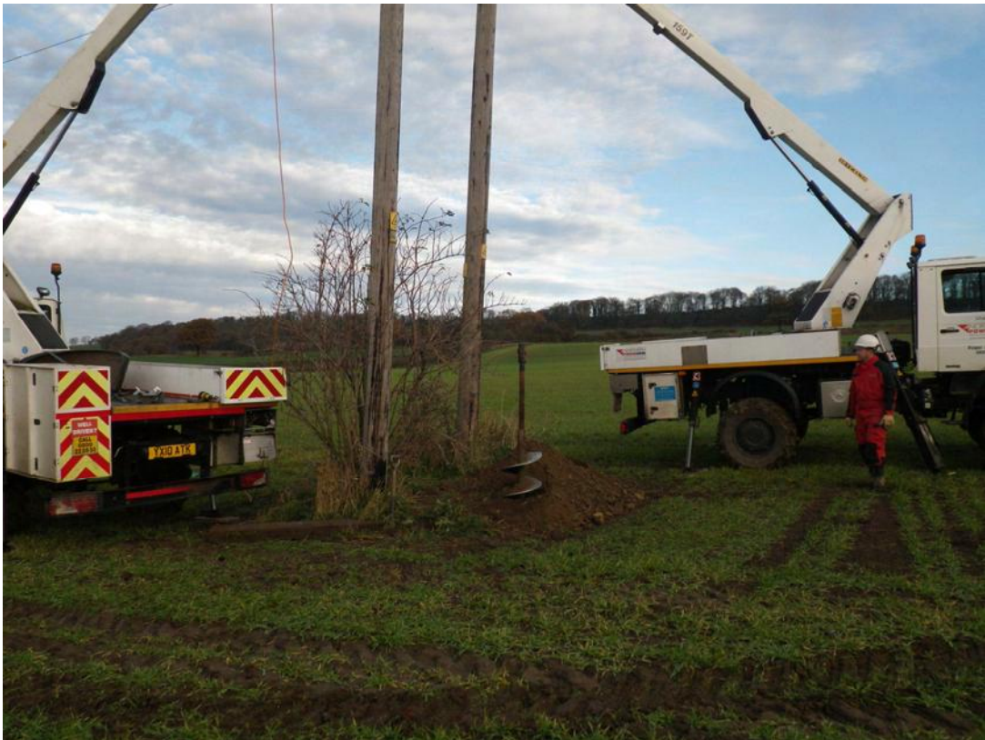
Plate 2 Drilling the replacement pole locations, looking north
