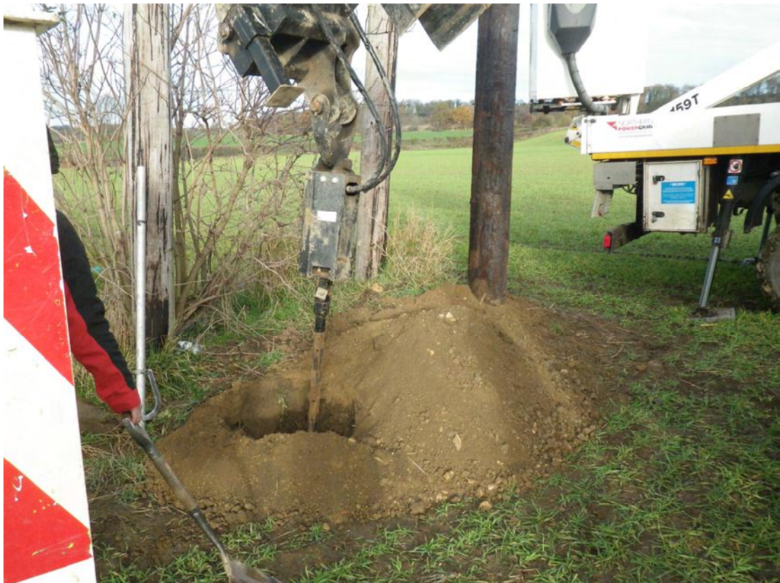
Plate 4 Drilling the second pole replacement position, looking north
