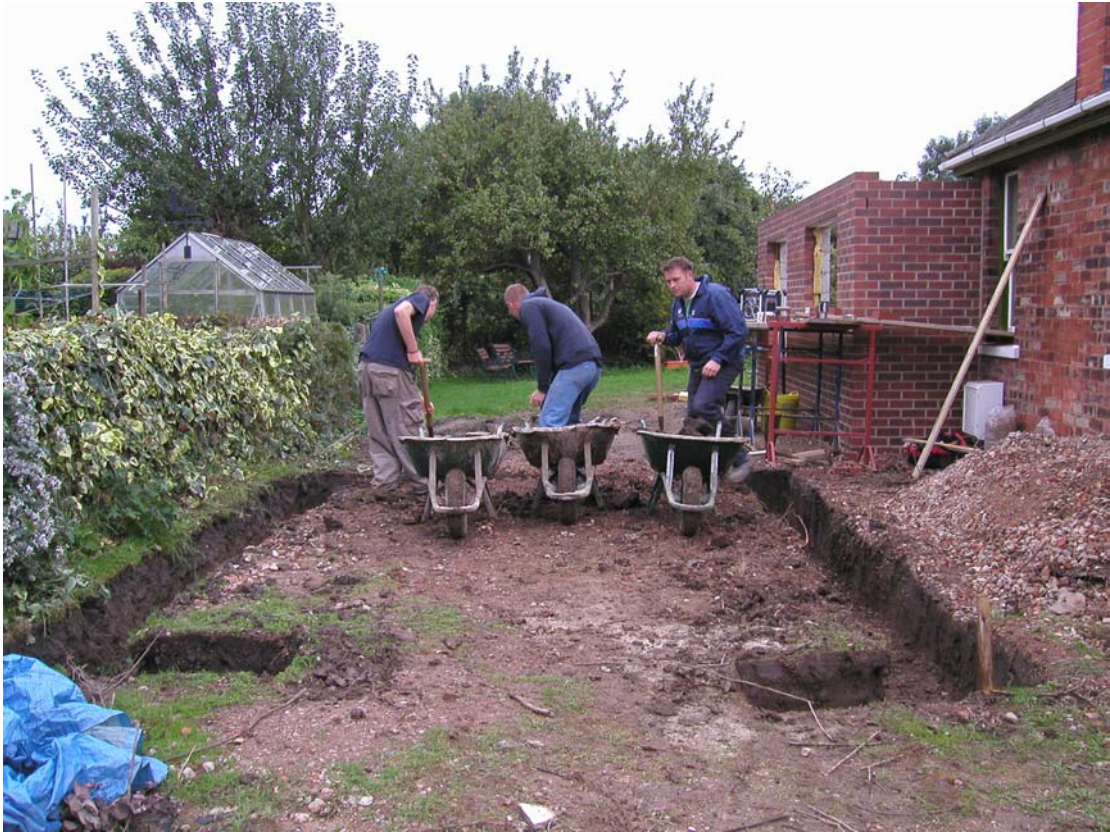
Plate 5 The excavation of the new garage foundations, viewed from the north-east.
