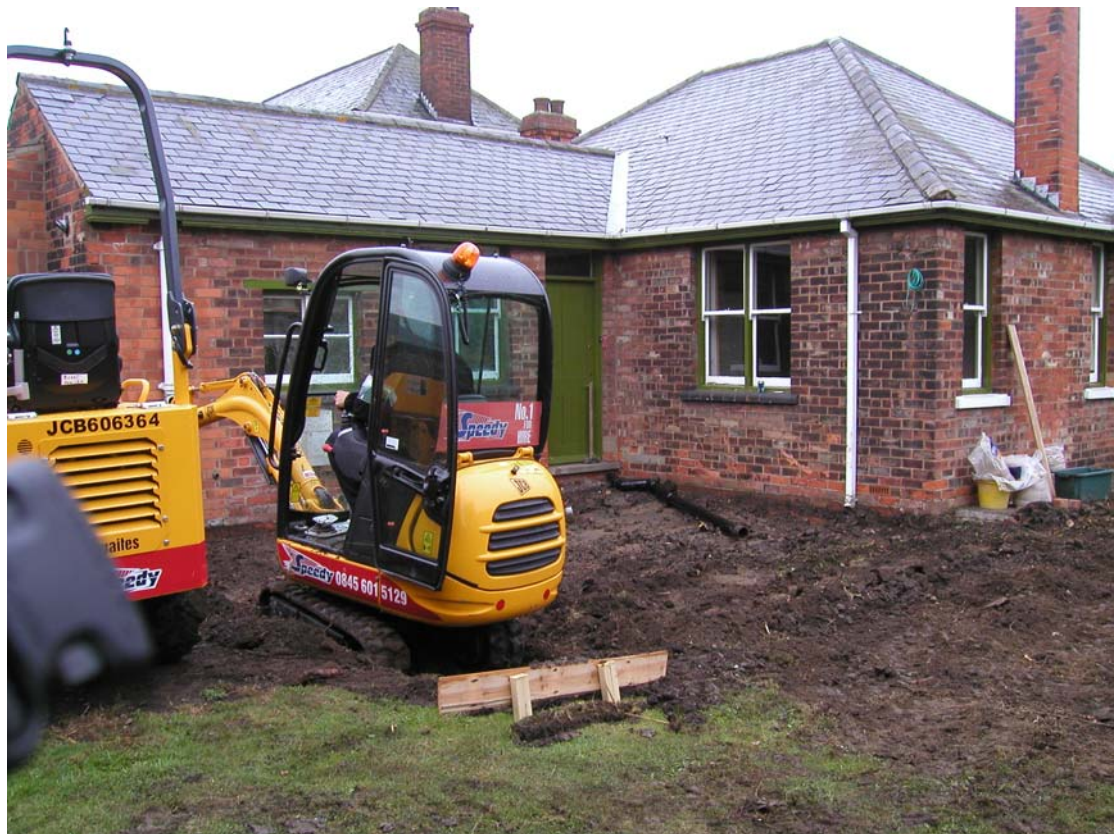
Plate 3 The north-western extension foundation trenches, looking north-east.
