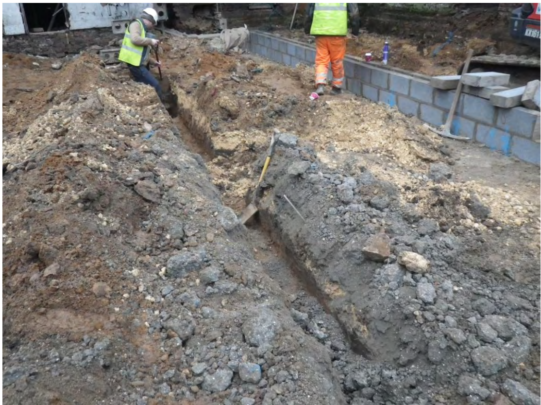
Plate 8 Drainage excavation in the eastern area of the site, looking south-west
