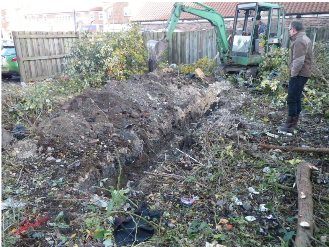
Plate 2 Excavation of the planning continuation trench, viewed from the west
