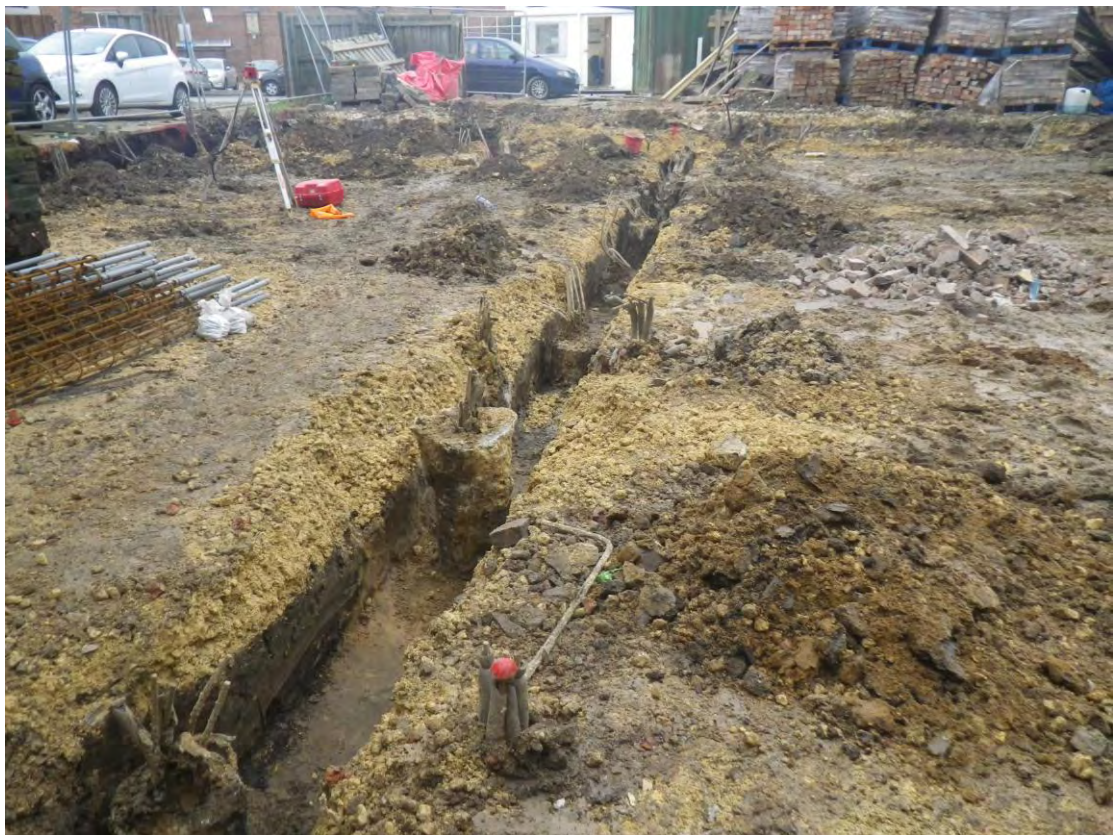
Plate 6 The central N-S aligned beam slot trench, looking north
