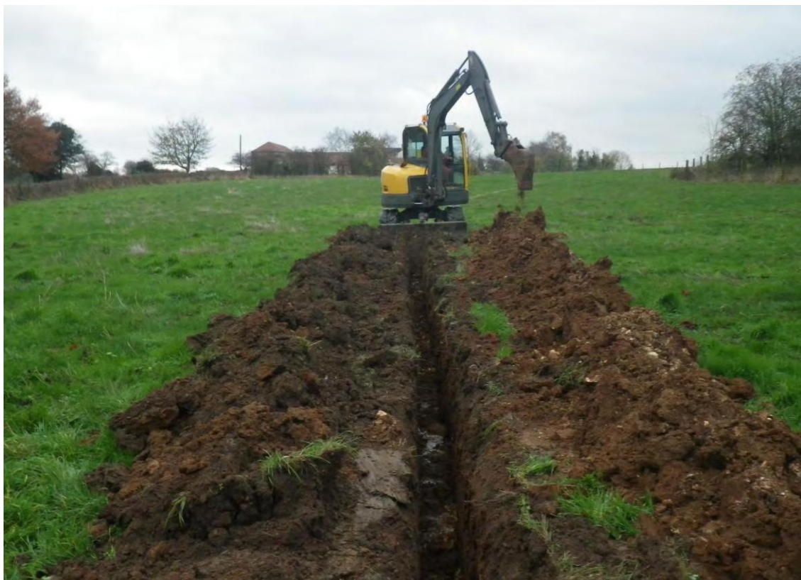
Plate 2 The most westerly part of the trench viewed from the west
