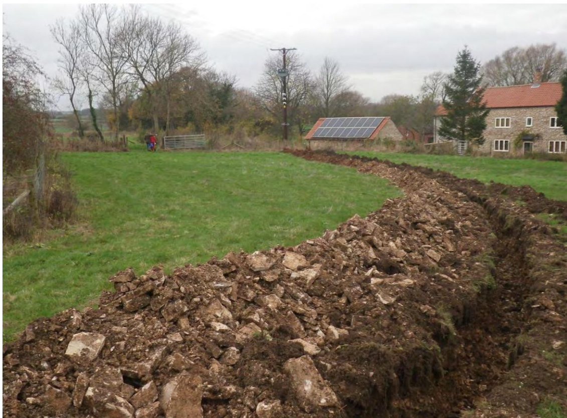
Plate 6 The bulk of the trench viewed from the south-east
