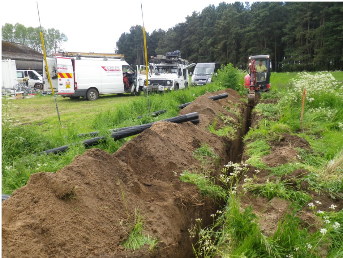
Plate 6 Field 3 cable trench viewed from the north-east
