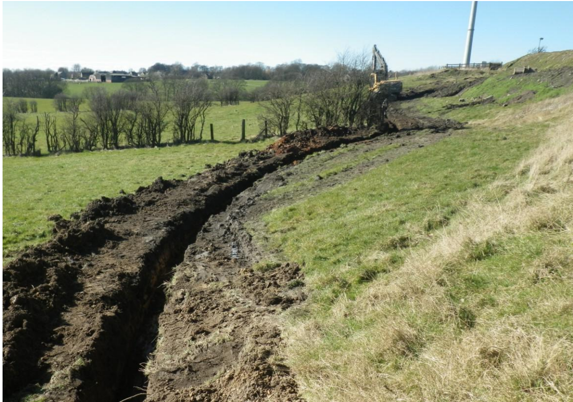
Plate 3 Easternmost portion of the main cable trench viewed from the south-east
