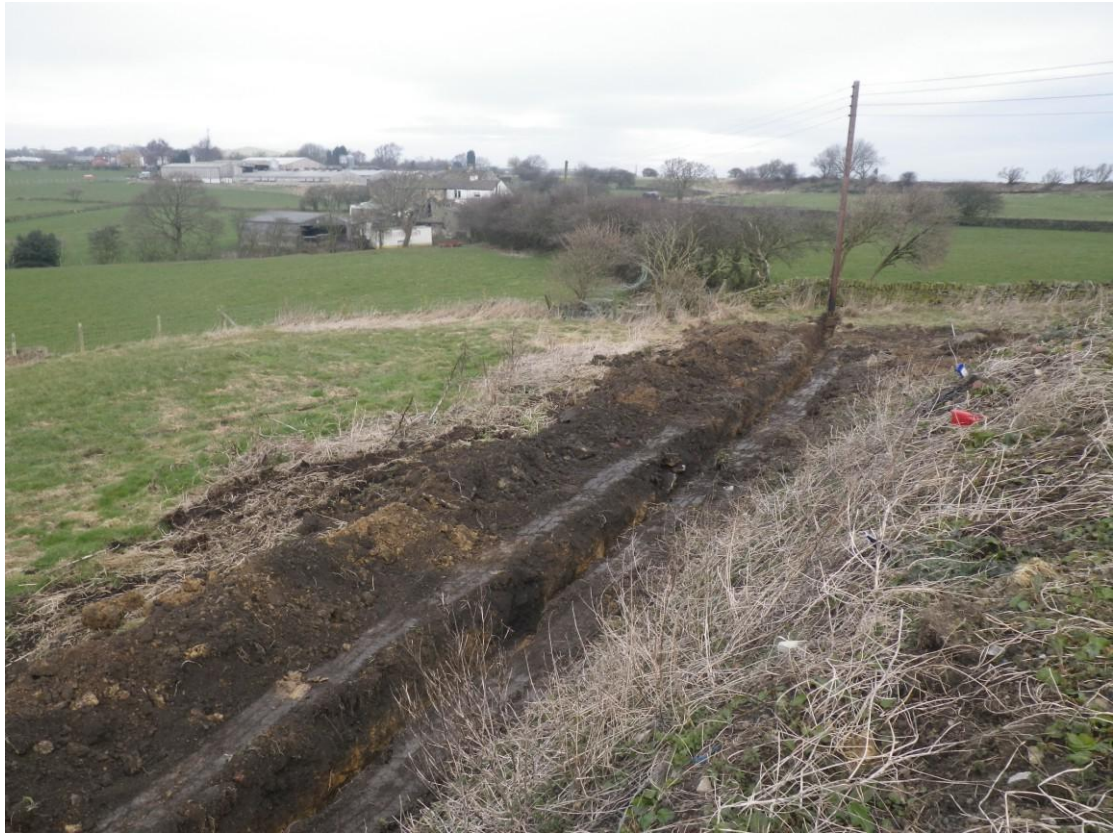
Plate 7 The western portion of the cable trench viewed from the east
