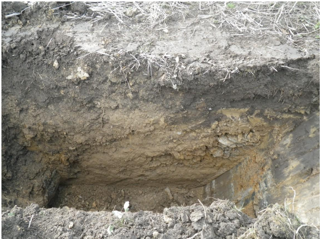
Plate 8 The pole stay trench viewed from the east
