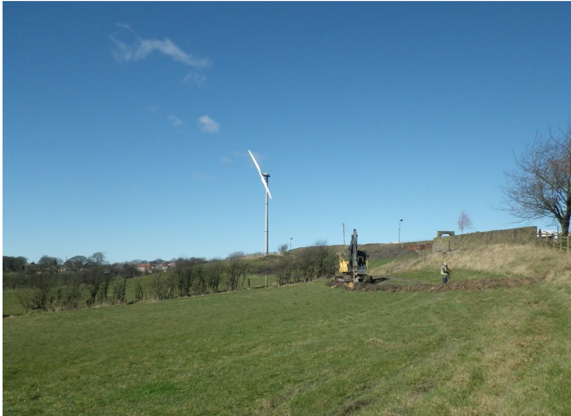
Plate 1 General view of the site from the south-east
