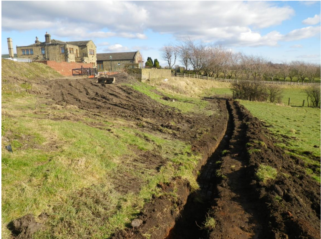
Plate 5 The central portion of the cable trench viewed from the north-west
