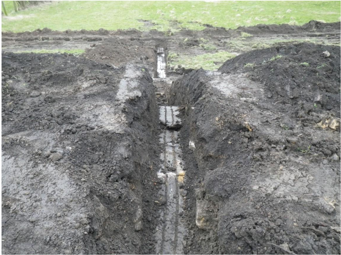
Plate 9 The cable trench spur viewed from the north
