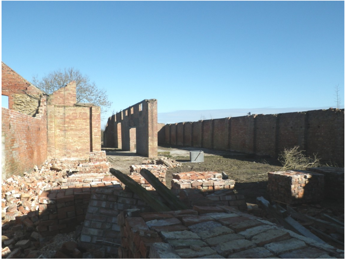
Plate 17 The interior of building 4 viewed from the south
