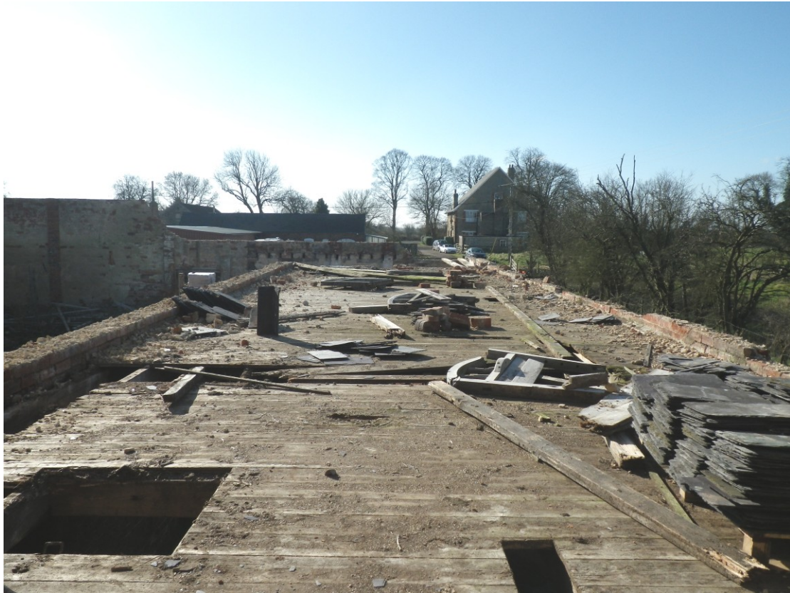
Plate 15 Building 3 at first-floor level as viewed from the north
