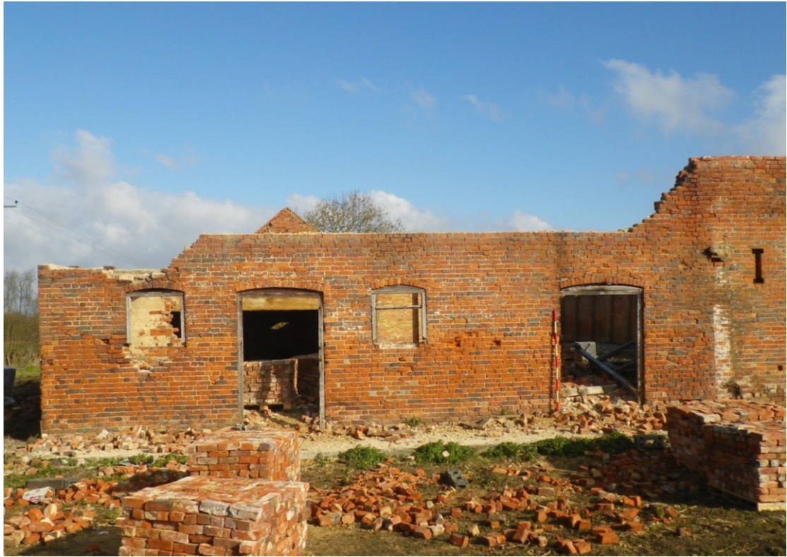
Plate 3 The western part of the south elevation of building 2 (2m scale)
