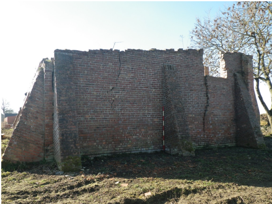
Plate 10 The north elevation of building 4
