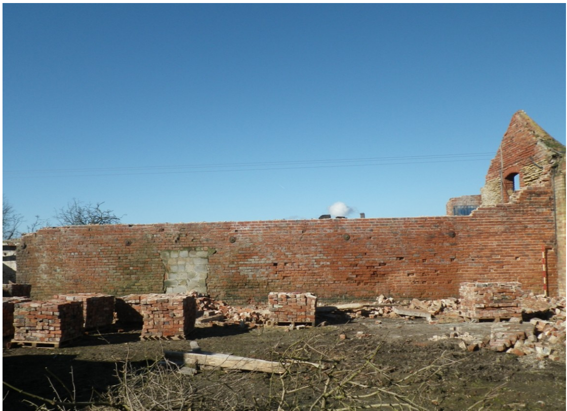
Plate 8 The east elevation of building 3 viewed from within building 4 (2m scale)
