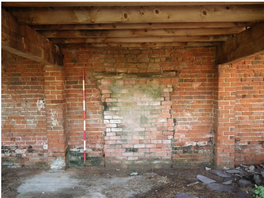
Plate 14 The blocked doorway in the east wall of the ground floor of building 3 viewed from the west (2m scale)
