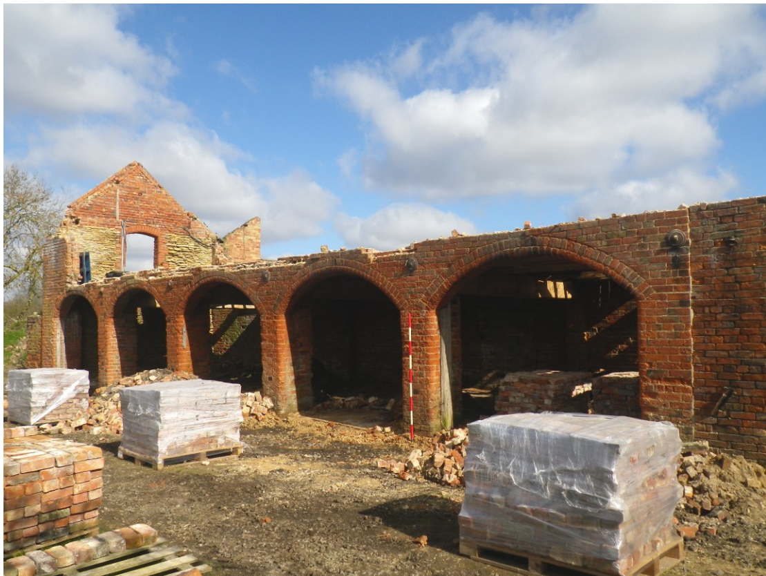
Plate 6 The west elevation of building 3 viewed from the south-west (2m scale)
