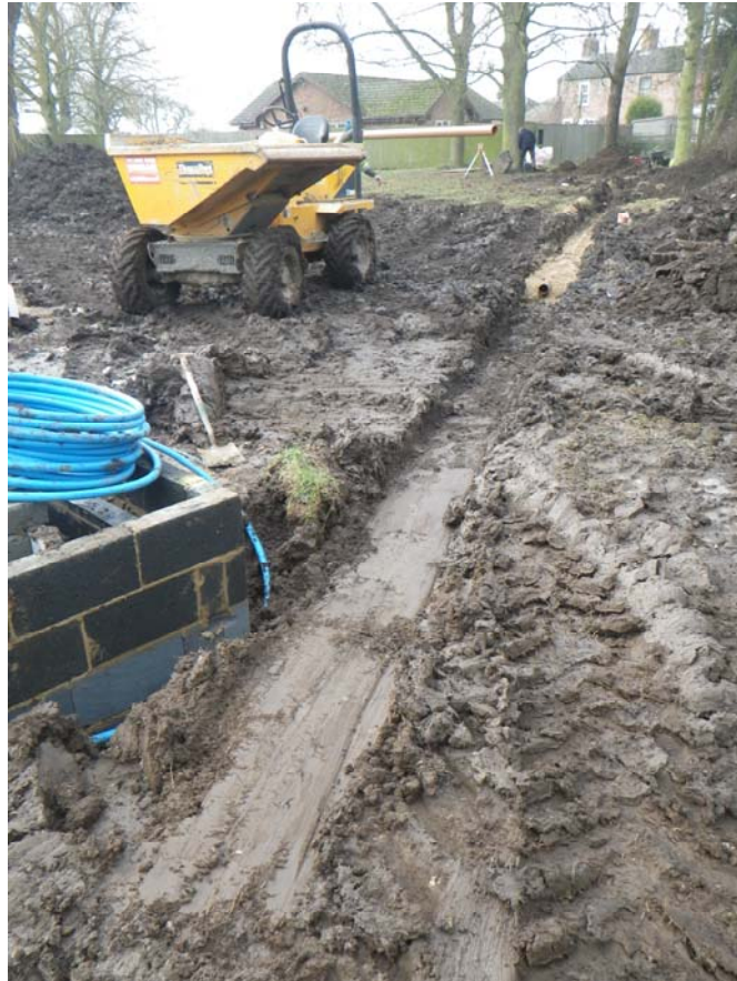
Plate 4 The main service/waste trench, looking NW
