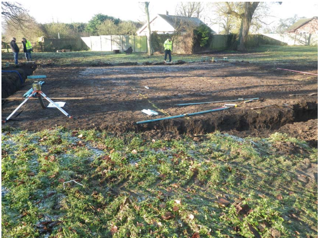
Plate 2 The outer edges of the plot during excavation, looking W
