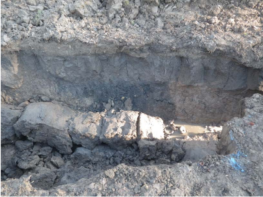
Plate 3 Showing the collapse area in the E corner of the trenches, looking NE
