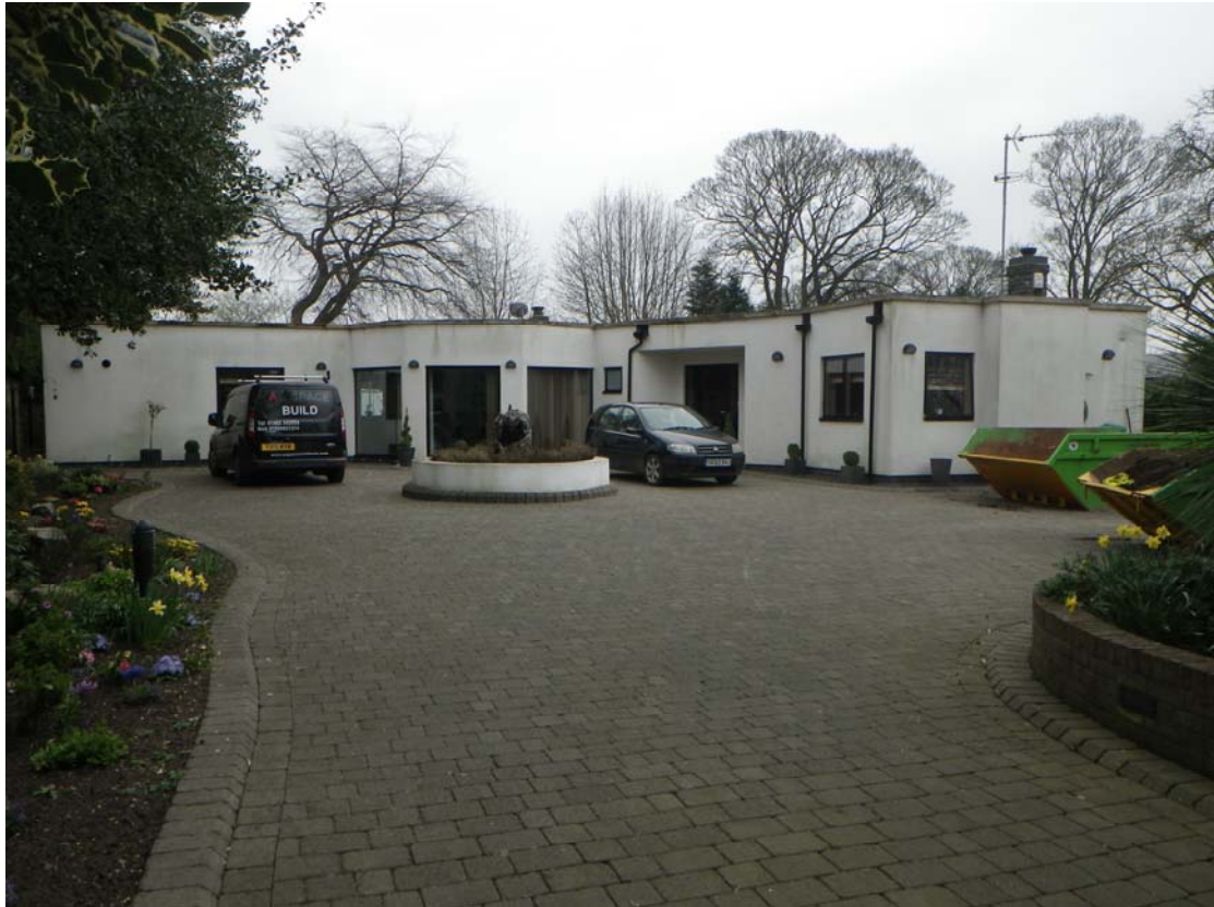
Plate 1 The site of the development from the entrance, looking E
