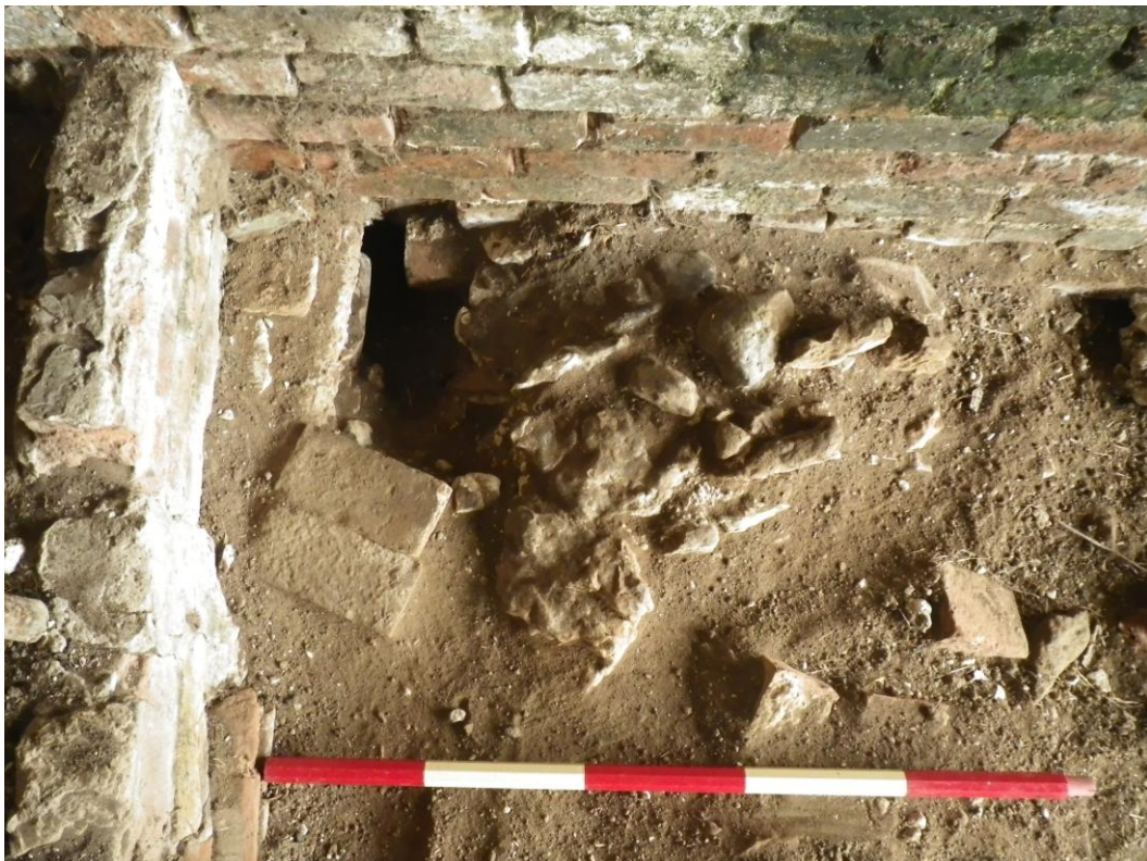
Plate 30 Exposed drain adjacent to the east end of the feeding trough (1m scale)
