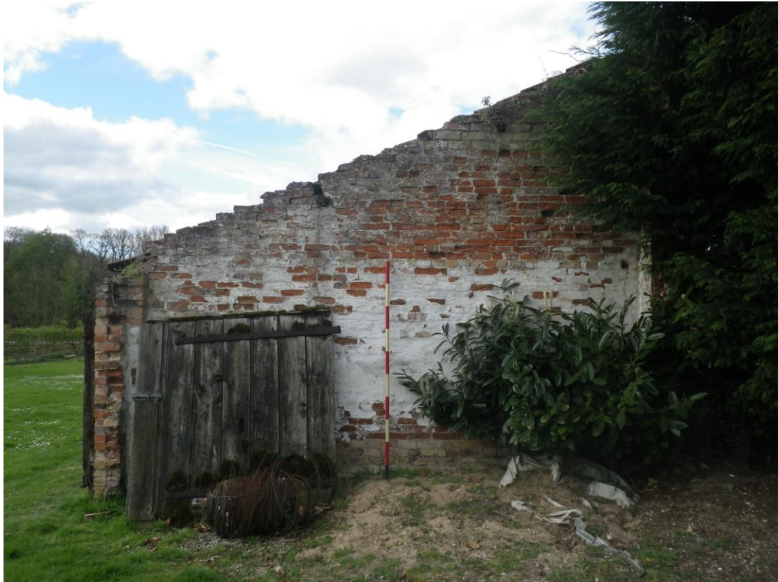
Plate 11 The east elevation (2m scale)
