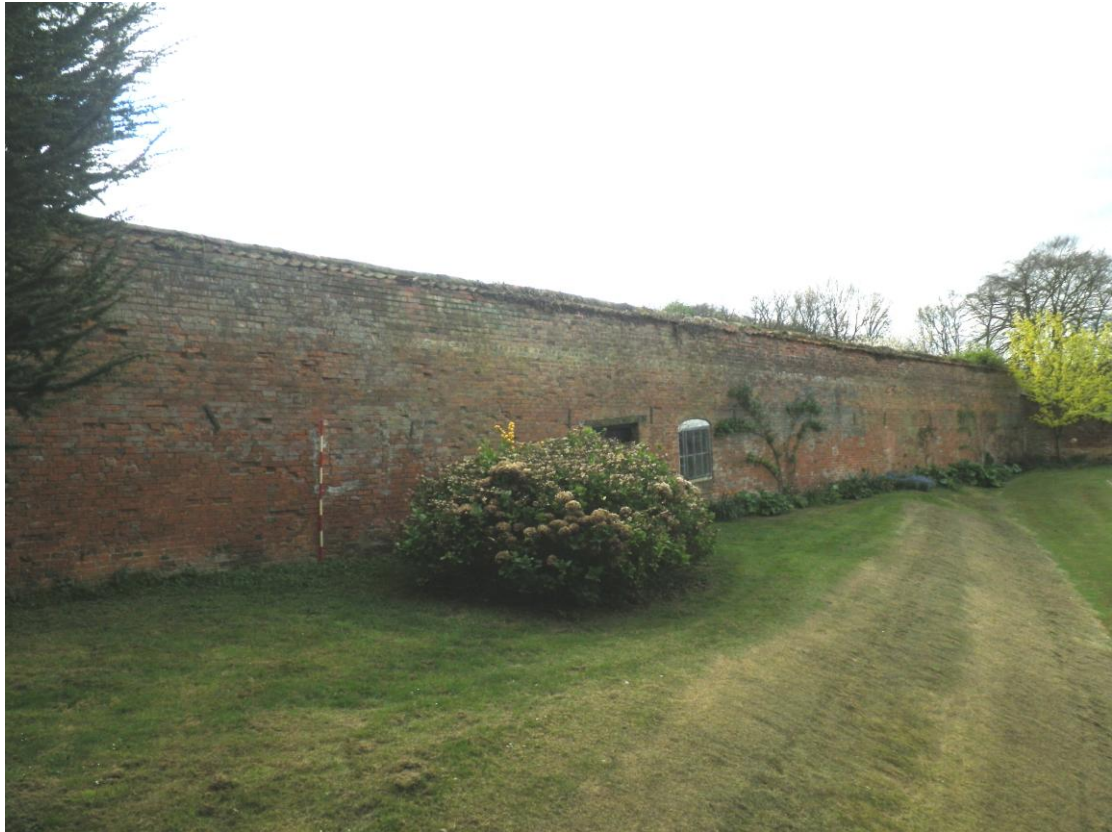
Plate 7 The north elevation viewed from the north-east
