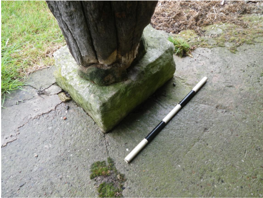
Plate 19 The stone base for the beam 1 post (0.5m scale)
