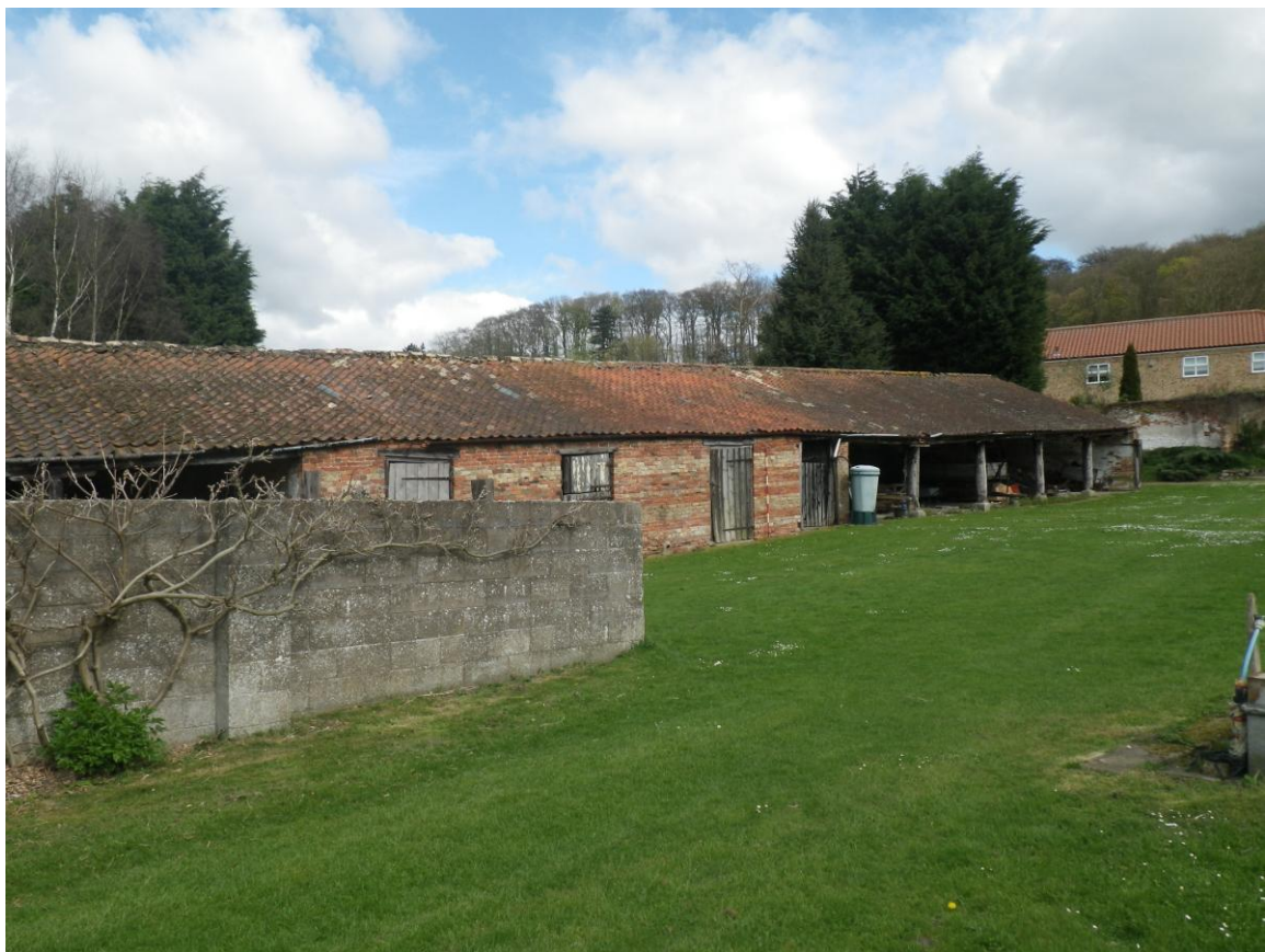
Plate 2 General view of the building from the south (2m scale)
