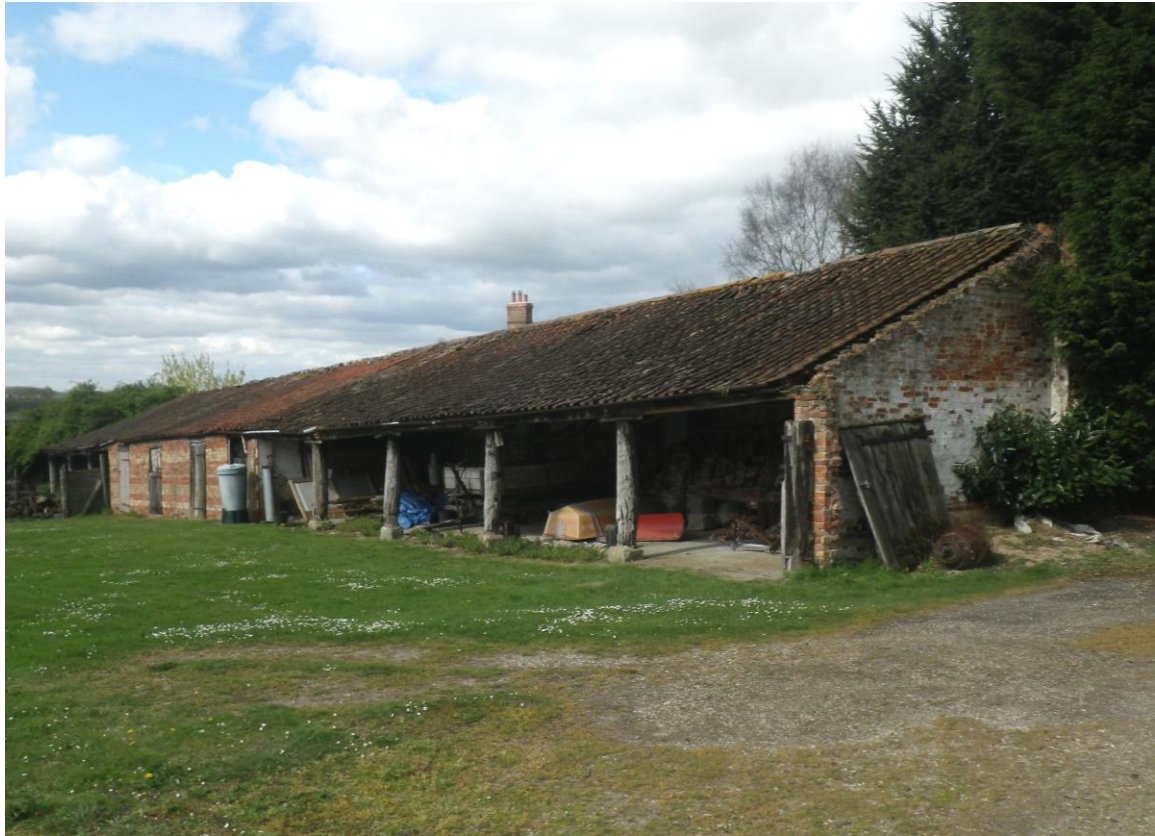
Plate 1 General view of the building from the east (2m scale)
