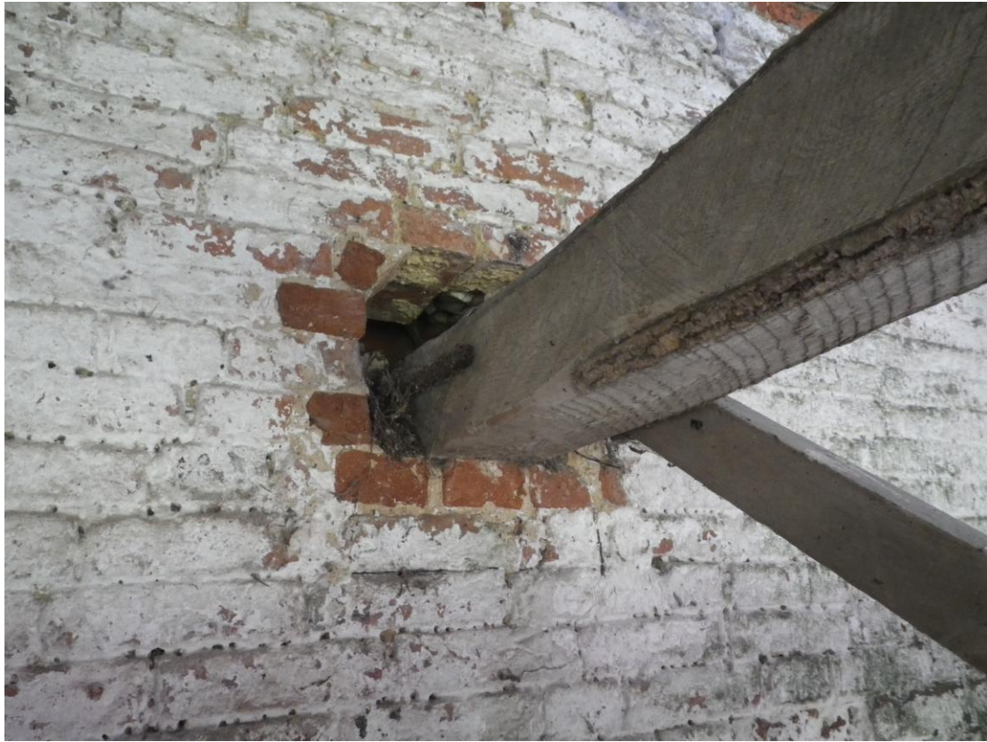
Plate 17 Setting in the north wall for beam 3 viewed from the south
