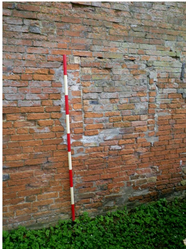
Plate 10 Blocked window (?) in the northern part of the north elevation (2m scale)
