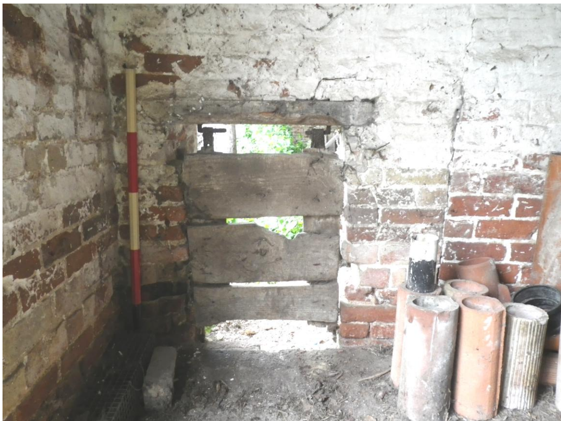
Plate 26 Wooden hatch suspended from lintel in the south corner of the room (1m scale)
