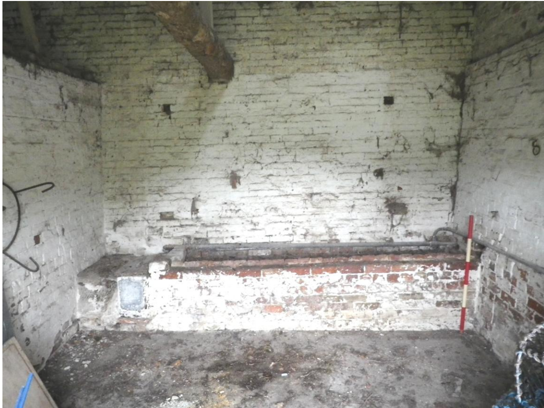
Plate 23 Room 2 viewed from the south-east (1m scale)
