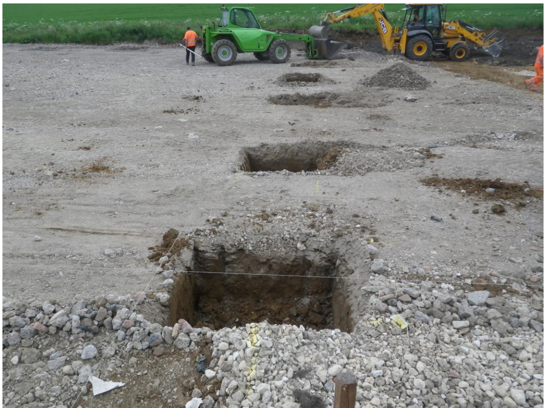
Plate 10: Foundation pits along the west side of the building, looking south
