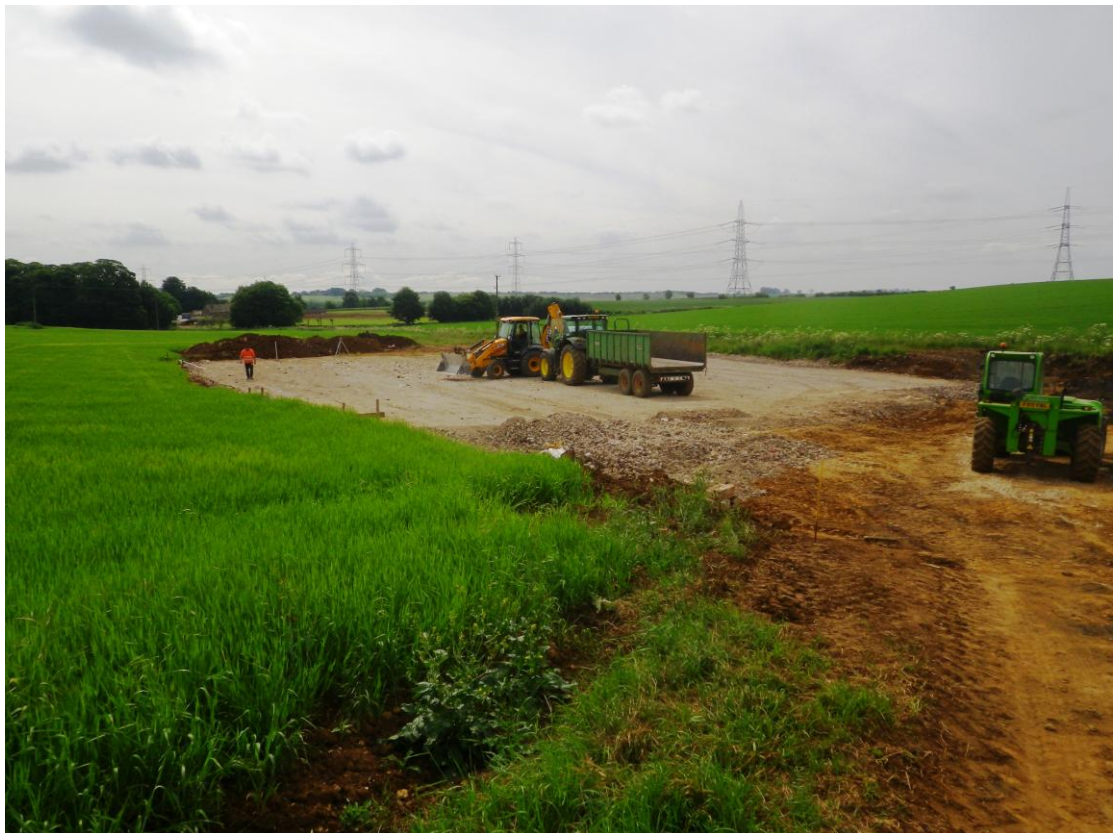
Plate 6: Site stripped and stoned-up, looking south-east
