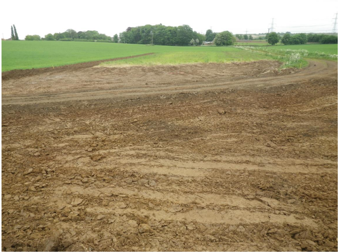
Plate 3: Ground reduction completed over the western part of the site
