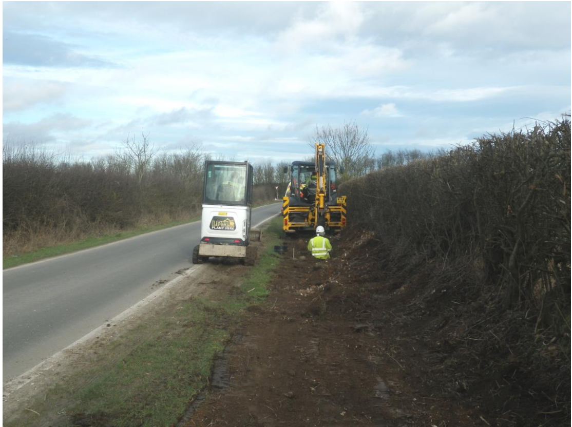
Plate 25 The Bonby Lane trenching comes to an end, looking north-east
