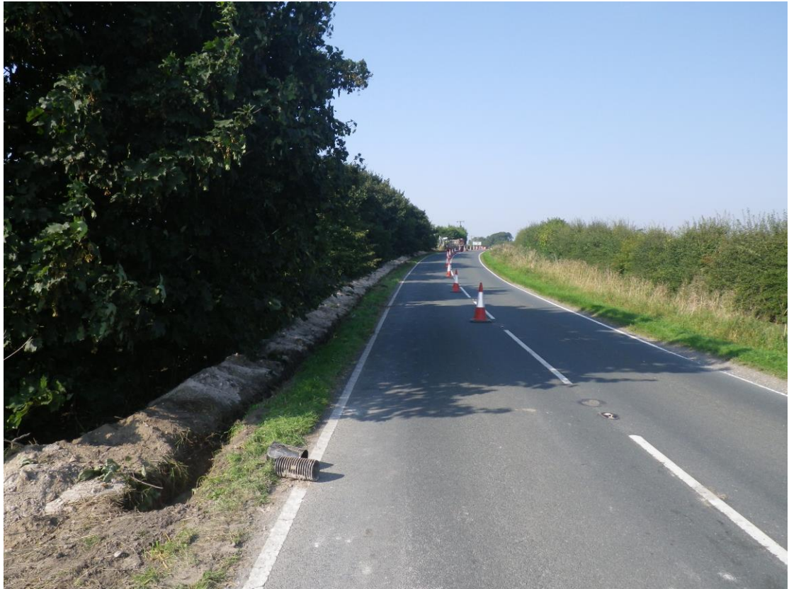
Plate 21 The B1206 trench looking north towards the junction with the A15
