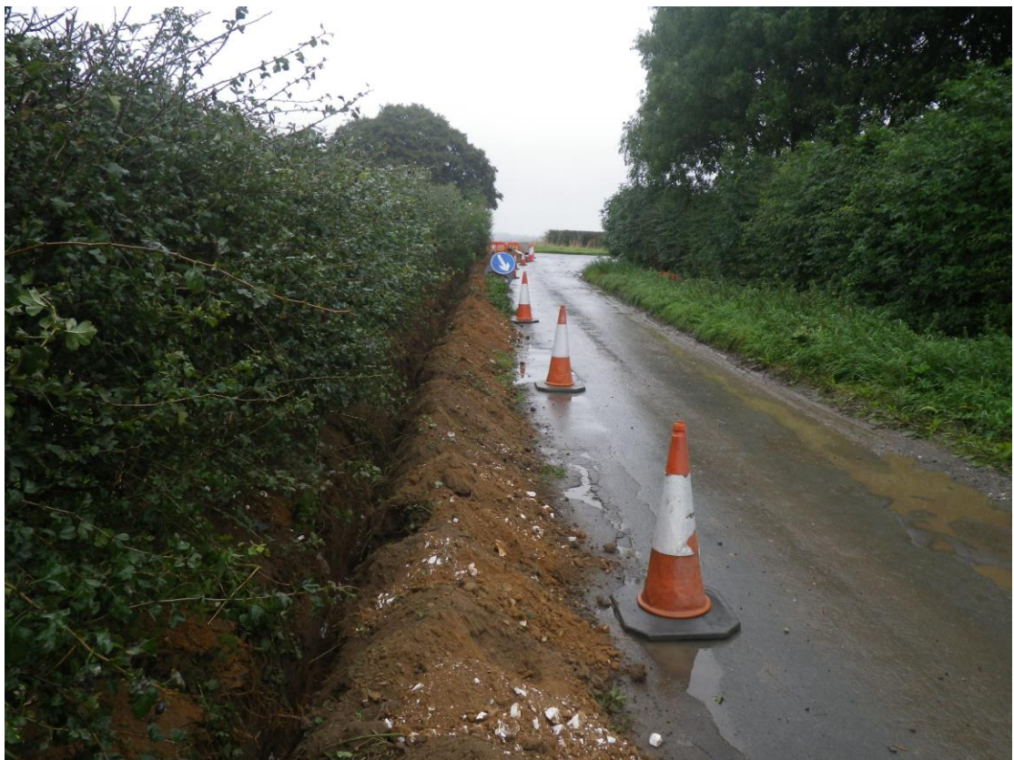
Plate 18 The cable trench alongside Wold Road looking north-east
