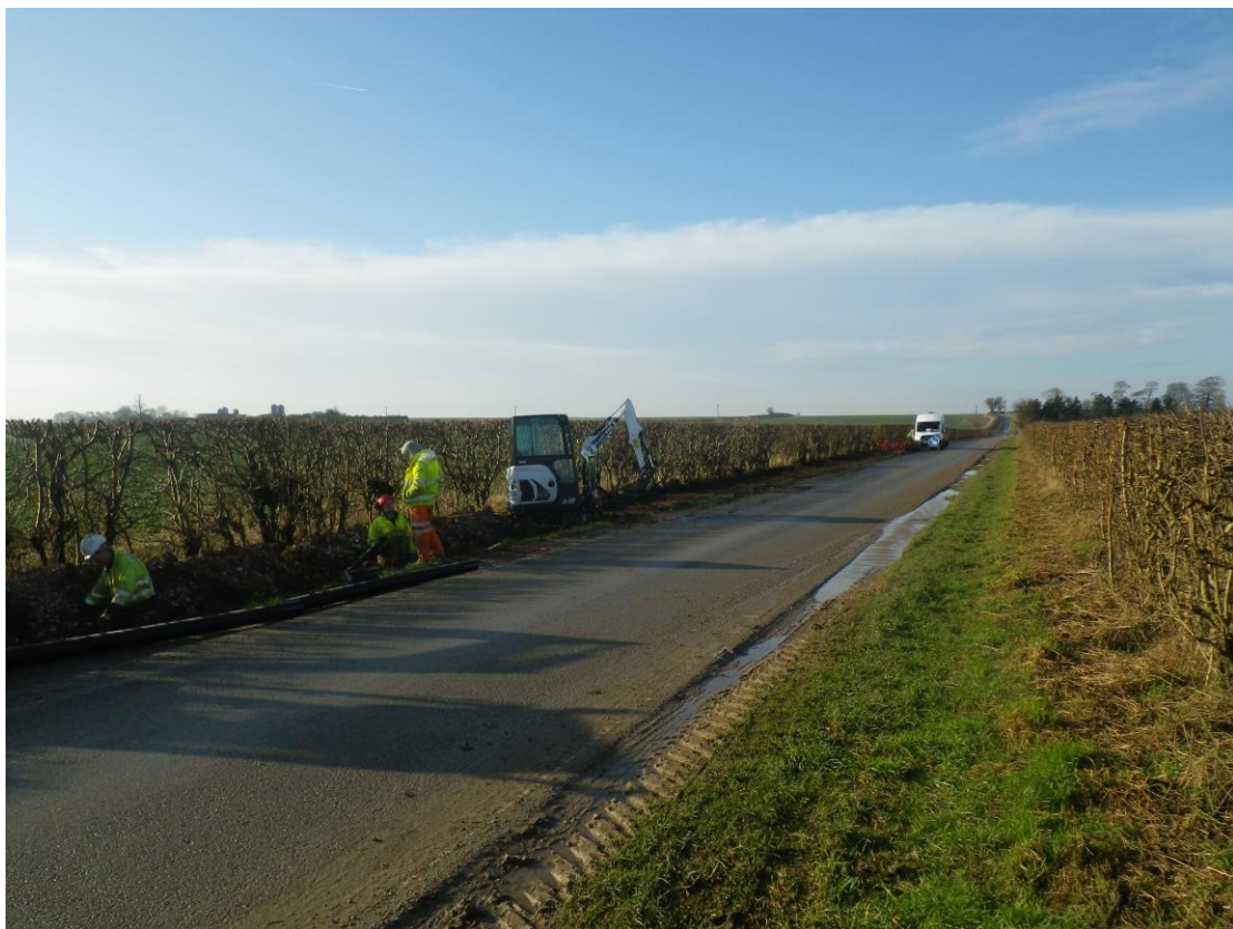
Plate 24 The central portion of the Bonby Lane trench looking south
