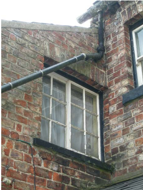
Plate 3 Bathroom window with north-south wall part covering the west reveal, looking south-west
