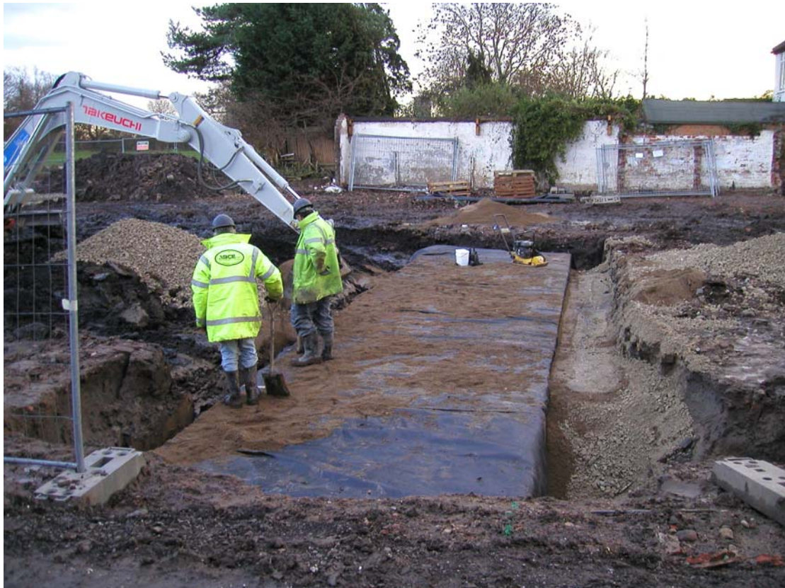
Plate 23 The Aquacell water storage tank in position, looking south
