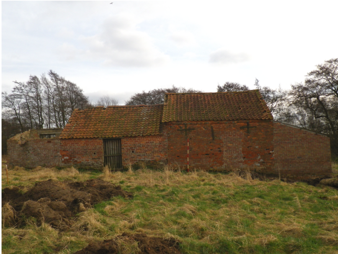
Plate 7 General view of the building from the north (2m scale)
