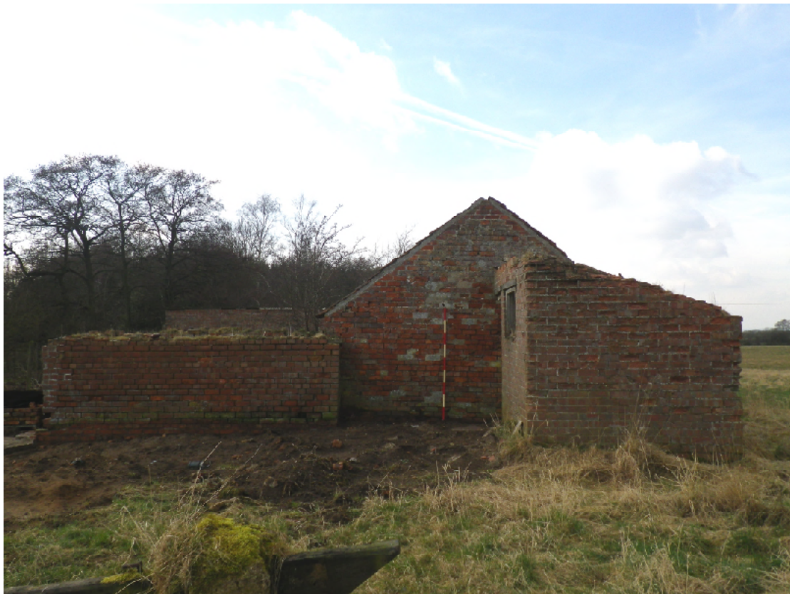
Plate 6 East facing elevations of Rooms 2, 3 and 4 (2m scale)
