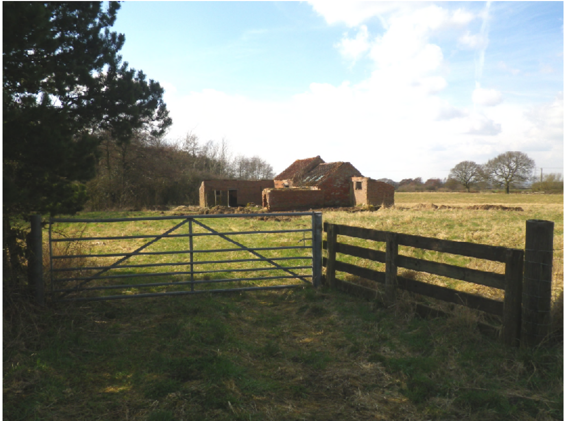
Plate 1 General view of the building from the south-east
