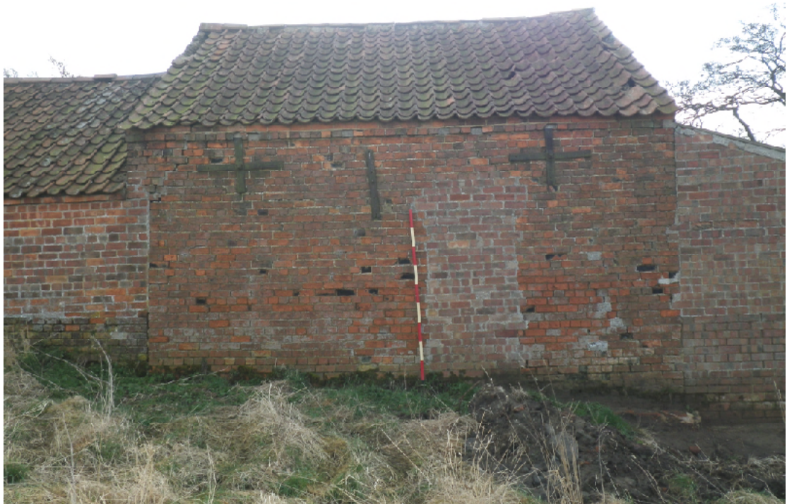
Plate 9 North facing elevation of Room 1 (2m scale)
