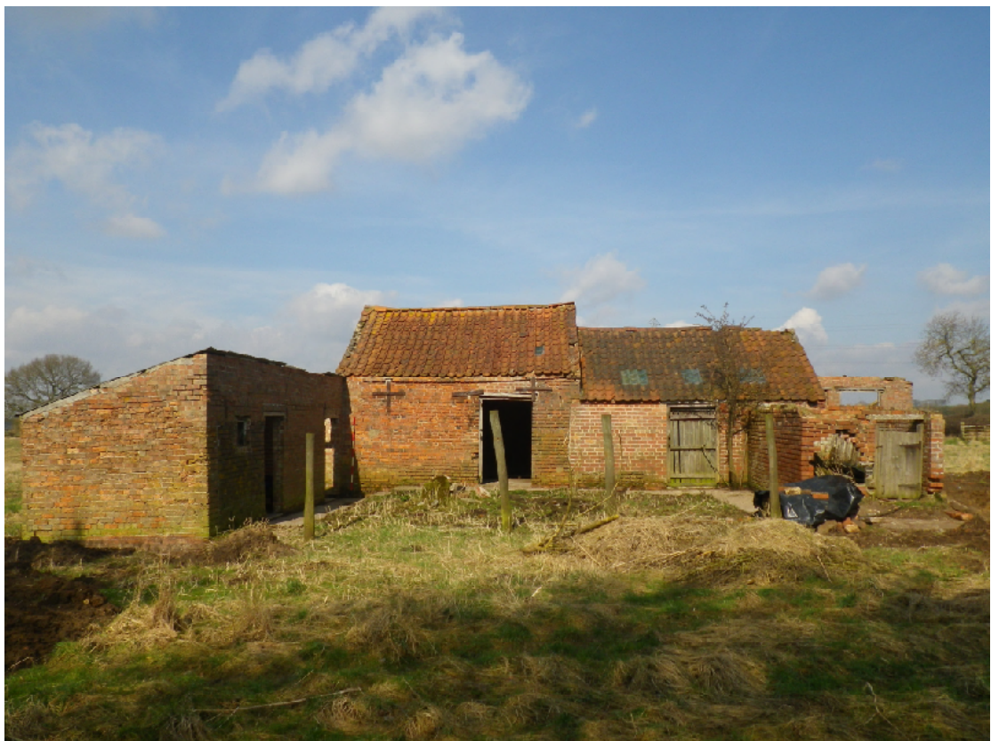
Plate 2 General view of the building from the south
