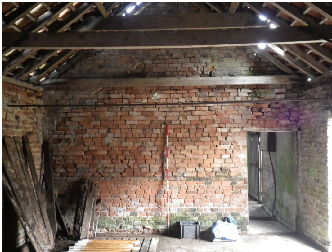
Plate 16 East wall in Room 1 (2m scale)
