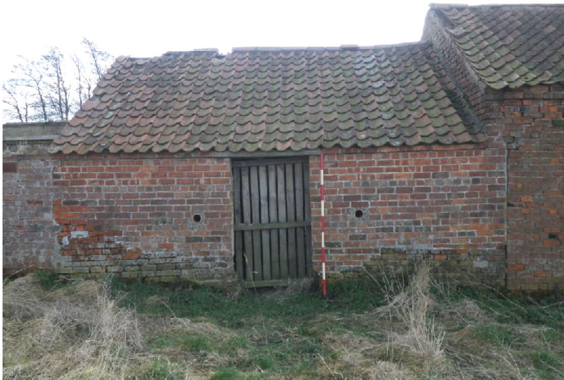
Plate 8 North facing elevation of Room 2 (2m scale)
