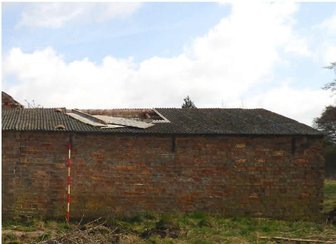
Plate 12 West facing elevation of Room 6 (2m scale)
