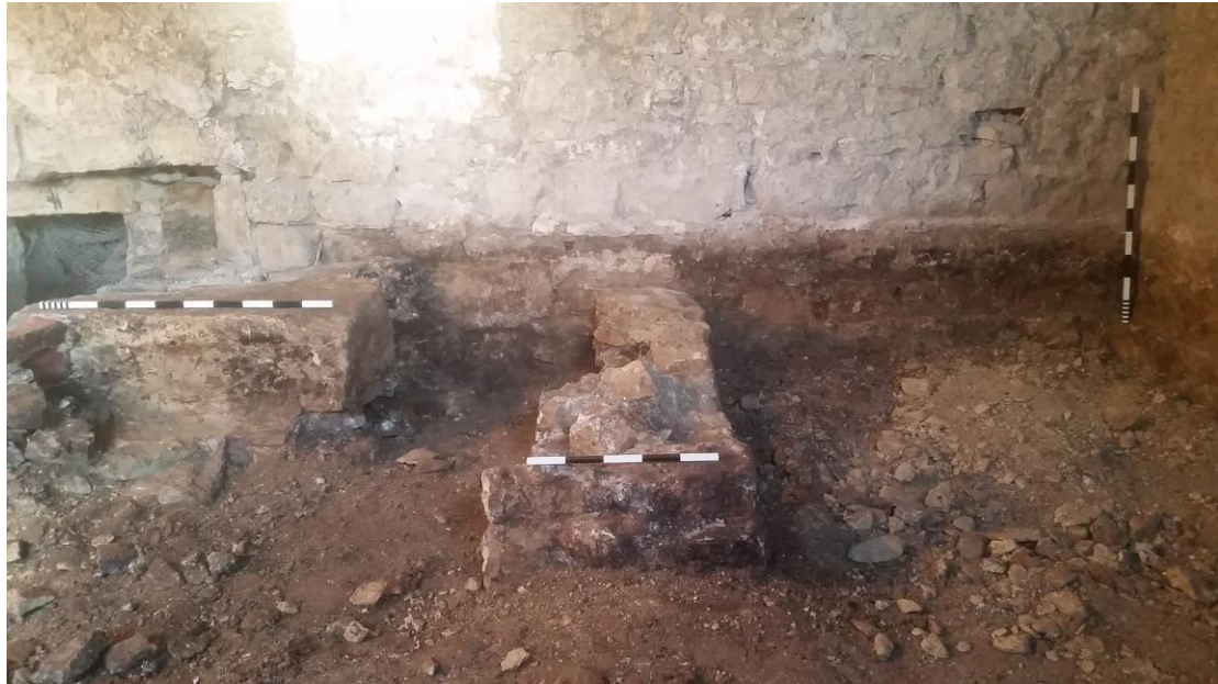
Plate 9 Interior dividing wall foundation remnant 111, oriented south-east – north-west, and overlying an earlier foundation. Looking north-west, 0.5m and 1m scales
