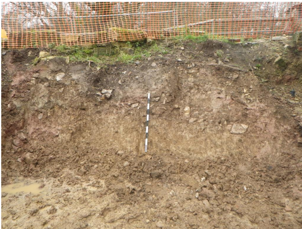
Plate 31 View of the truncated bank to the west of the mill, showing the upper construction cuts associated with the mill, looking north, 1m scale
