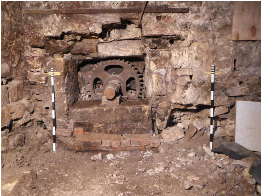
Plate 4 North-west layshaft, showing several alterations and insertions, following removal of Slot 1. Looking north, 1m scales
