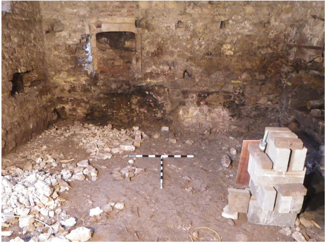
Plate 13 Full ground reduction in the mill interior, looking west, 1m scales
