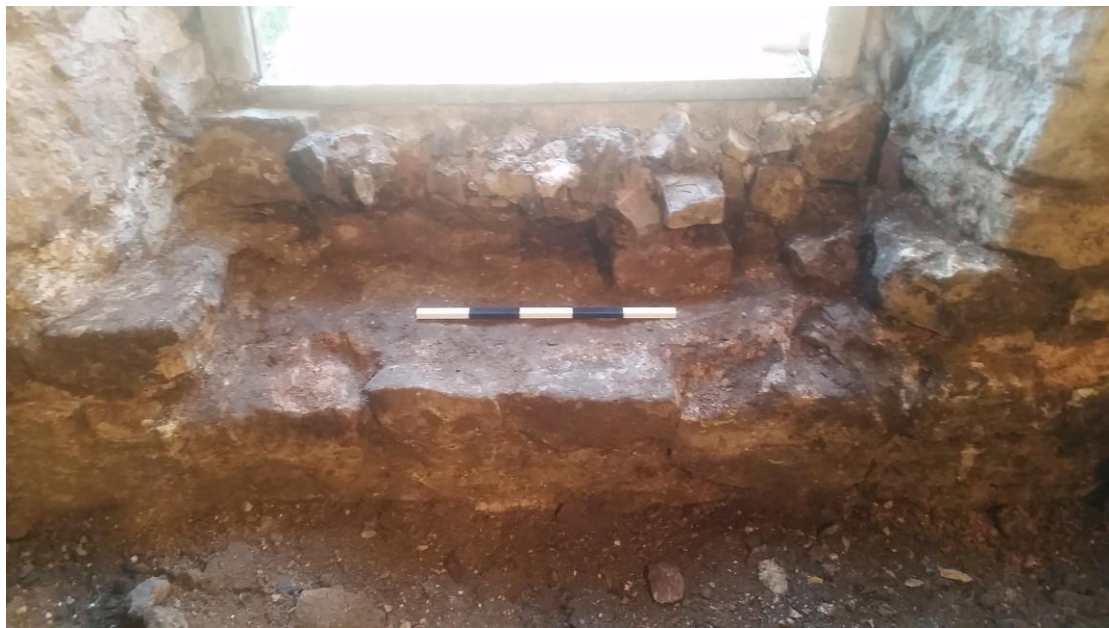
Plate 16 The central, southern doorway to the mill, from the interior, looking south, 0.5m scale
