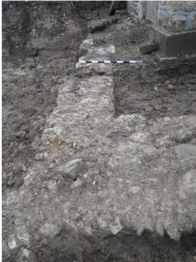
Plate 33 Wall 116 shown in association with the current mill wall foundations, looking north, 1m scale
