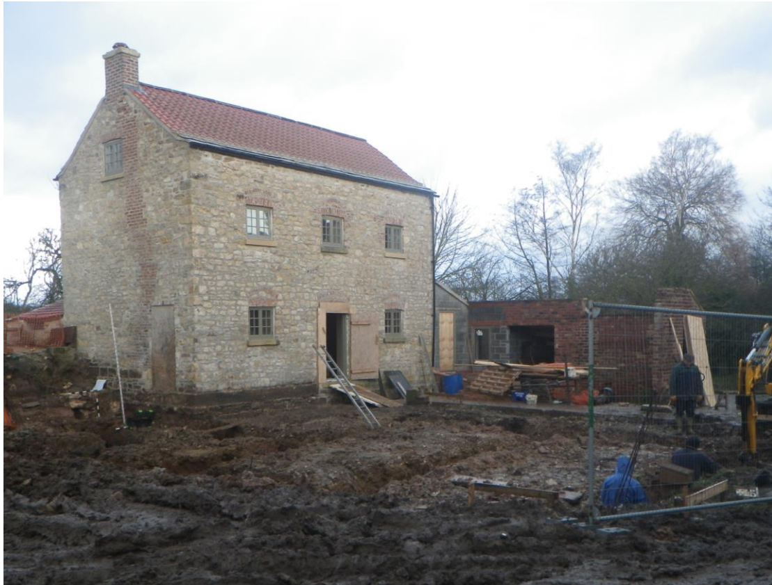
Plate 1 Norton Watermill, shown from the south-west
