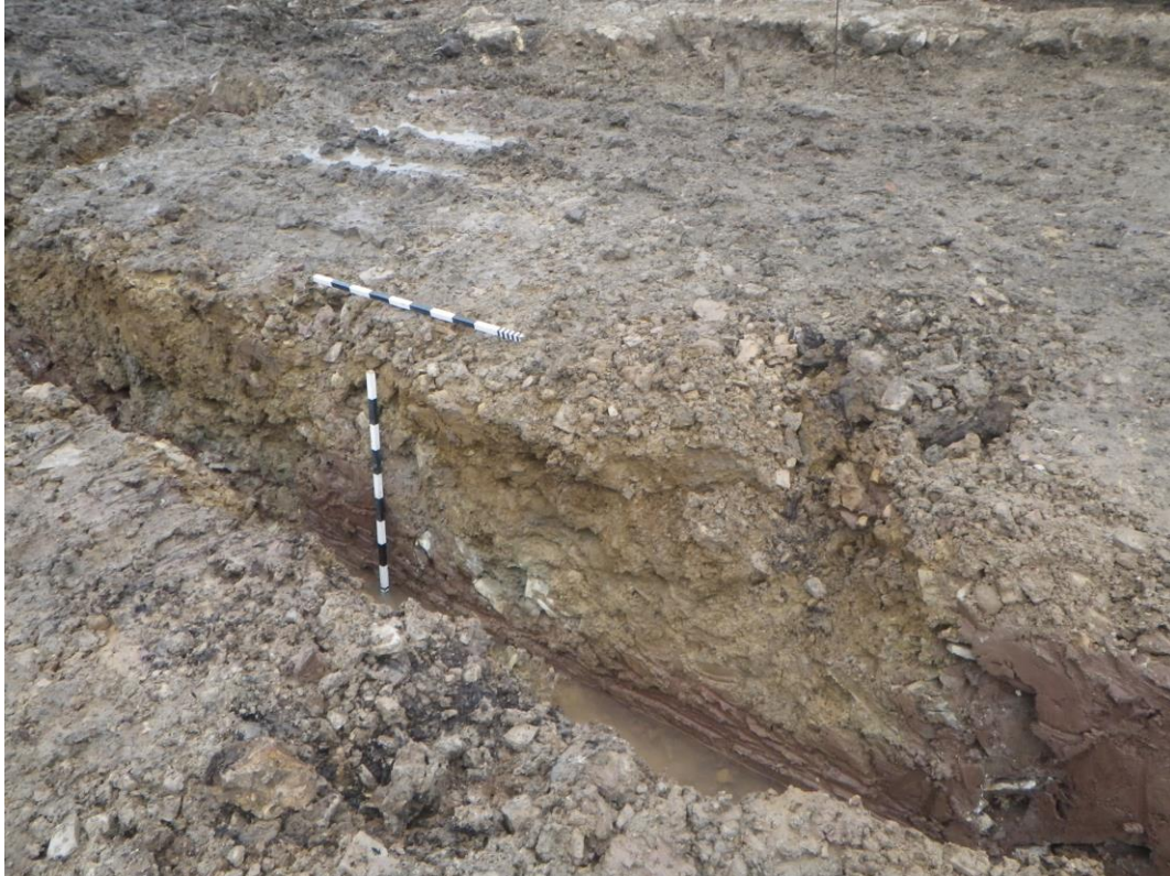
Plate 36 View of the typical stratigraphy in the strip foundation trenches to the south and west of the mill, looking north-west, 1m scales
