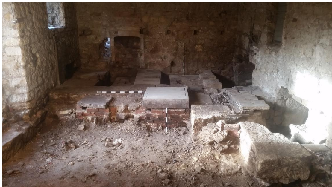
Plate 2 The western interior of the mill, following the removal of all the above floor mill apparatus and flooring and after some initial ground reduction. Wooden trapdoor in centre, leading to Slots 1, 2 and 3 behind and the two layshaft cavities to the right. Fireplace to left rear. Looking west, 1m & 0.5m scales
