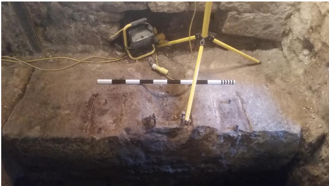
Plate 8 Detail of ironwork bolts for 19 th century layshaft set into earlier stone ashlar-type blocks around Slot 3. Looking south, 1m scale
