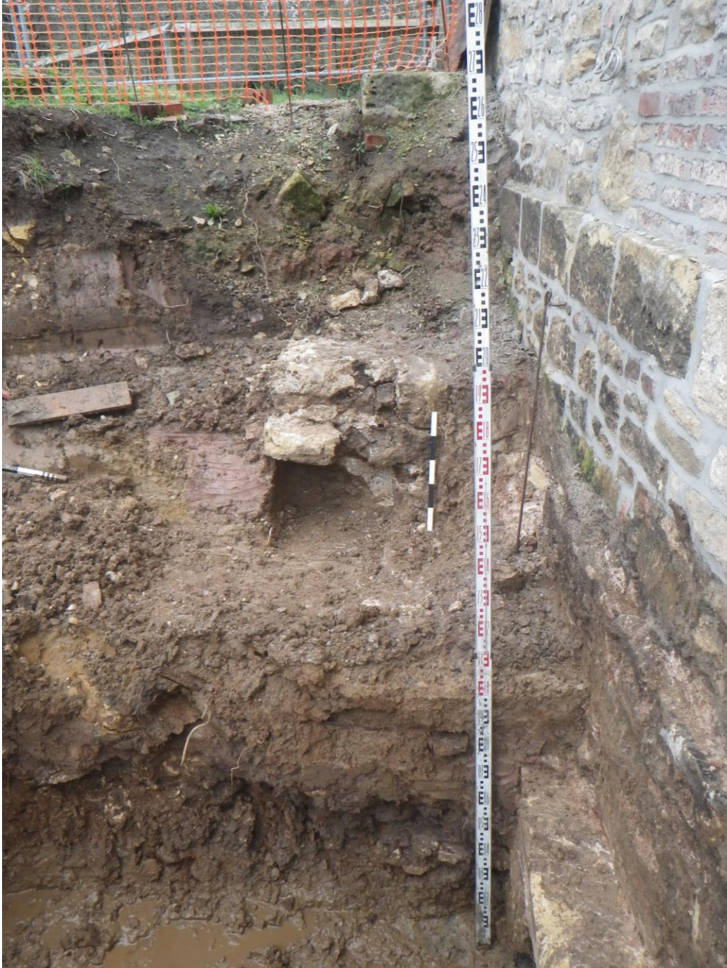
Plate 32 Multi-level shot of the foundations for the early wall 116 (centre) juxtaposed with the early footings 117 (right) of the current mill, with deposits associated with both construction horizons visible both below and to the left. Looking north. 1m scale and surveying staff to height of 2.8m
