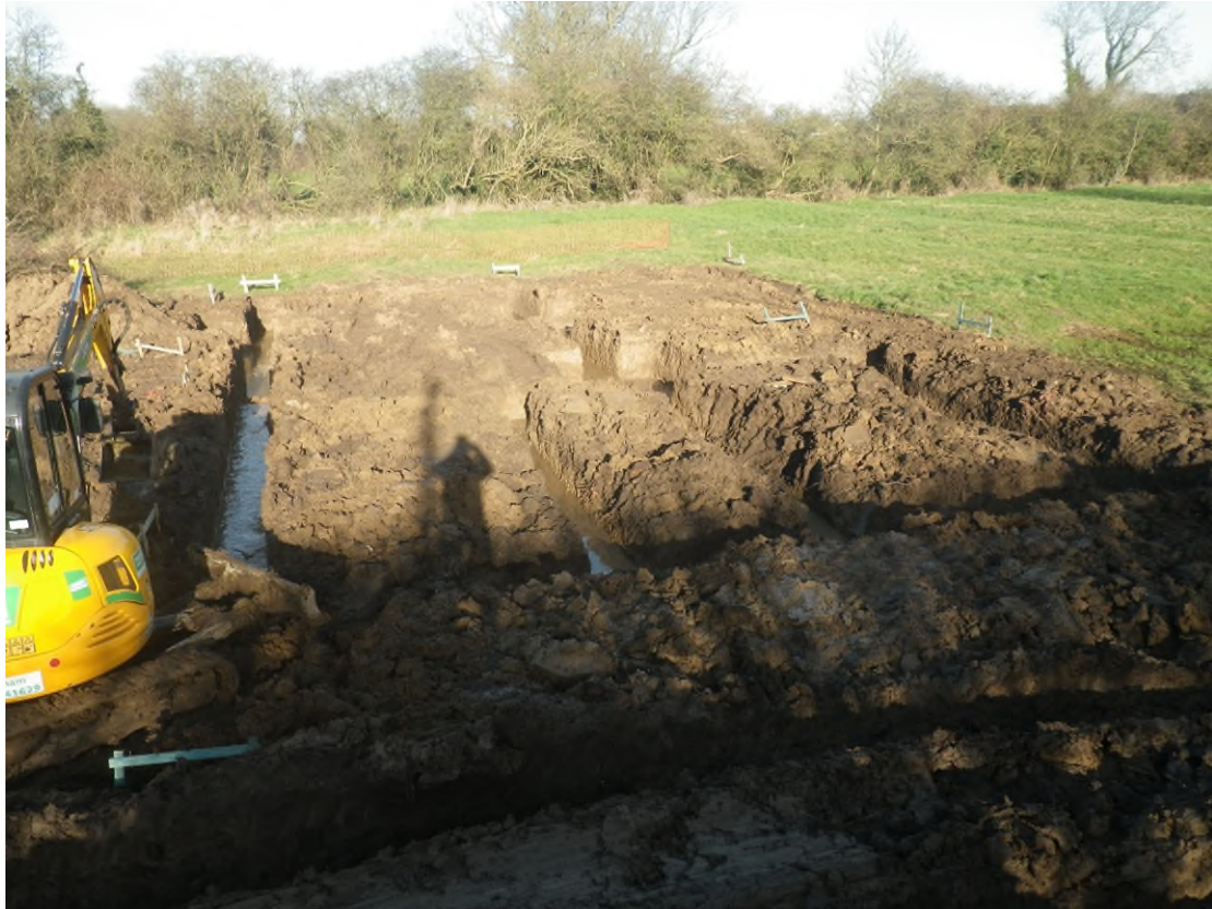
Plate 5 Plot 1 house foundations fully excavated, looking N
