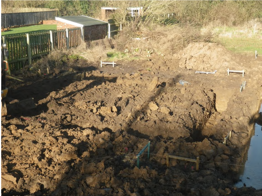
Plate 7 Plot 1 garage foundations fully excavated, looking NW
