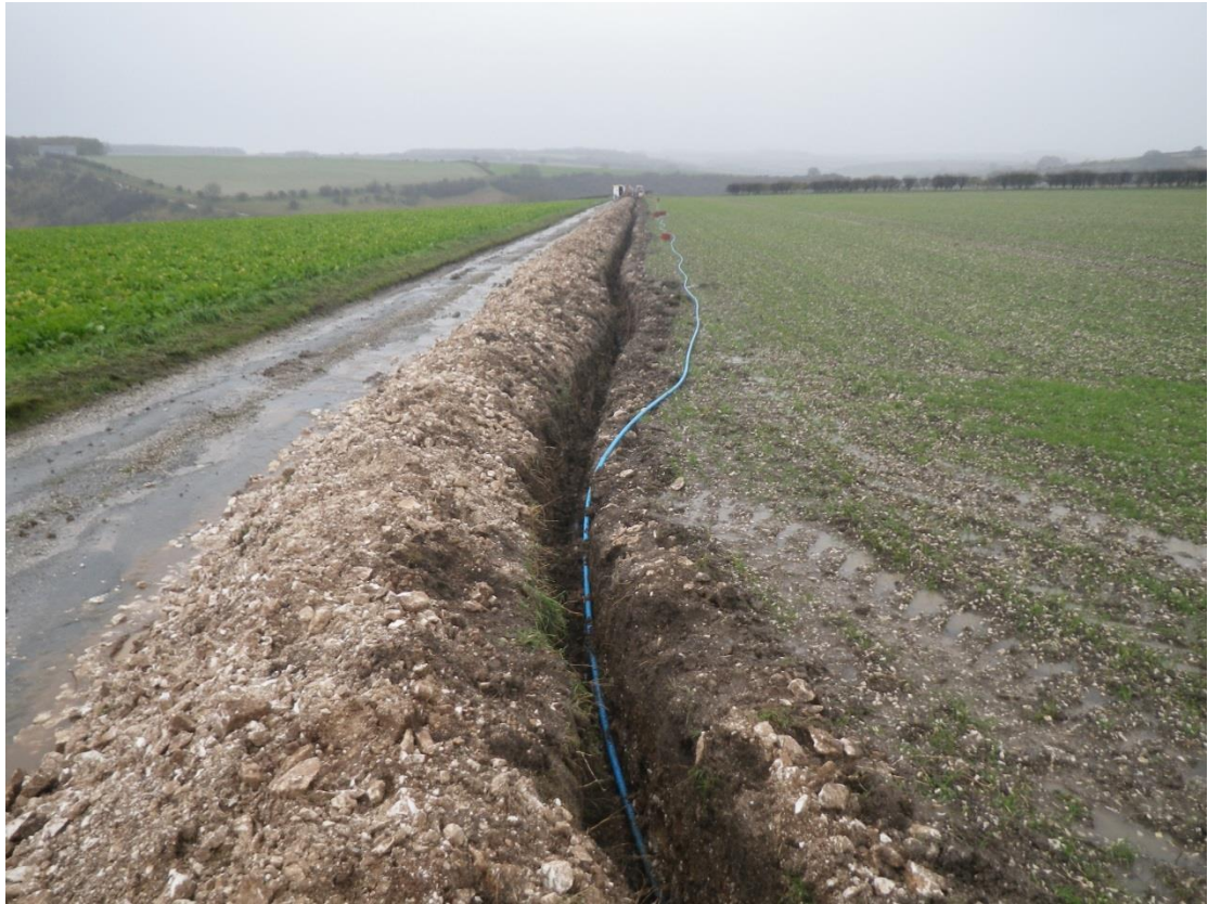
Plate 3 Trench running along the northern edge of field A, looking north-east
