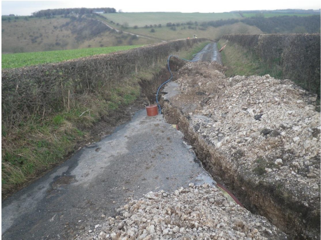
Plate 5 Trench crossing road between fields A and B, looking north-east
