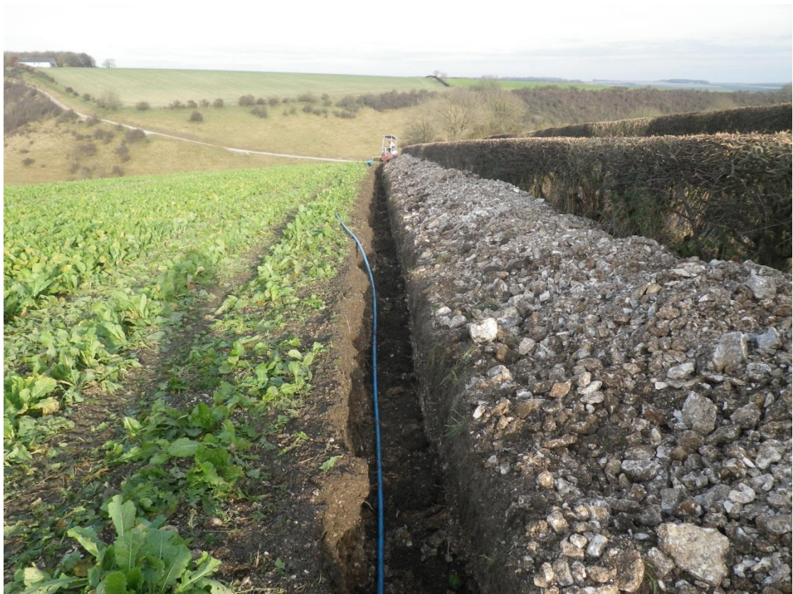
Plate 6 Trench running along the southern edge of field B, looking north-east
