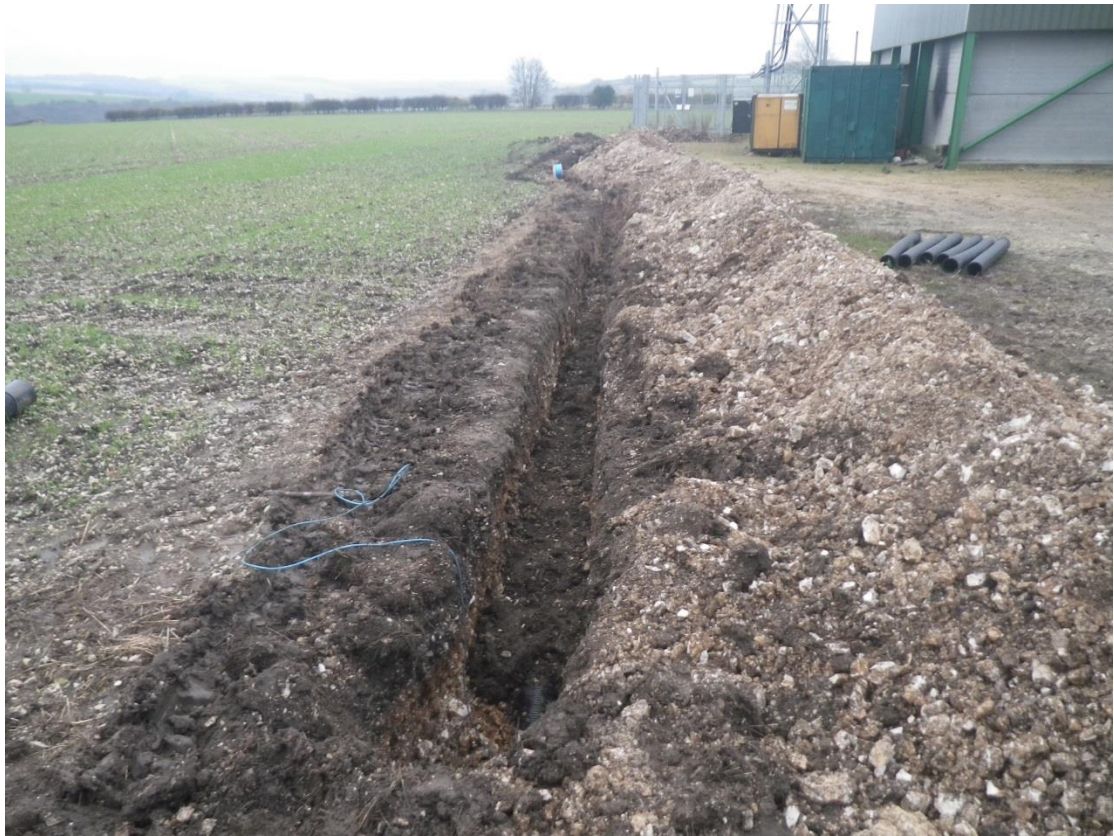
Plate 1 Cable trench to the west of the transmitter tower, looking east
