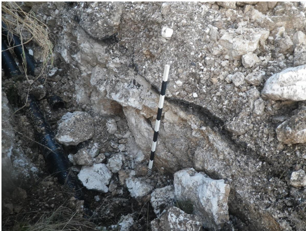
Plate 16 Chalk beneath road in trench immediately to the west of the junction with the trench excavated in field C
