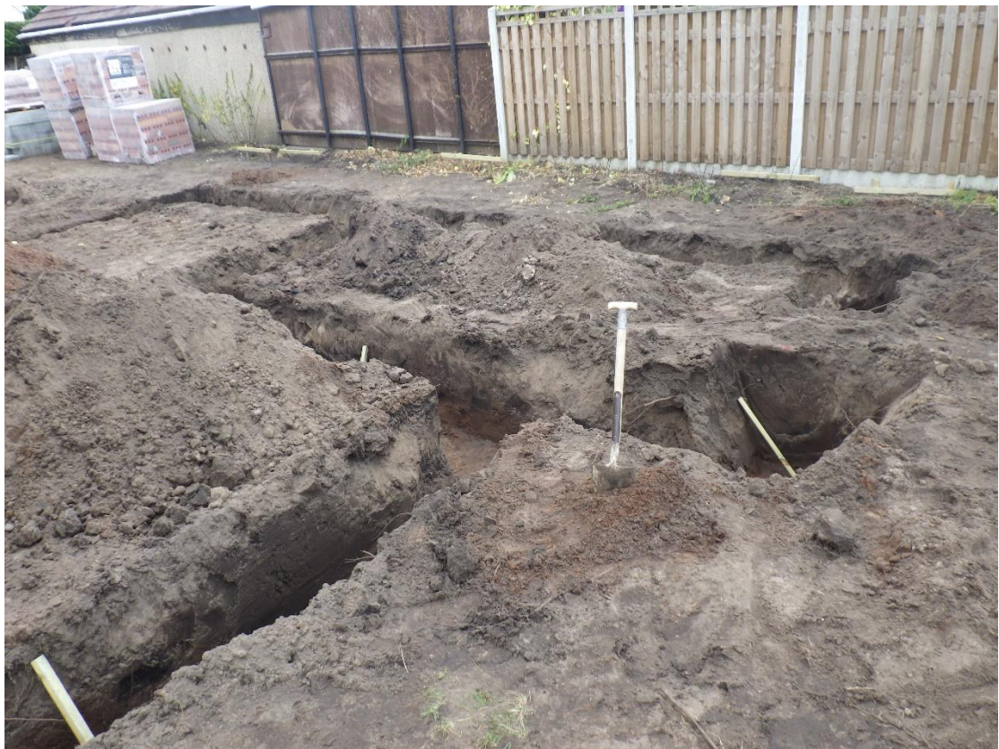
Plate 6 General view of the completed garage foundations, looking north-east.
