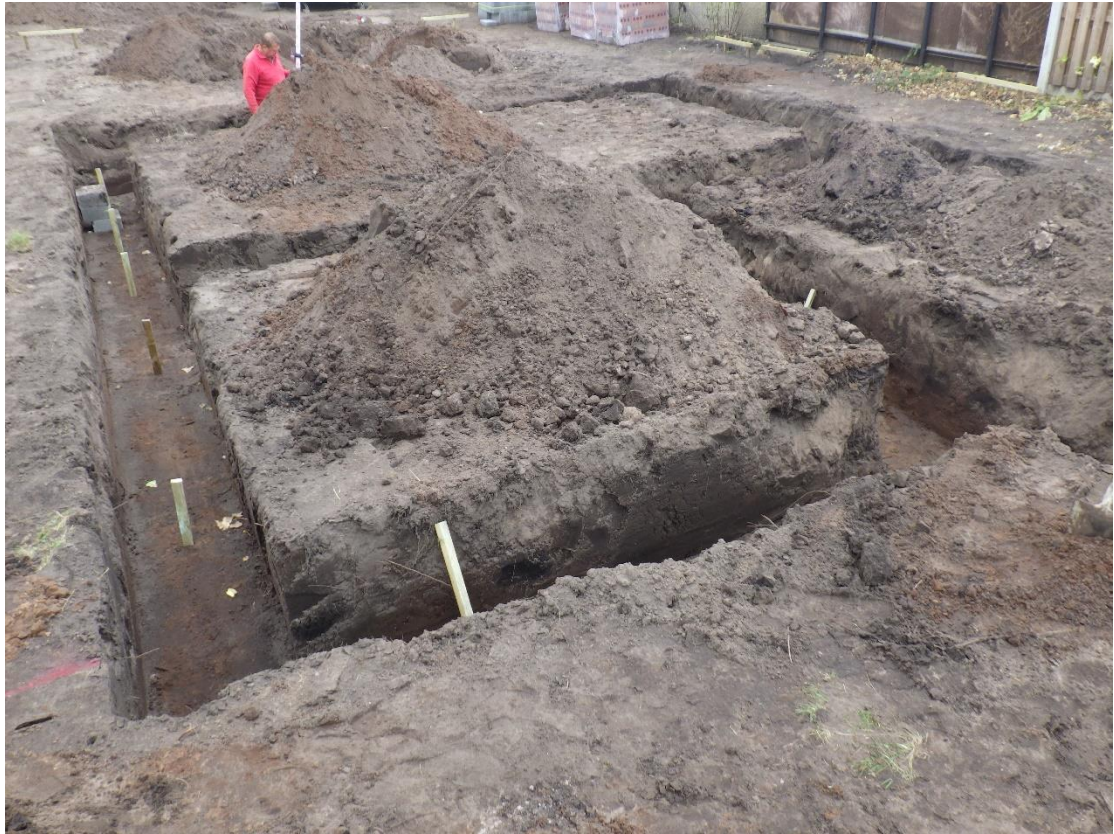
Plate 5 General view of the completed house foundations, looking north-east.
