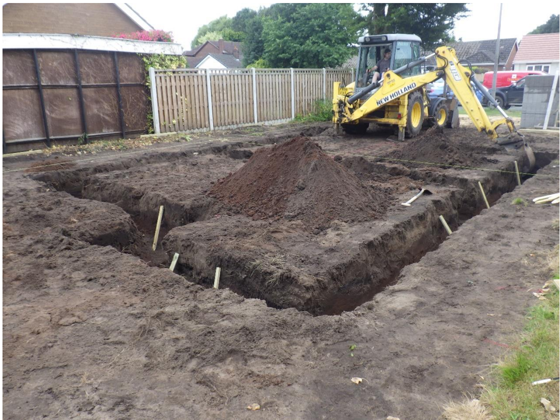
Plate 2 General view of excavations, looking south-east.
