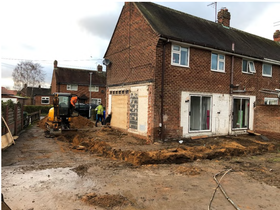
Plate 2 The completed foundation trench for the new extension
