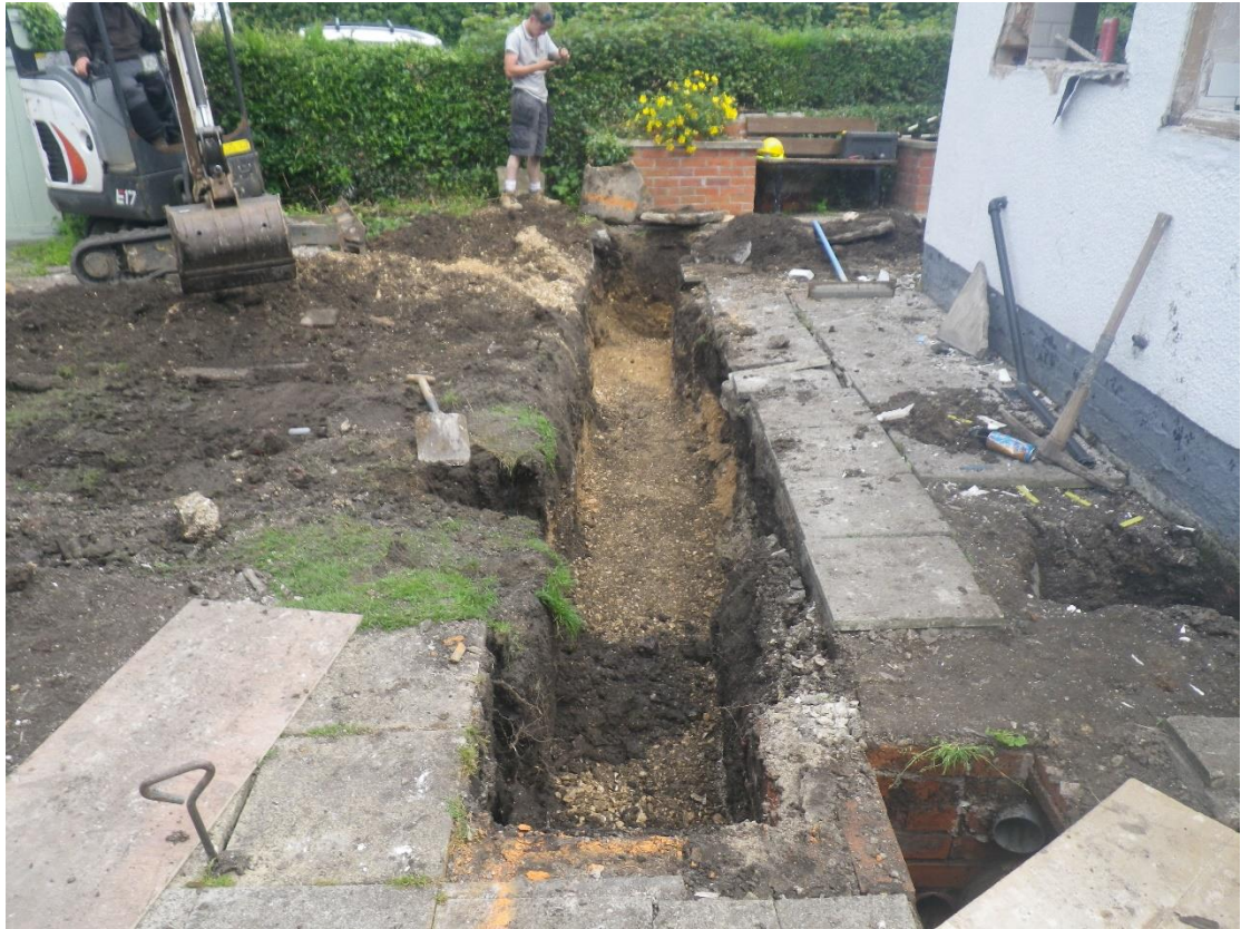
Plate 5 House extension footings, looking east
