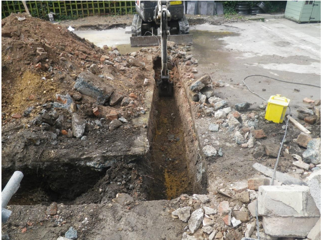
Plate 7 New garage footings, looking east
