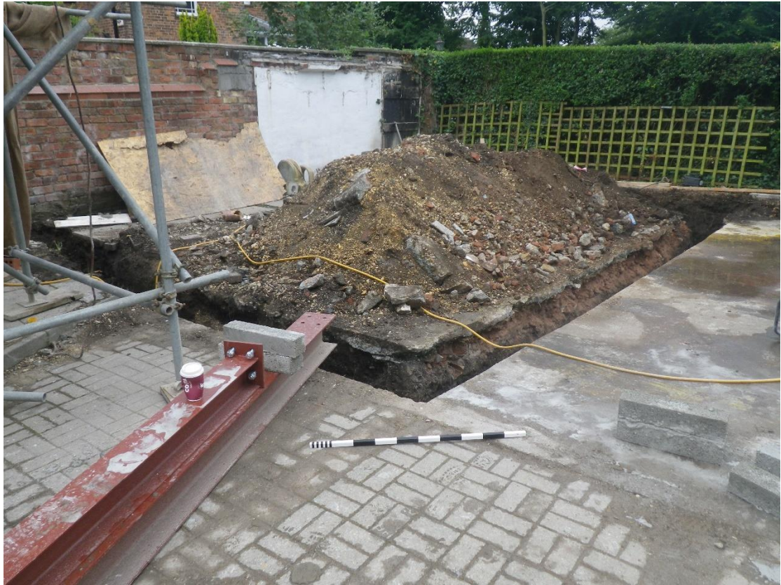
Plate 9 Overall shot of excavated new garage footings, looking east (1m scale)
