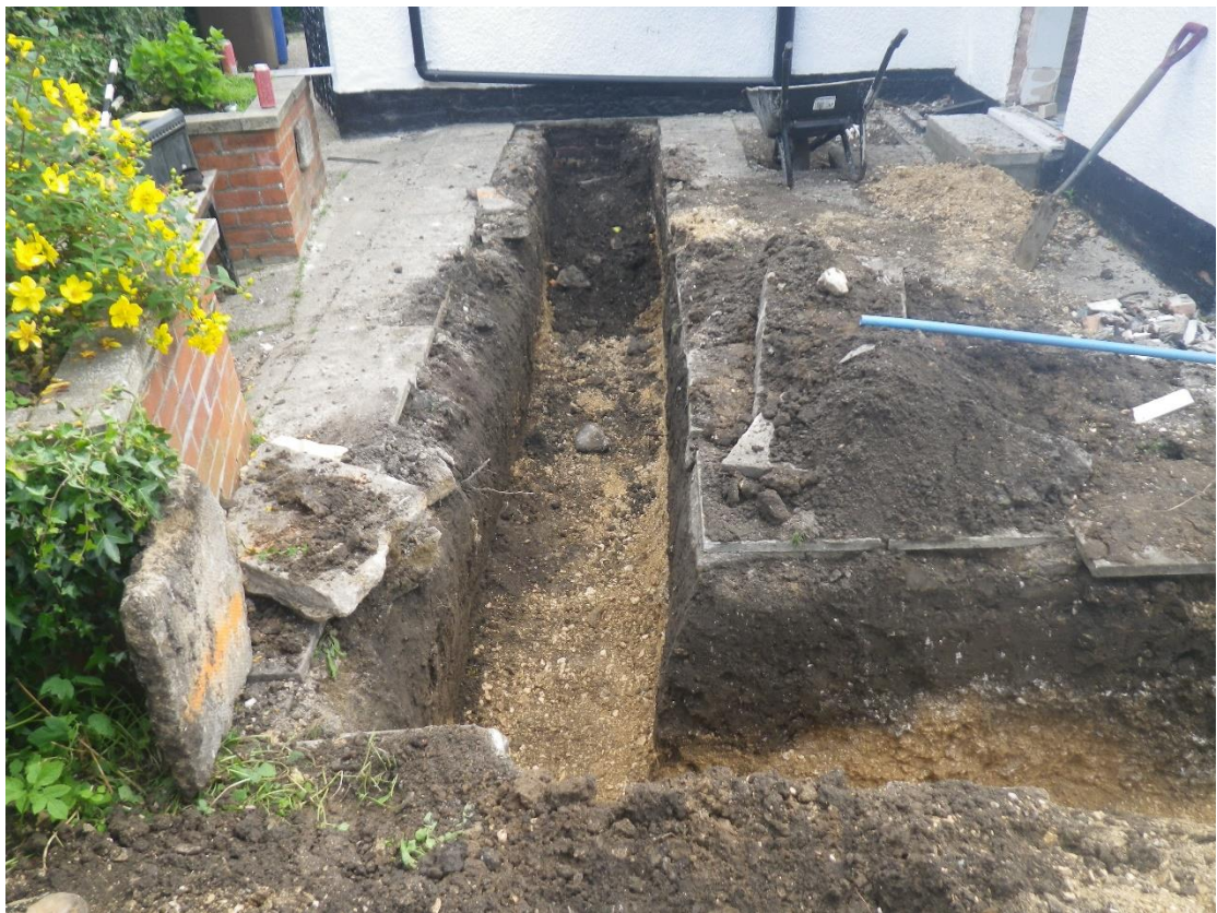
Plate 4 House extension footings, looking south
