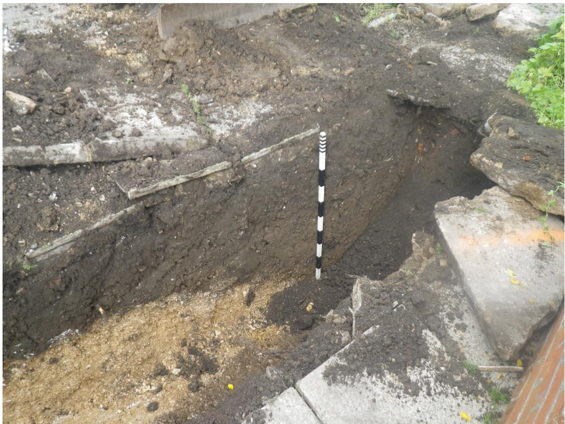
Plate 2 Ditch 1005, north west corner of house extension footings, looking north east (1m scale)
