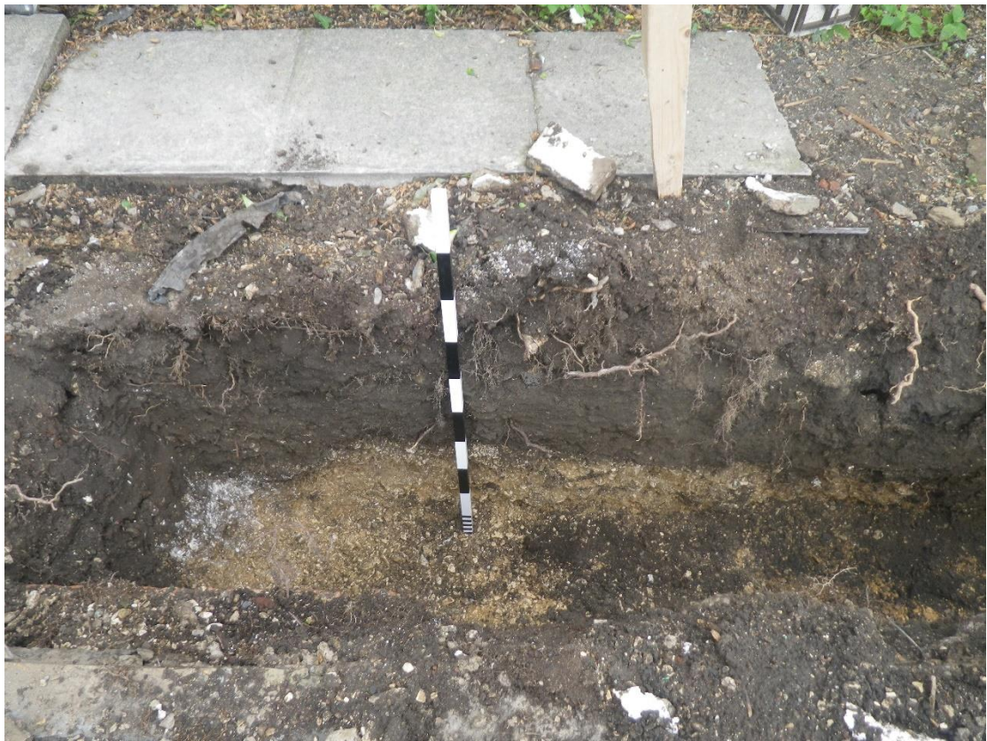
Plate 8 New garage footings with overlying soils (1m scale)
