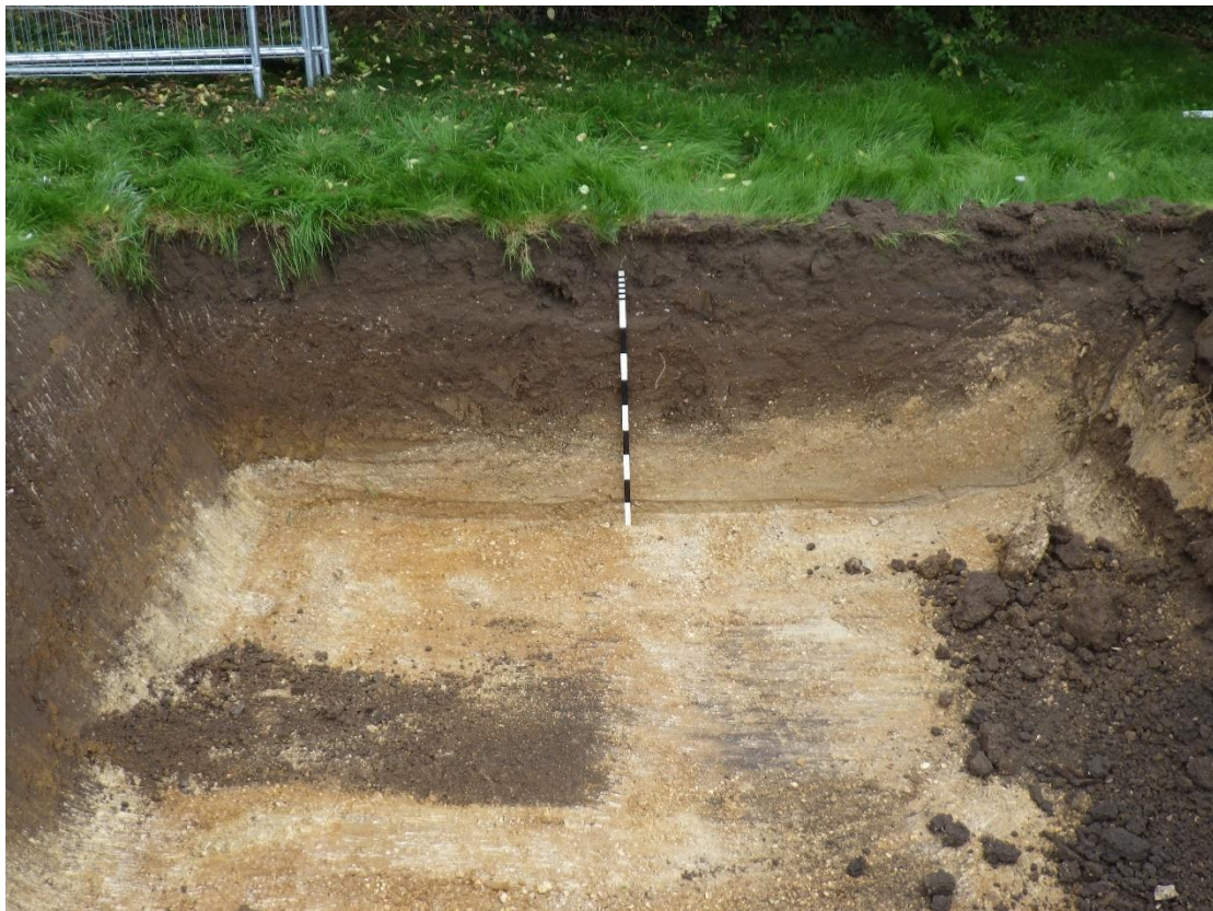
Plate 2 Representative section of materials within tank pit, looking north (1m scale).
