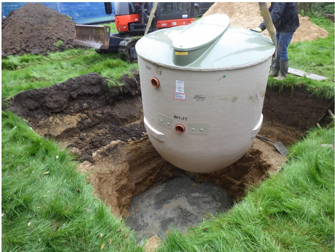
Plate 4 Soakaway tank being placed by machine, looking southGebner-east.
