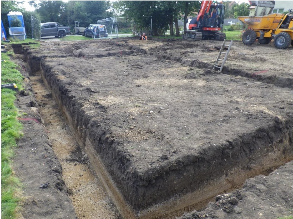
Plate 11 General view of the completed house foundation, looking south-west.
