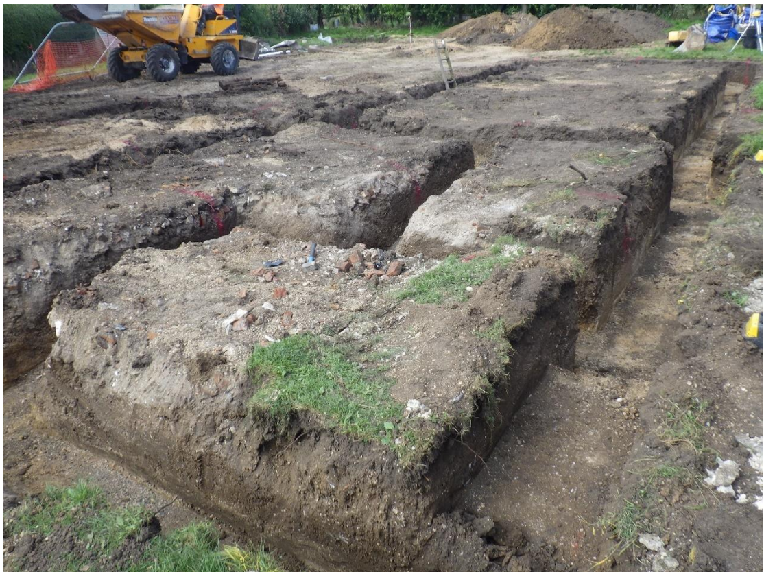
Plate 10 General view of the completed house foundation, looking north-west.
