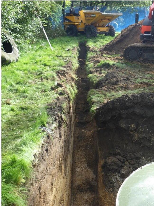
Plate 5 General view of soakaway pipe trench, looking east.
