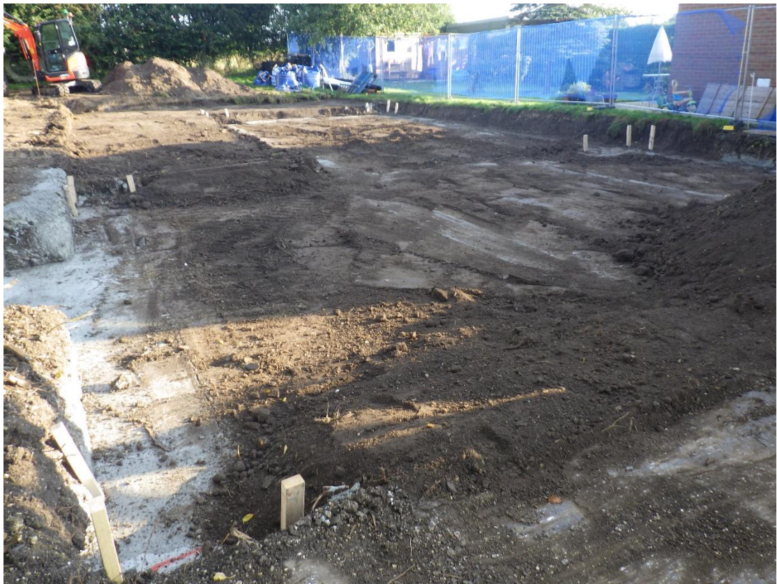
Plate 12 General view of concreted foundation and additional ground reduction, looking north-east.
