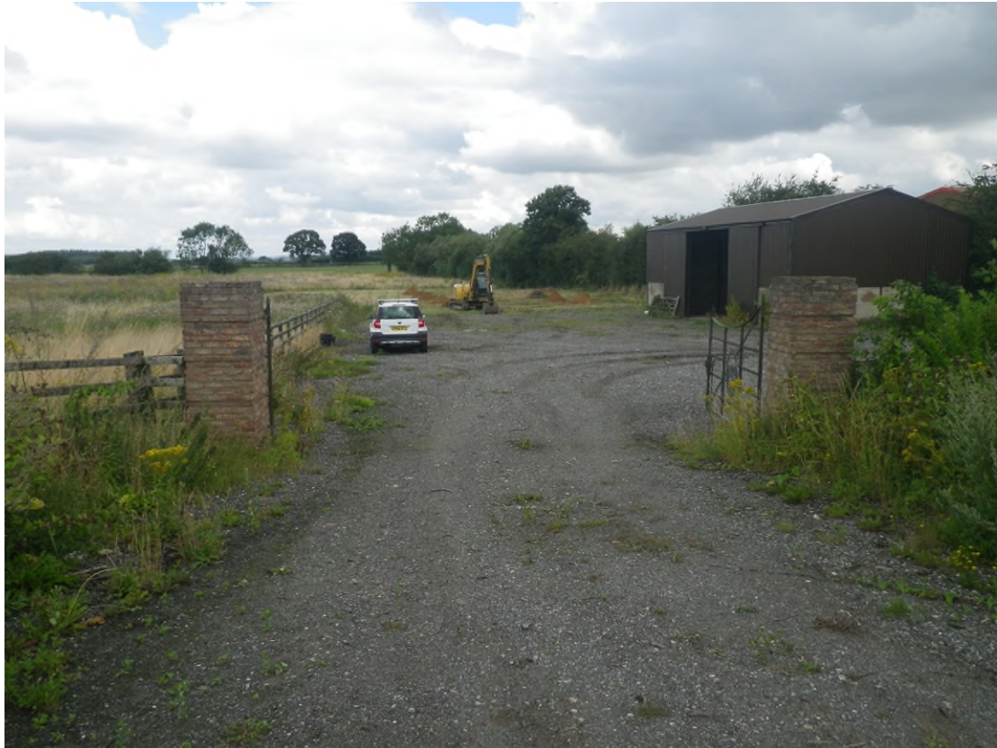
Plate 1 The development site, looking north
