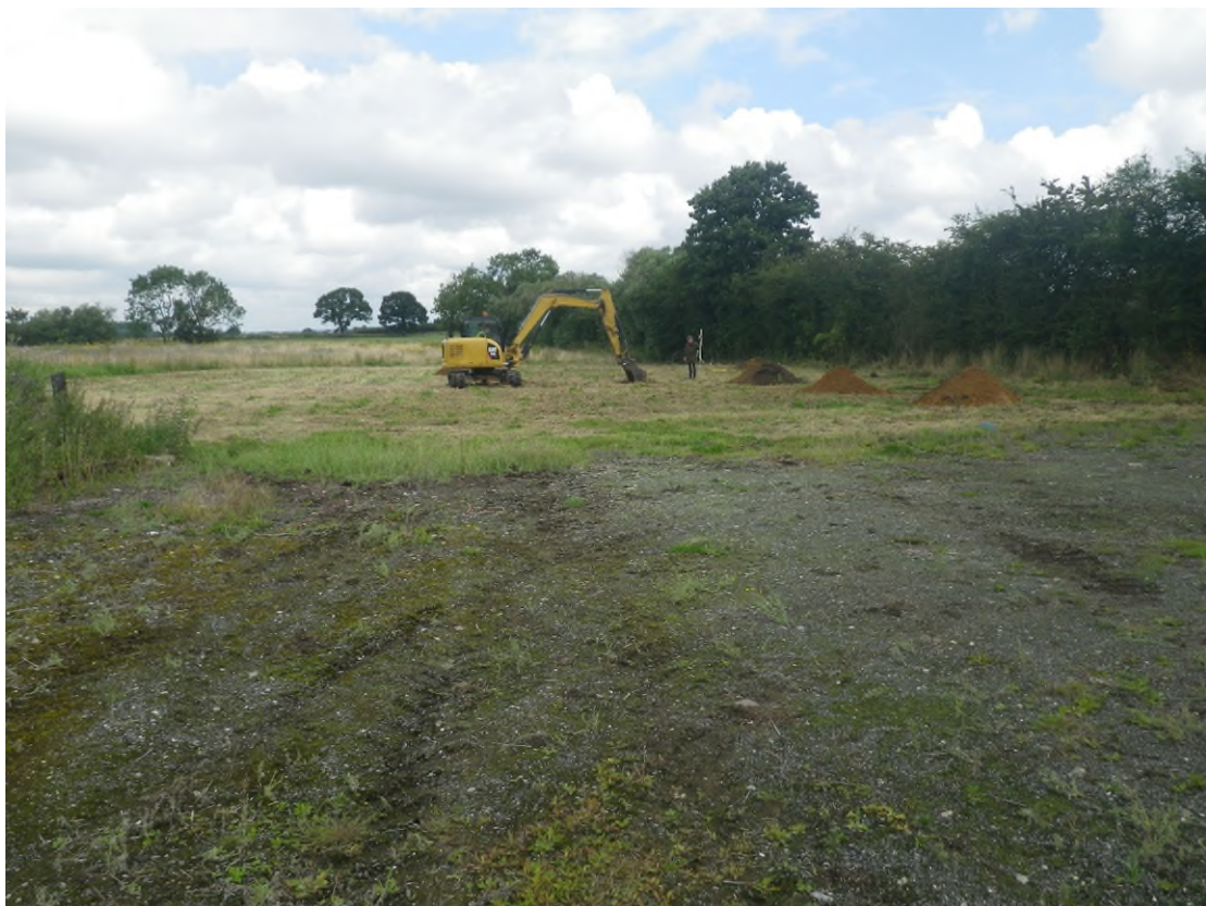
Plate 2 The excavation of the foundation pit in progress, looking north
