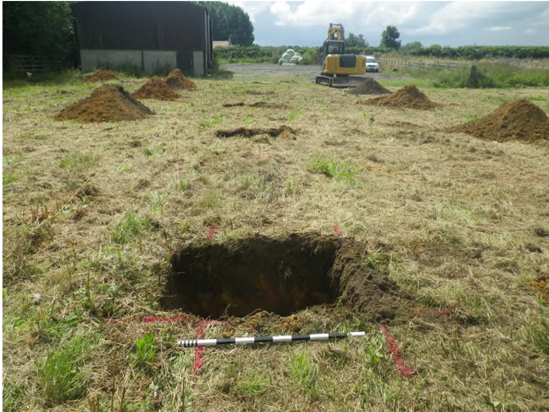
Plate 3 The western alignment of foundation pits, looking south
