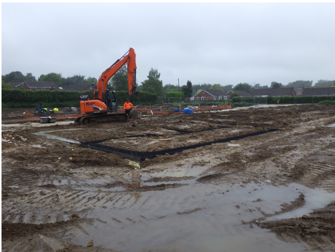
Plate 8 Overview of foundations dug into piling mat, looking north west.
