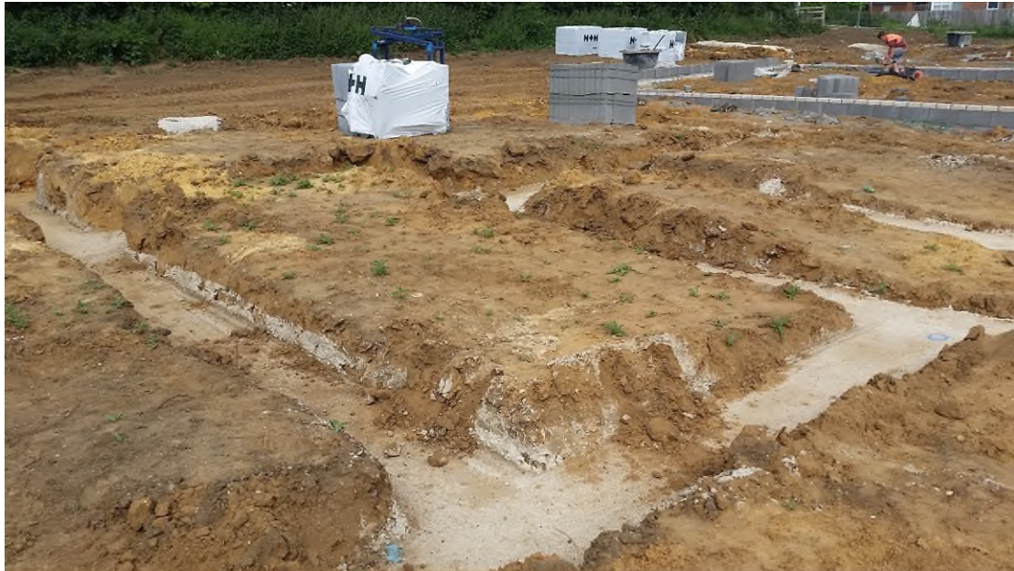
Plate 7 Excavated and concreted house foundation, looking north west.
