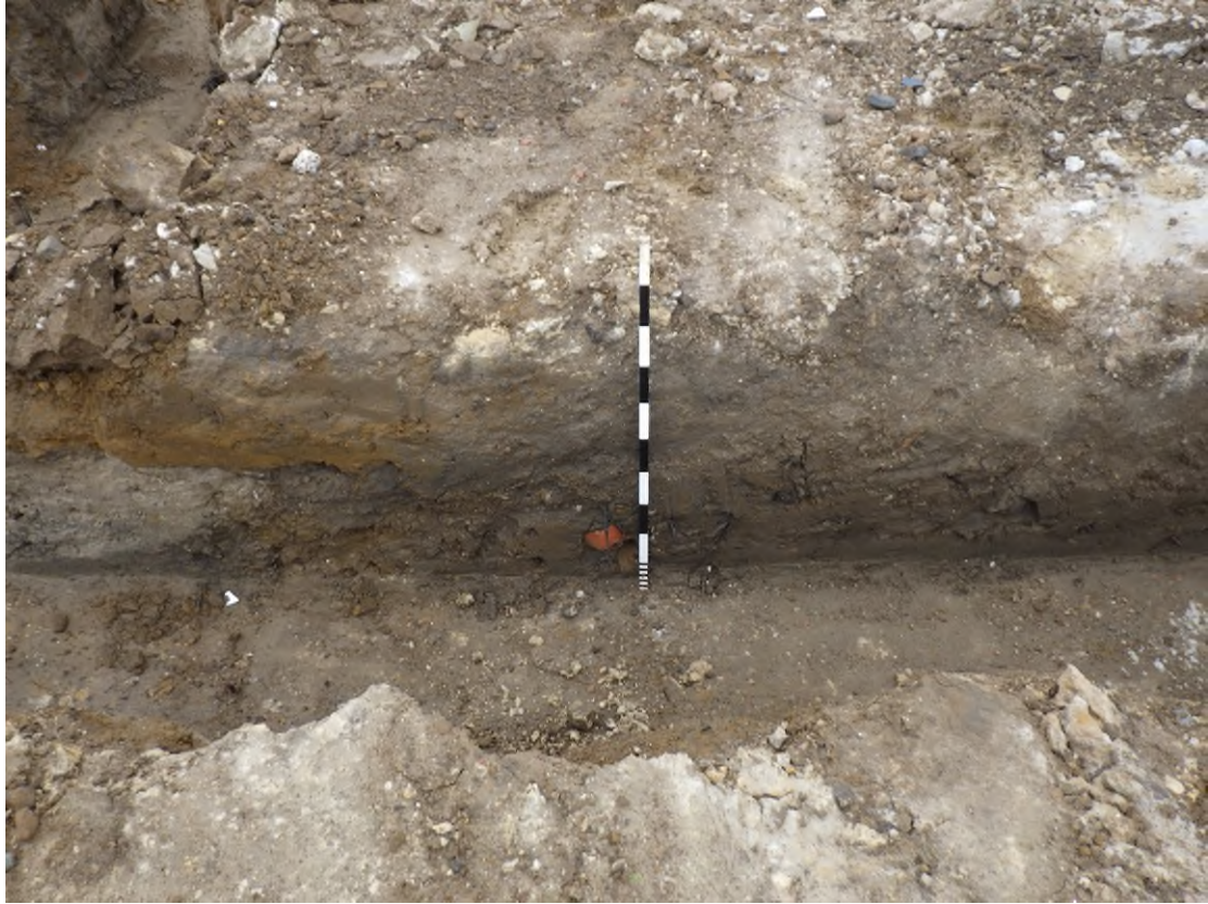
Plate 9 Representative section of piling mat material within house foundation, looking east (1.00m scale).
