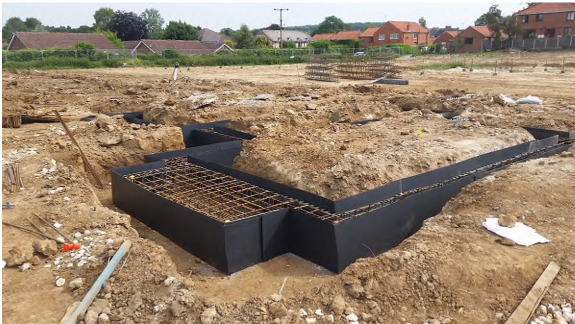
Plate 6 Excavated house foundation awaiting concrete, looking north east.
