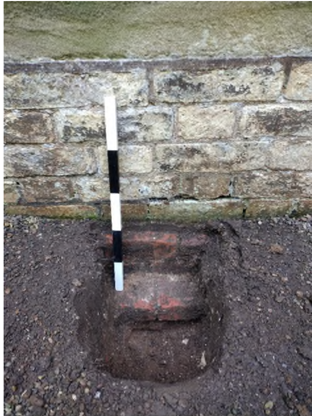
Plate 3 Intervention pit #2 on the western side of the north porch, showing a similar sequence of events as on the eastern side of the porch; post-medieval red brick stepped foundation 103, with the 1866 white brick north porch 101 sitting directly atop. Looking east, 0.5m scale.
