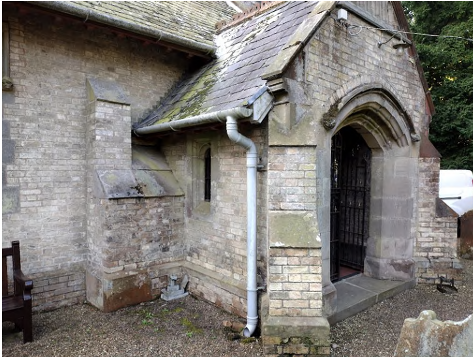
Plate 1 View of the north porch from the north-east.
