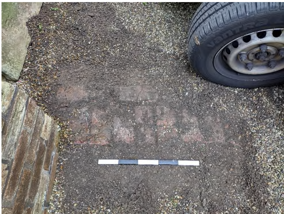
Plate 4 A further example of the likely post-medieval red brick foundation remains of the church demolished pre-1814 surviving at the current ground level. This example lies to the south-west of the north porch and north of the tower.
