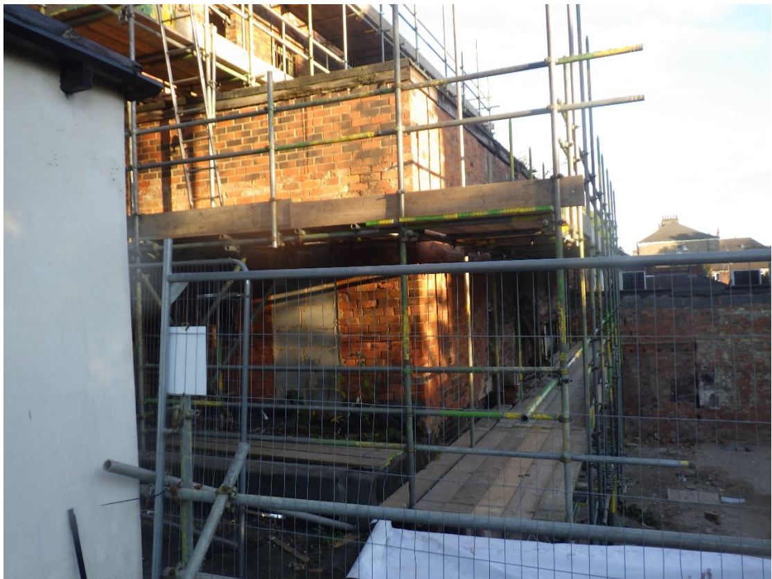
Plate 2 Oblique view of eastern elevation, looking north-west.
