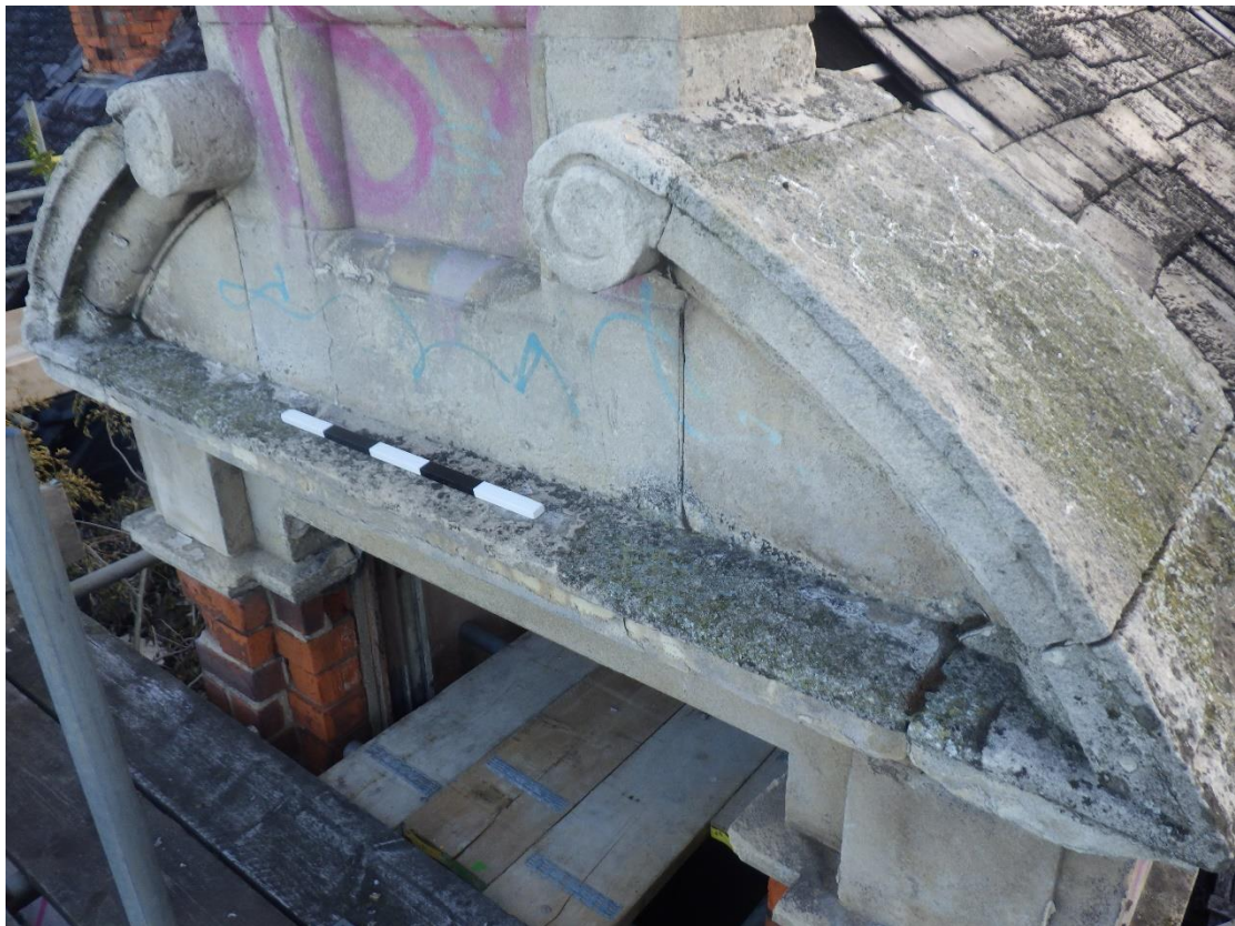
Plate 12 Overview of stone detail above dormer window, looking north-east (0.50m scale).
