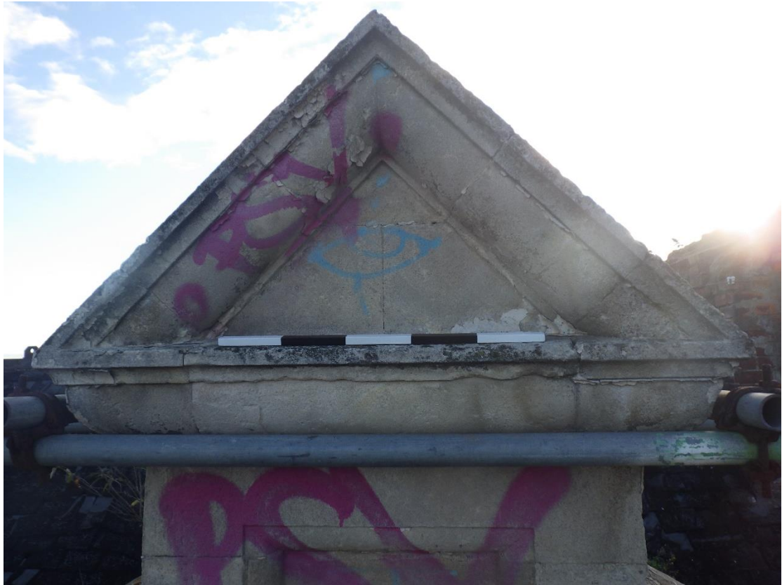
Plate 13 Decorative stone capping above dormer window, looking east (0.50m scale).
