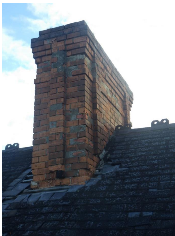
Plate 9 General shot of chimney stack showing outdented brick patterns, looking north-east
