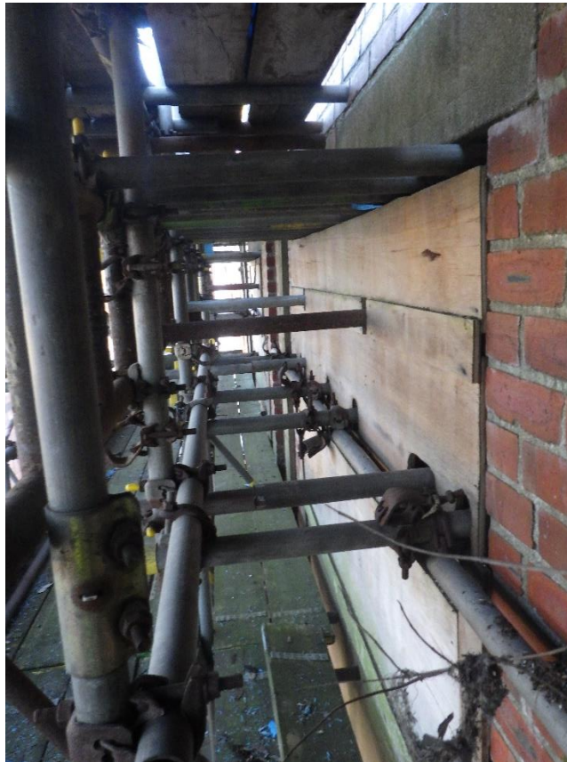
Plate 16 General view of boarded up windows on second storey, looking north.
