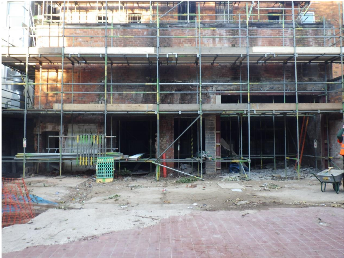
Plate 1 General view of eastern elevation, looking west.
