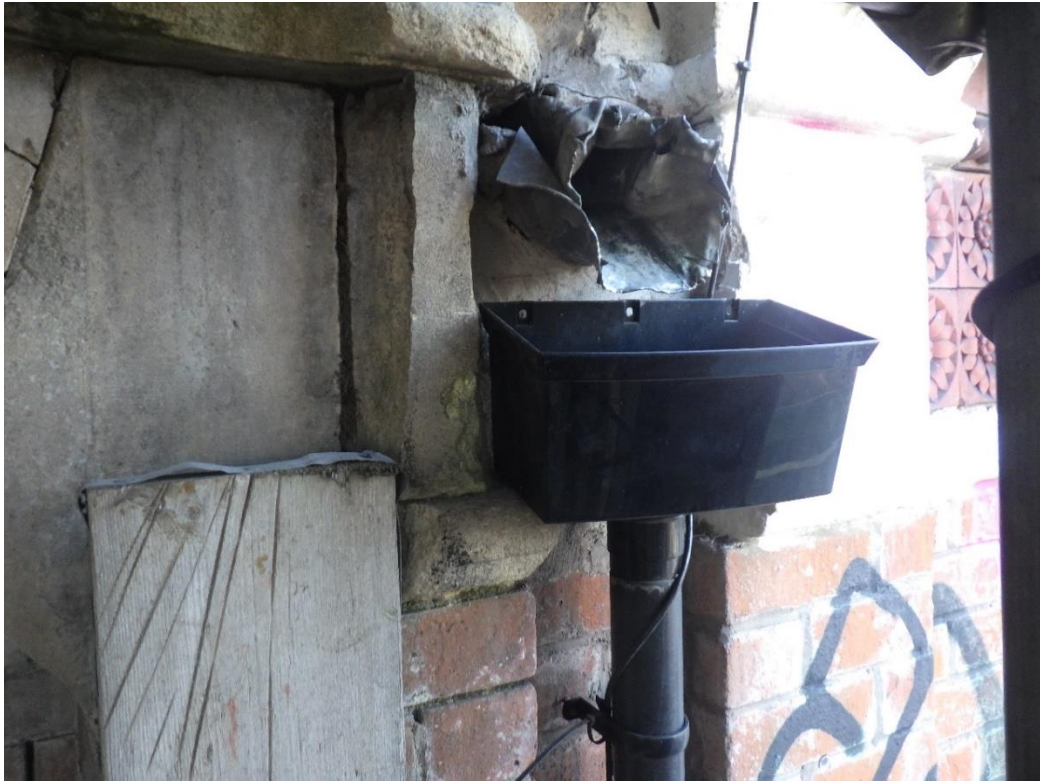
Plate 17 In-situ drainpipe feeding into modern replacement fall pipe, looking south-east.
