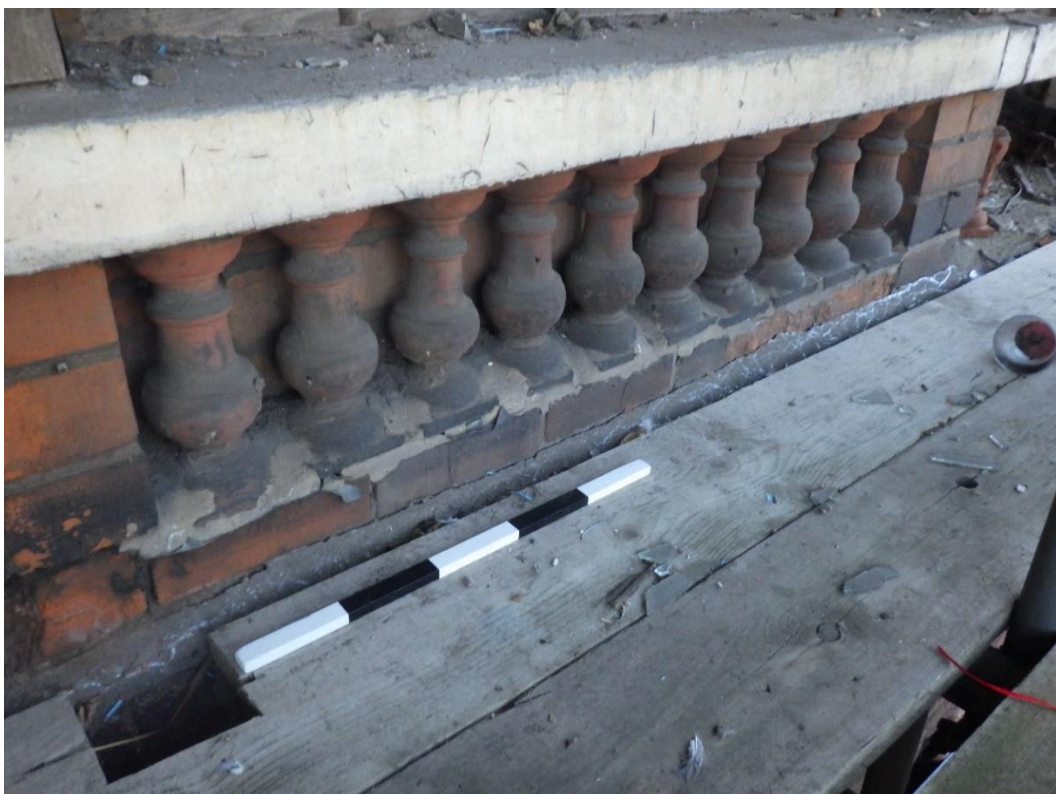
Plate 20 Detail shot of decorative columns underneath sill of bay window on first storey, looking south-east (0.50m scale).
