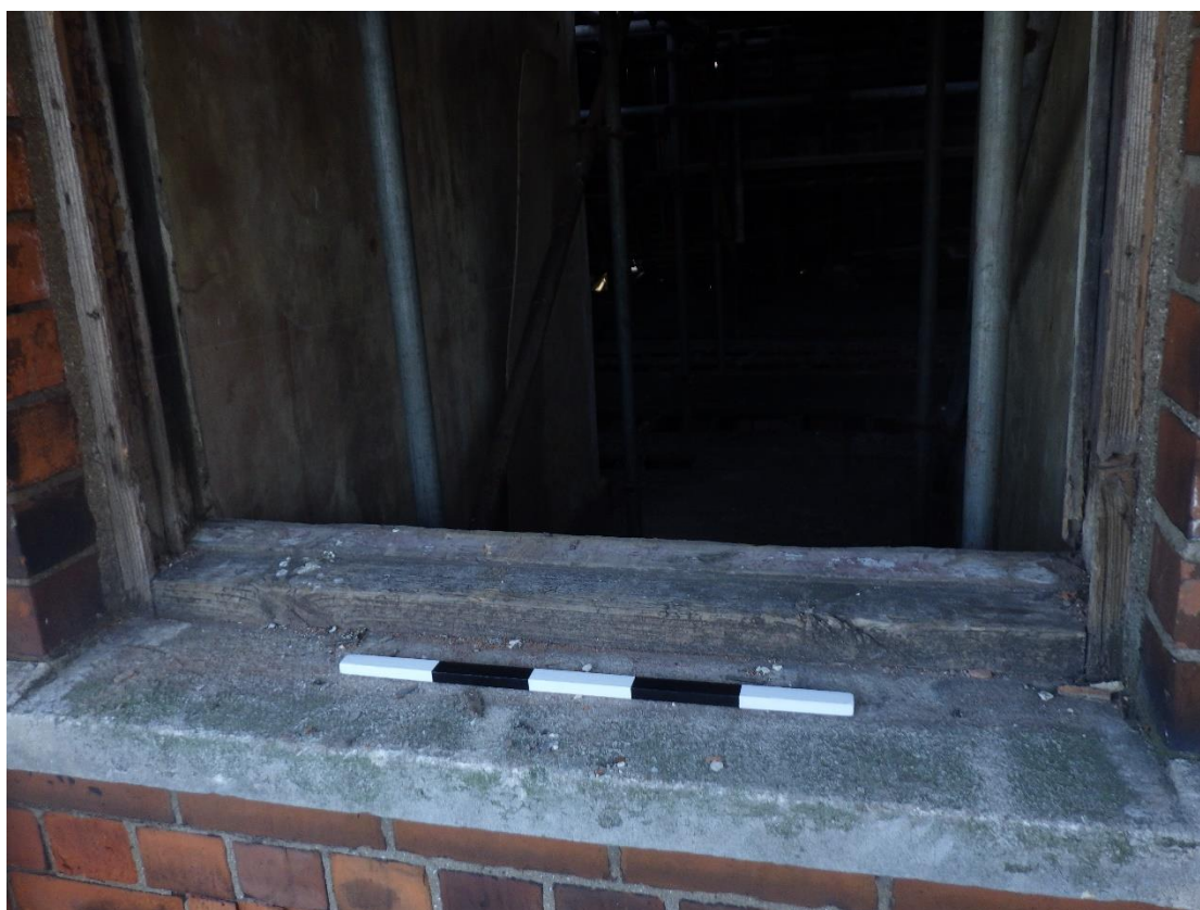
Plate 10 Detail shot of sill of dormer window, looking east (0.50m scale).
