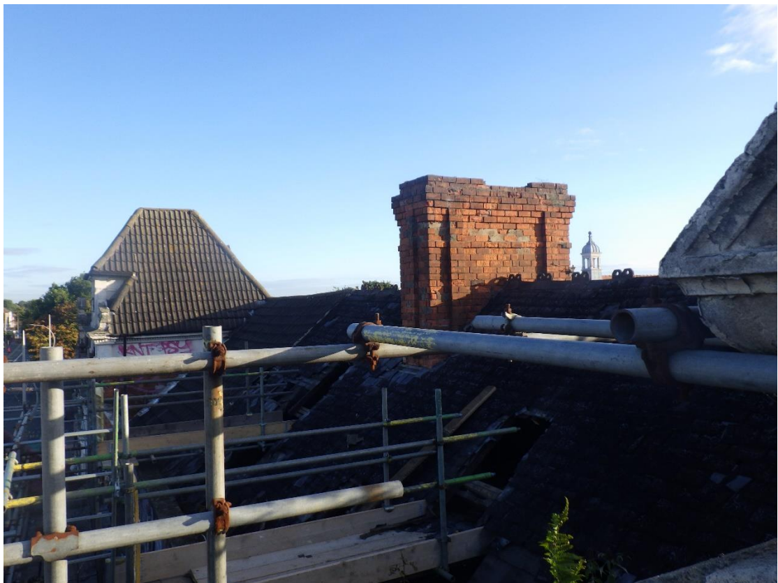
Plate 14 General view over rooftop of Brunswick Arcade, looking north-east.
