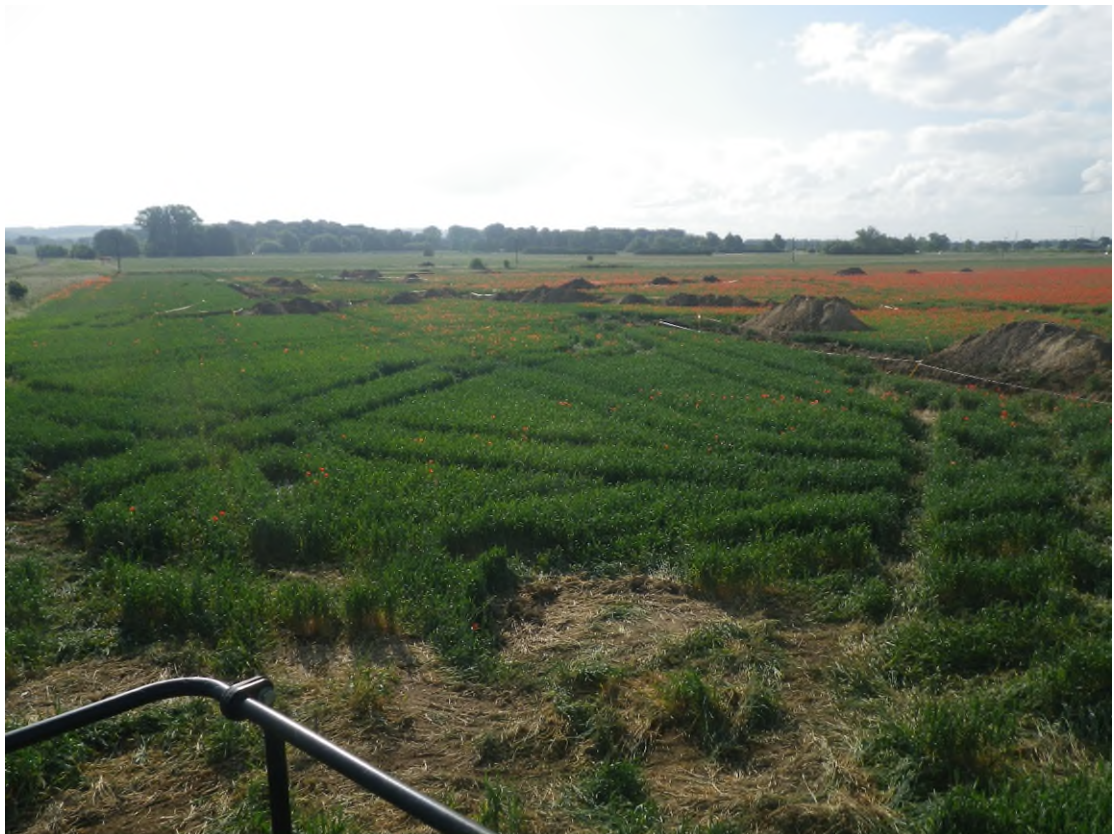
Plate 2 - Elevated view of open trenches looking east
