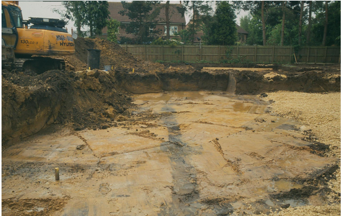
Plate 9 Land drain (504), looking south-southeast.
