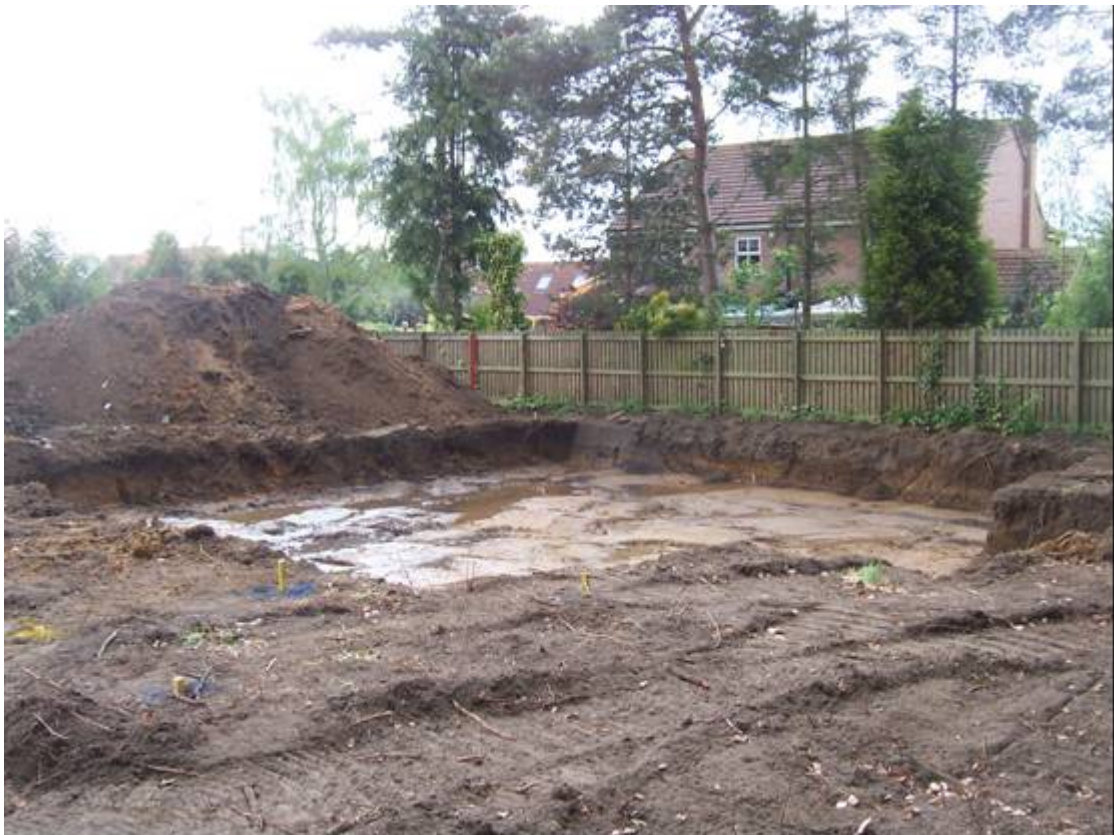
Plate 4 Plot 4, viewed from the northwest.
