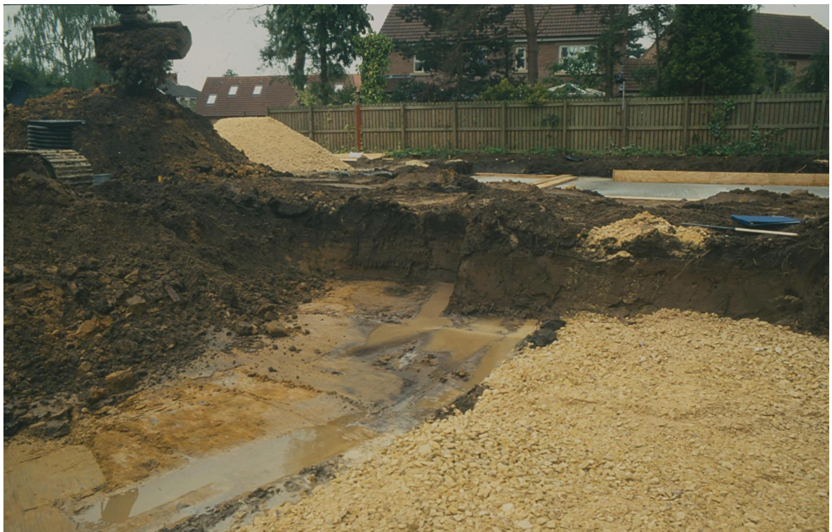
Plate 8 Ditch (507) in Plot 5, looking south.
