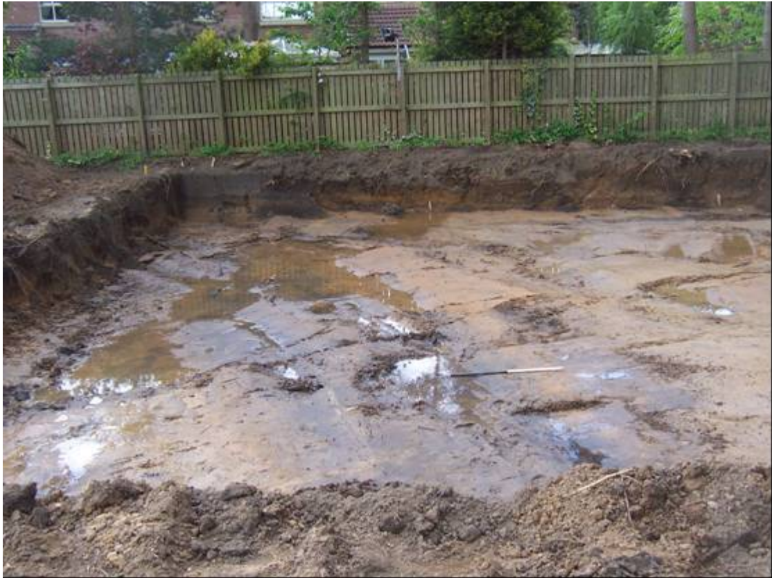
Plate 5 Former boundary ditch (409), viewed from the north. 1.00m scale.
