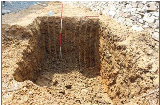
Plate 4. Excavation for attenuation tank, looking South, Scales: 2m and 1m.
