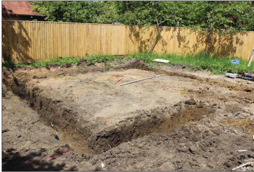
Plate 1. Completed excavation of footing, looking North West, Scales: 1m x2.
