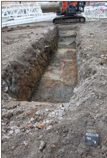
Plate 8. Trench 4 looking south west. Scales: 2m, 1m and 0.3m.
