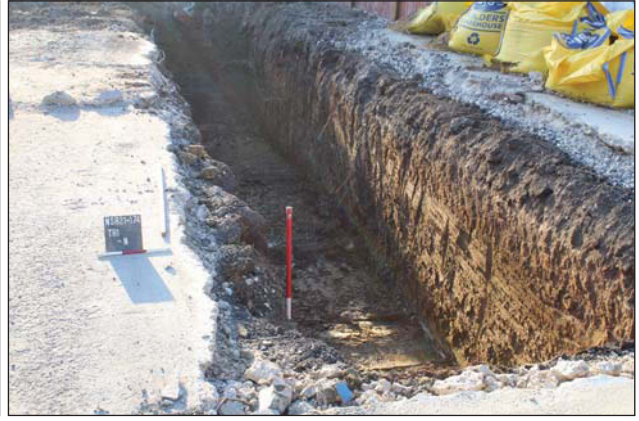
Plate 2. Trench 1 looking south west. Scale: 2m.
