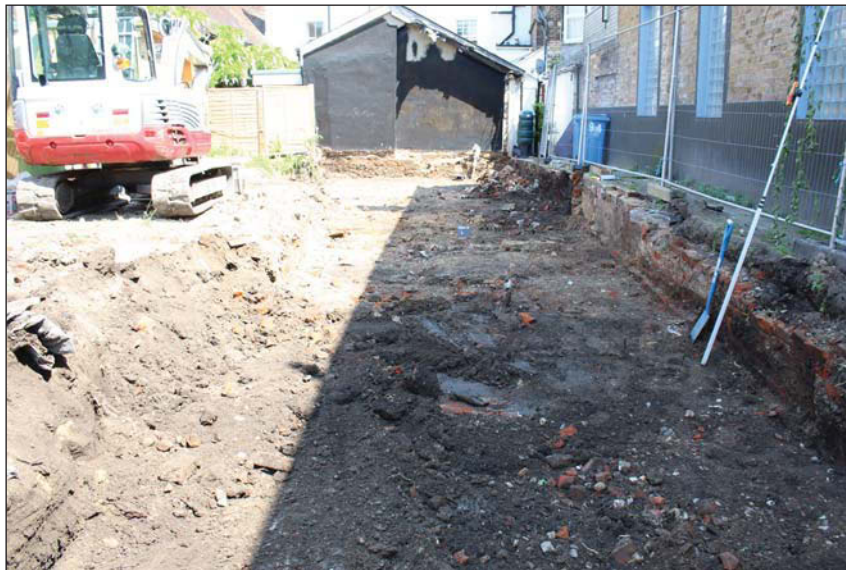
Plate 2. Eastward facing base of excavation, Scales: 0.3m.
