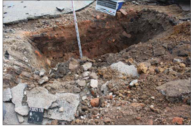
Plate 2: TP 1 showing brick viaduct foundations looking North. Depth of scale: 1.1m
