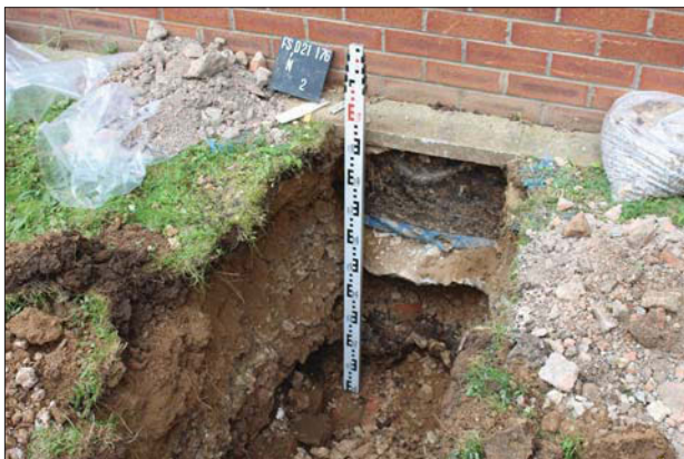
Plate 5: TP 2 looking South. Depth of scale: 1m
