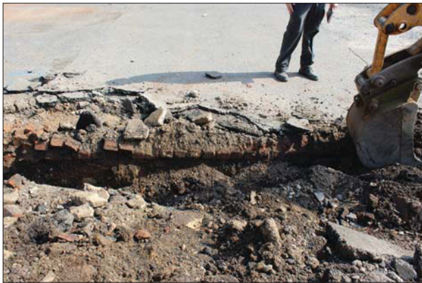
Plate 3: TP 1 extended to east to reveal more of brick foundations, looking North
