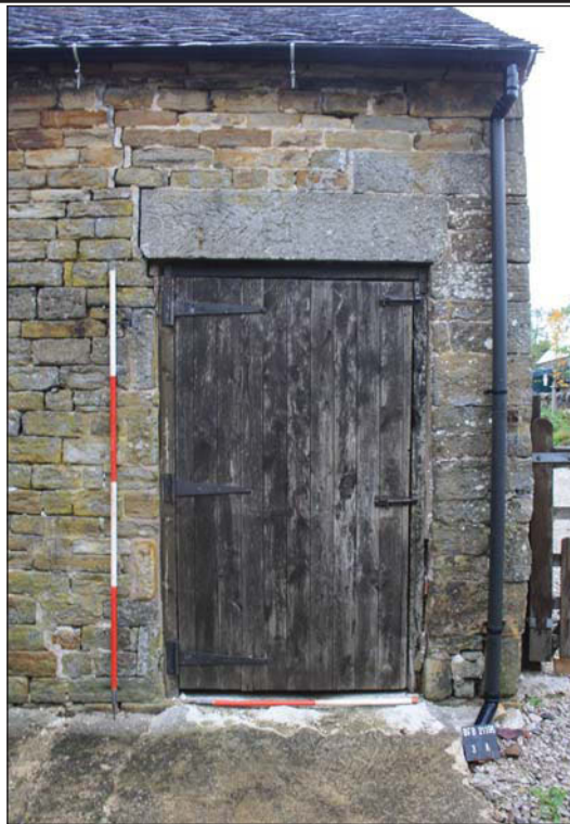
Plate 31. The two-metre high stable door in the southern elevation, looking north, Scales: 2m and 1m.
