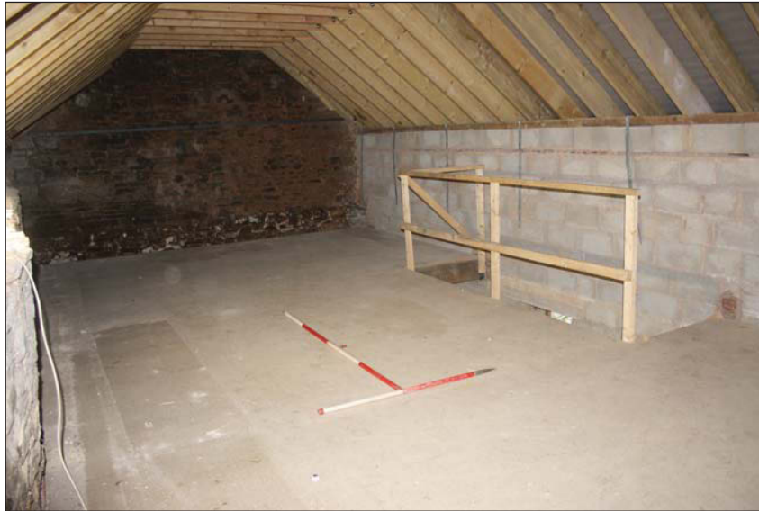
Plate 23. First floor, looking south, scales 2m and 1m.
