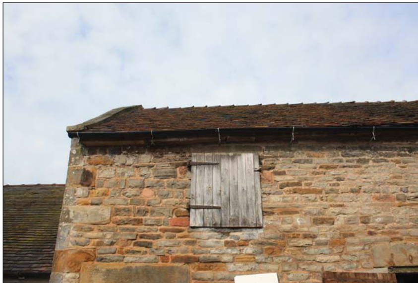
Plate 14. Detail of first floor window hatch on the front elevation of cow-house, looking west.
