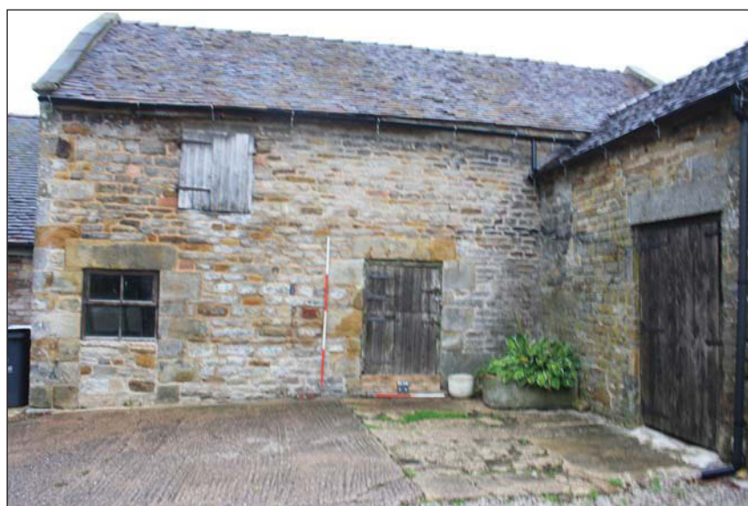
Plate 2. Eastern elevation of cowhouse showing how the structure is built onto the slope, looking west, Scales: 2m and 1m.
