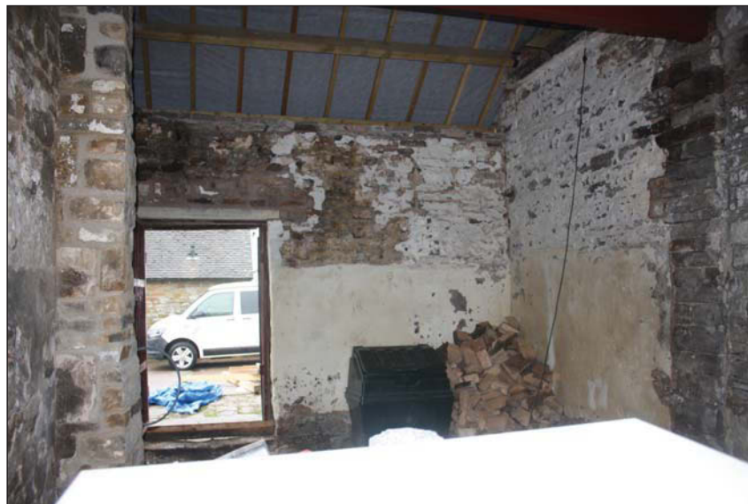
Plate 41. View to stable showing lime wash, looking south.
