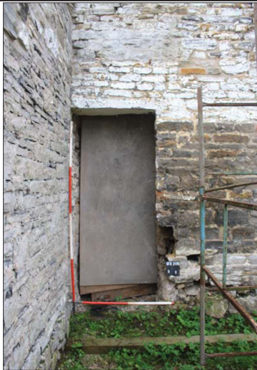
Plate 5. Additional later opening to north elevation of cow-house, looking south, Scales: 2m and 1m.
