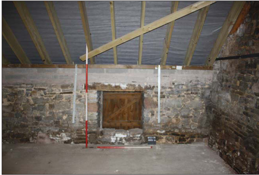
Plate 25. First floor pitching eye, looking east, scales 2m and 1m.
