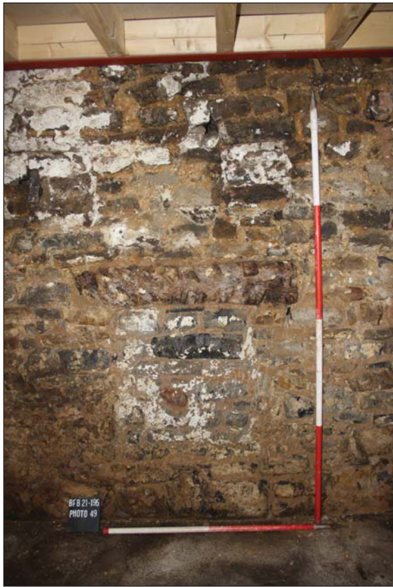
Plate 21. Blocked window, looking south, scales 2m and 1m
