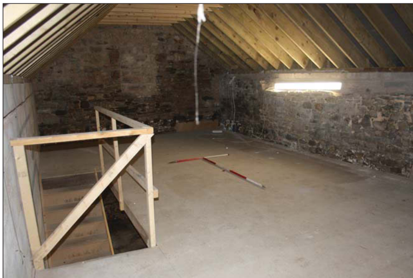
Plate 24. First floor, looking north, scales 2m and 1m.
