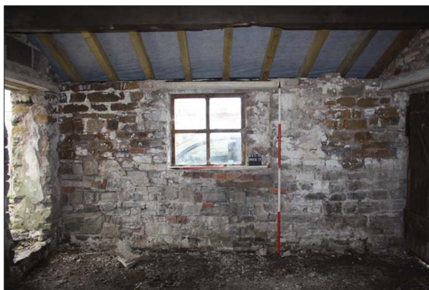
Plate 42. View to lean-to extension, looking north, Scales: 2m and 1m.
