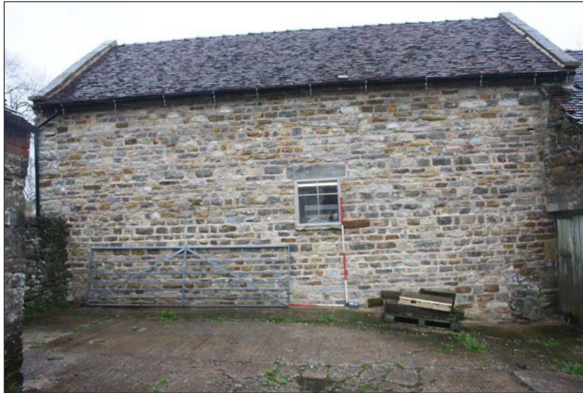
Plate 11. West elevation of cow-house showing slope and neighbouring farmyard, looking east.
