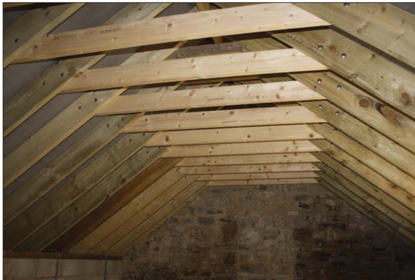
Plate 28. Roof detail, looking north.
