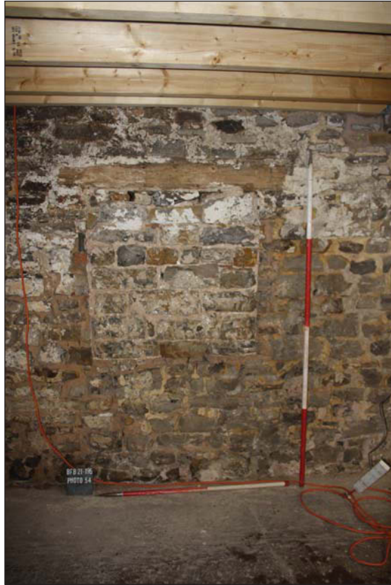
Plate 19. Blocked window / door, looking east, scales 2m and 1m.
