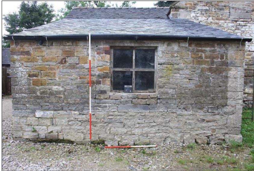
Plate 35. North elevation of lean-to extension, looking south, Scales: 2m and 1m
