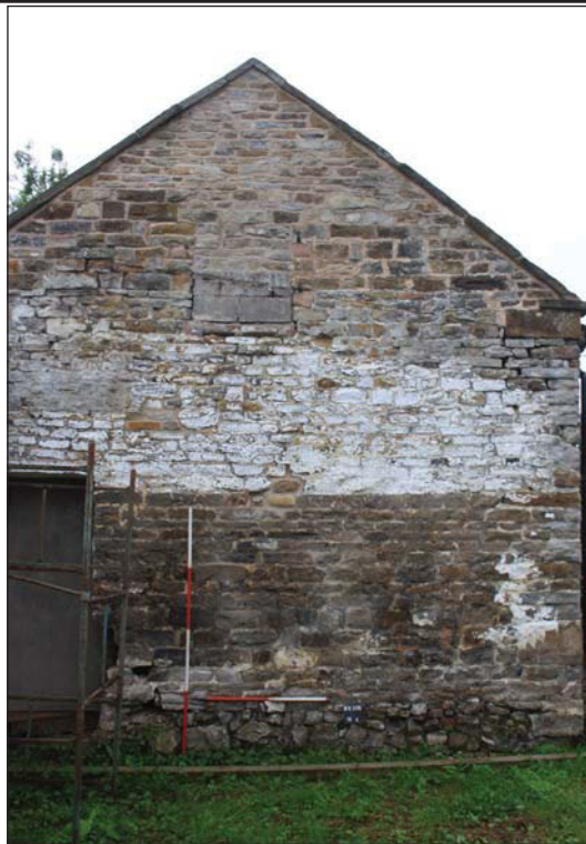
Plate 7. Northern elevation showing cow-house gable, looking south, Scales: 2m and 1m.
