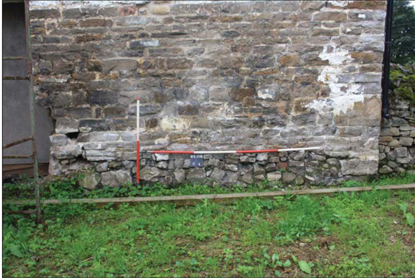
Plate 9. Rubble course walling visible at base of north gable of cow-house, looking south, Scales: 2m and 1m
