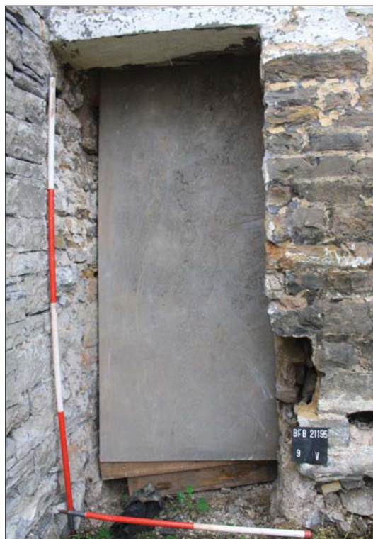
Plate 6. Detail of later doorway cut into northern cow-house wall, looking south, Scales: 2m and 1m.
