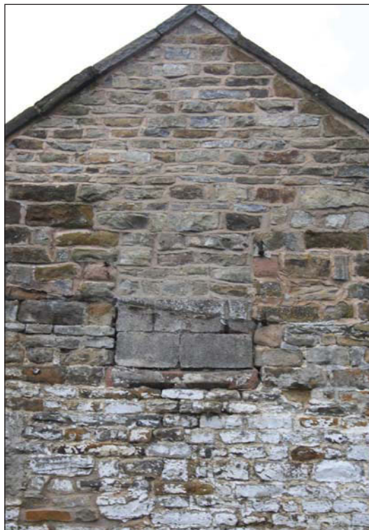
Plate 8. Detail of blocked hayloft opening in north gable of cow- house, looking south,
