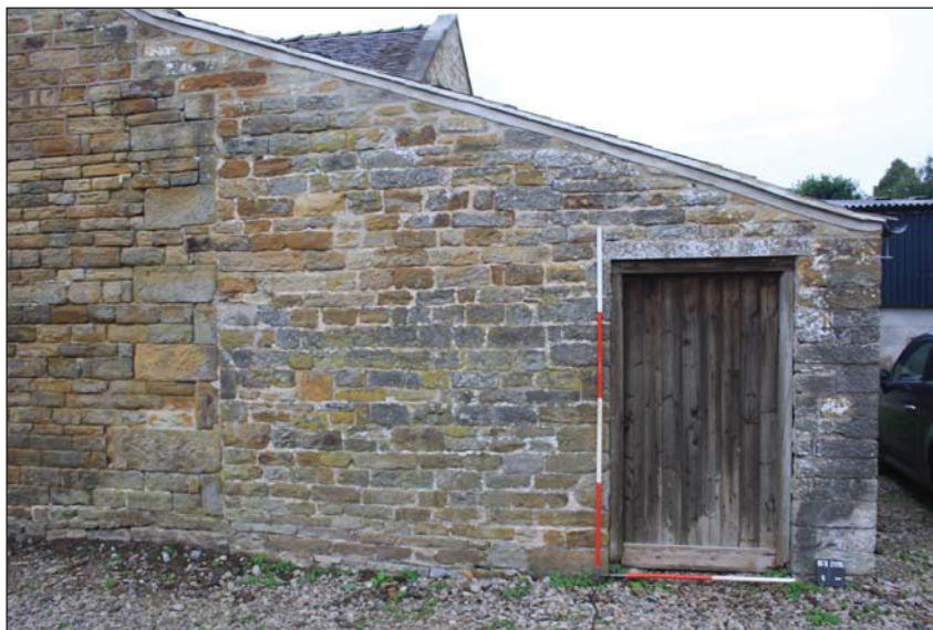
Plate 34. Lean-to door showing evidence of extension to stable, looking west, Scales: 2m and 1m.
