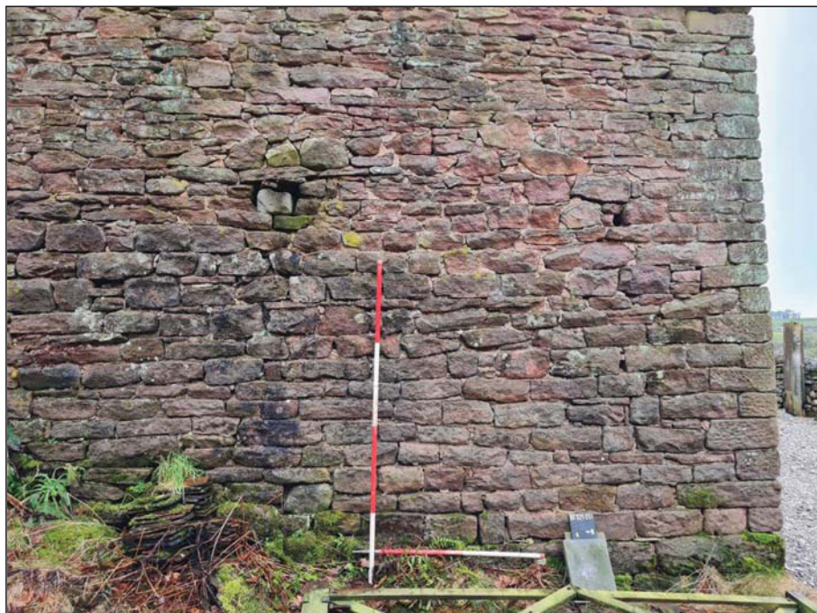
Plate 8. East elevation detail.
