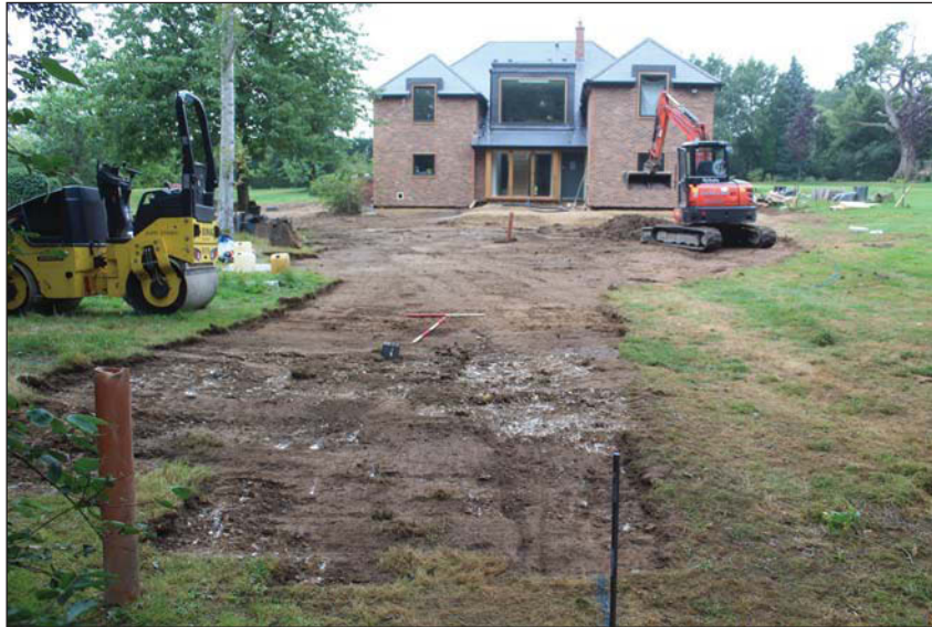
Plate 3. Driveway Strip, looking South, Scales: 2m and 1m.
