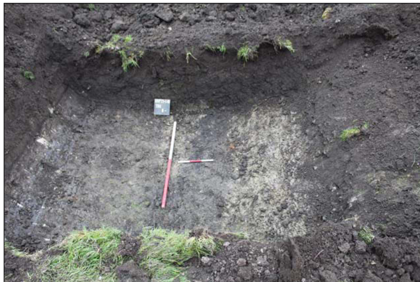
Plate 3. Trench 5, looking North East, Scales: 1m and 0.3m.
