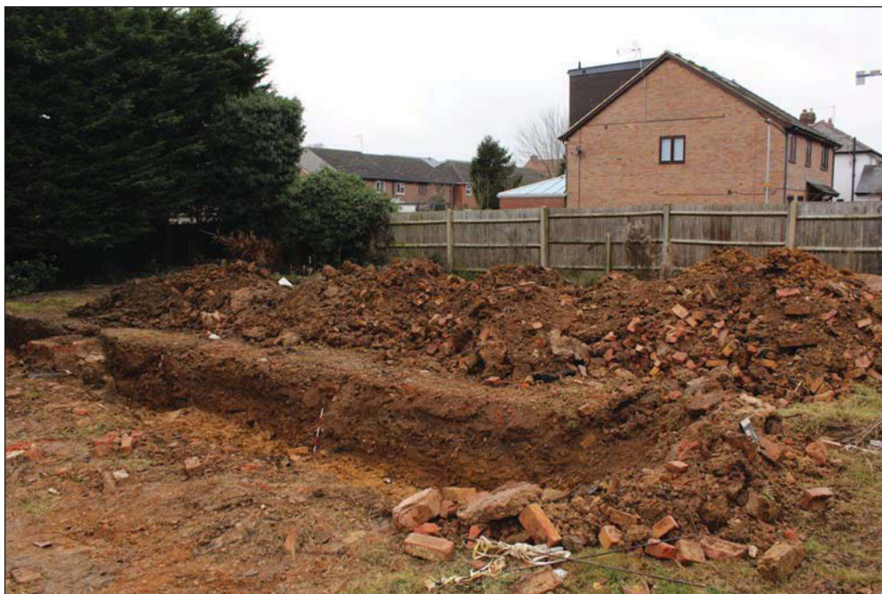
Plate 4. General view looking South west (and Trench 2).
