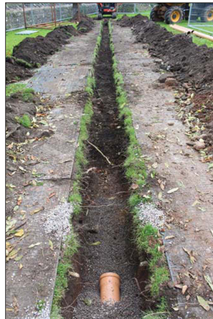
Plate 8. Working shot of south east end of trench, looking south east.
