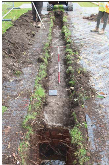
Plate 7. Concrete surface 61, looking south east, Scales: 2m and 0.5m.
