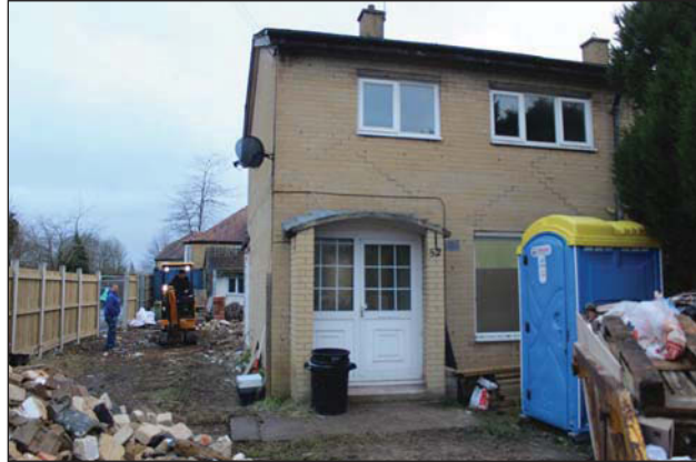
Plate 1. Front elevation of house, working area on left.
