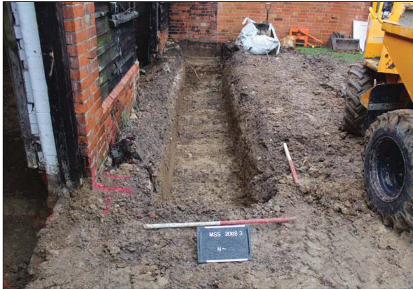
Plate 9. Exterior ground reduction, looking East, Scales: 1m x2.
